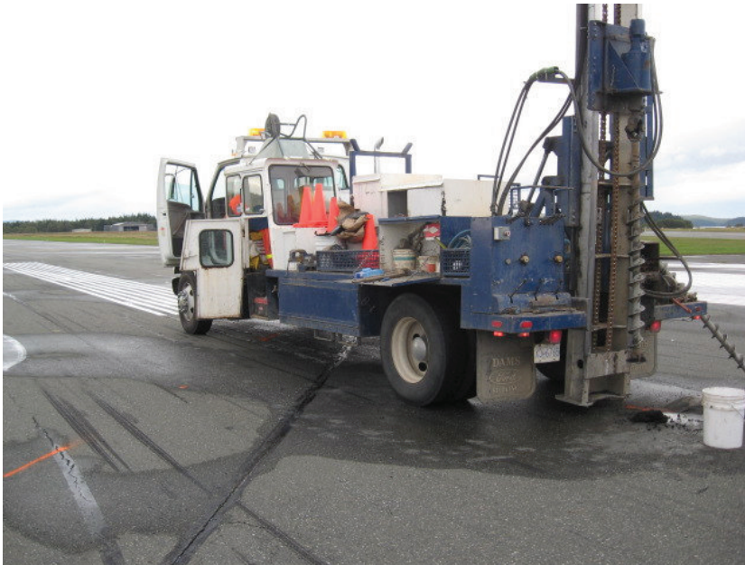
Photo 4: Drill rig set up at AH10-05.
