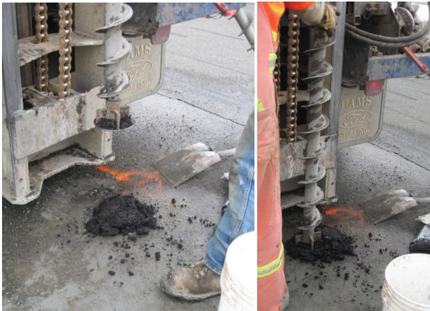
Photo 5: Placing and compacting asphalt patch at AH10-05.
