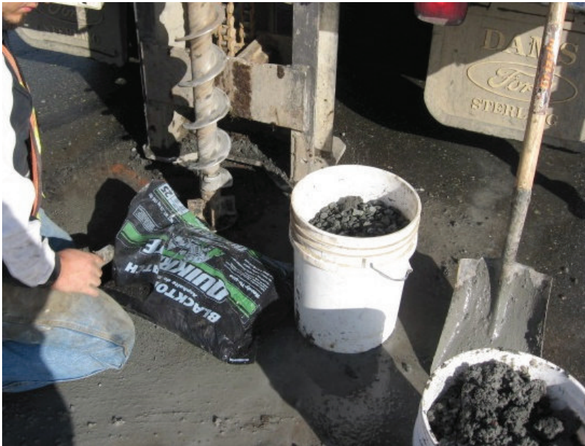
Photo 8: Preparing asphalt patch at AH10-06.
