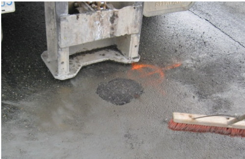
Photo 6: Asphalt patch complete at AH10-05.
