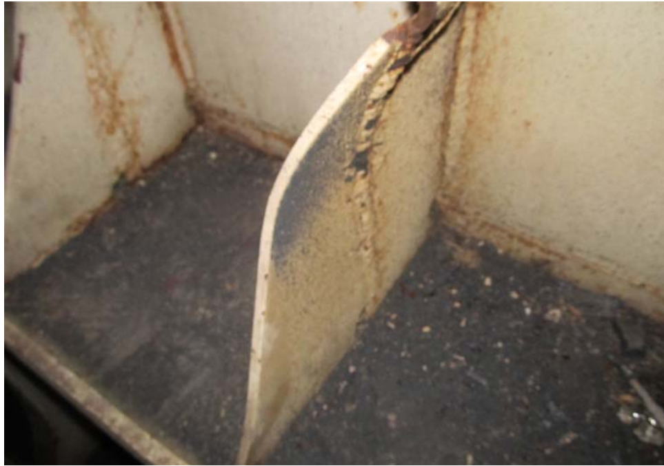
Typical tripped bracket
