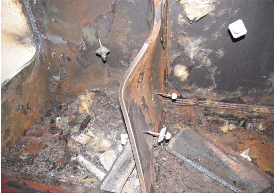
Typical tripped bracket
