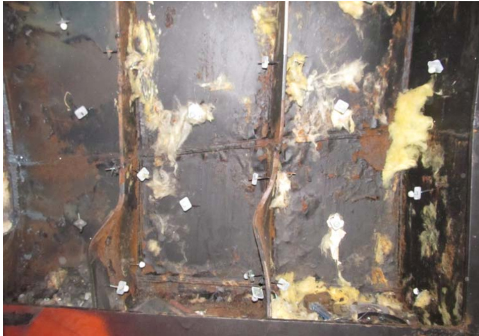
Damaged frames, brackets
