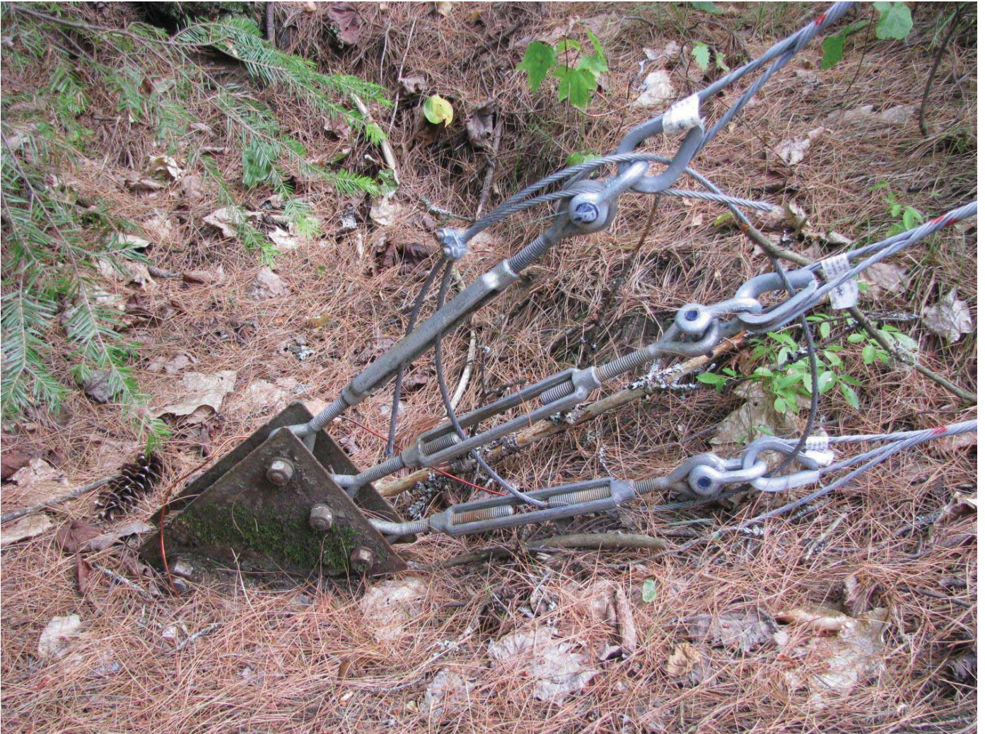
Figure 3.13: Sample Existing Guy Wire Support- Angle 1:
