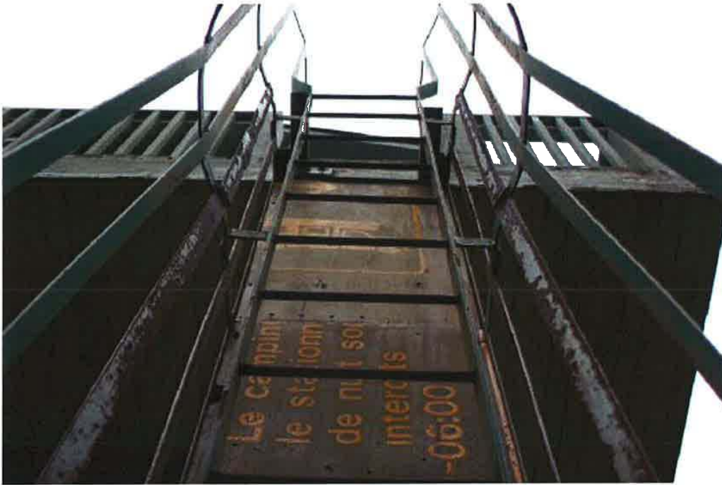
Photo 14: Rusting of cage bars and rungs requiring repairs
