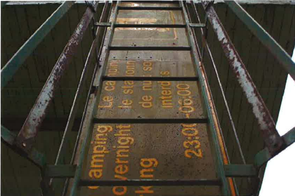
Photo 15: Rusting of cage bars and rungs requiring repairs
