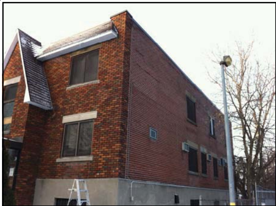
Photo N° 1: View of South (front) and East walls of Ogilvy CCC, for which bricks mortars are different
