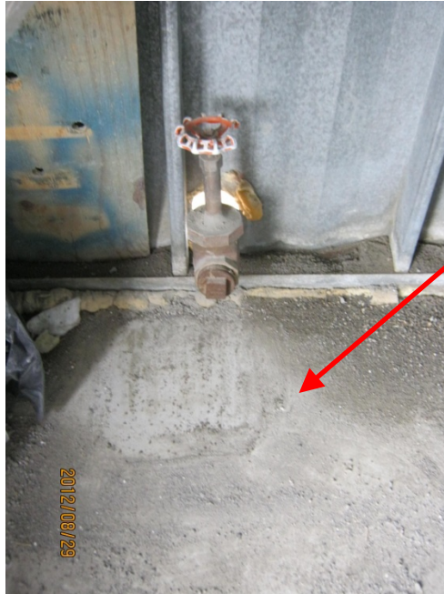
Photo 3 Date: Aug 29, 2012 Location: FTB, Interior Description: Lead containing dust on the concrete floor as indicated by red arrow
