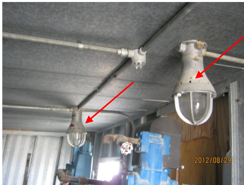
Photo 4 Date: Aug 29, 2012 Location: FTB, Interior Description: Suspected mercury lamps as indicated by red arrows
