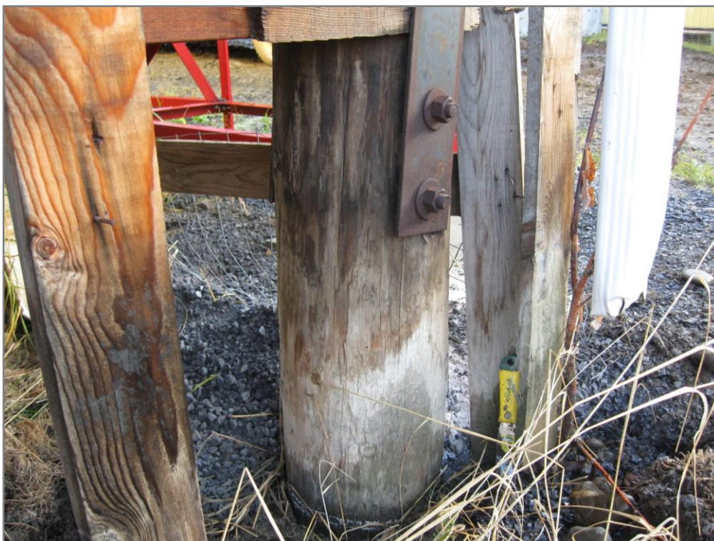
Photograph 6. Southeast pile and cribbing where wood shaving sample obtained. ↑
