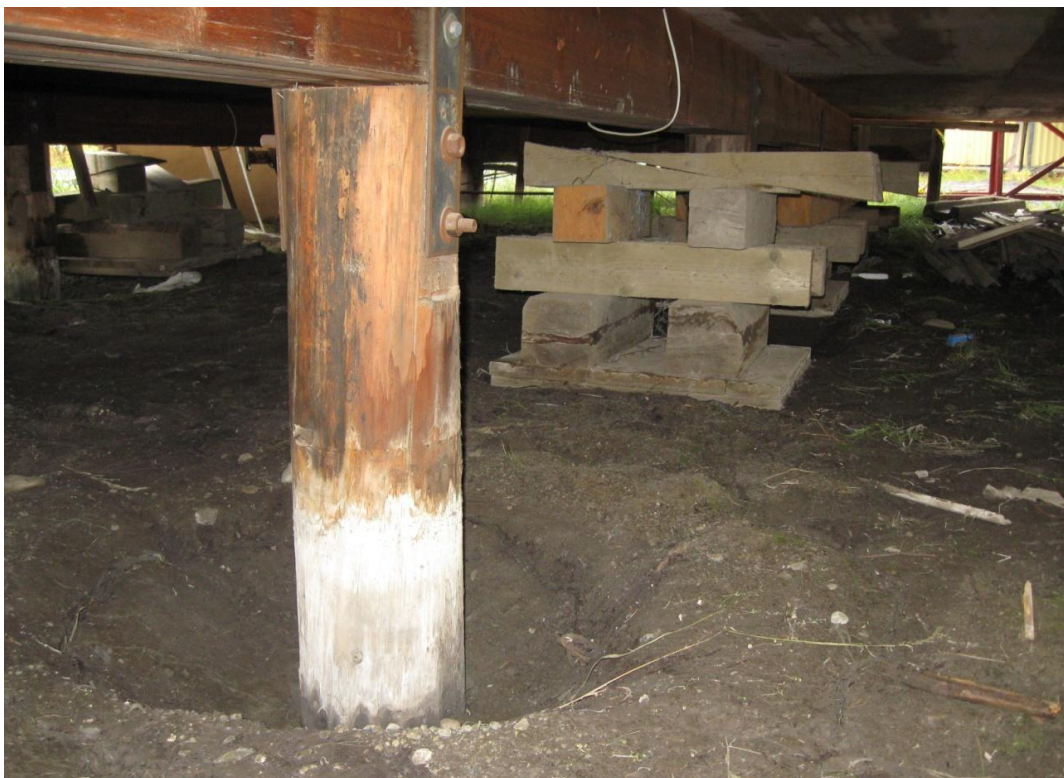
Photograph 5. House piles with erosion wells and cracked soil. ↑
