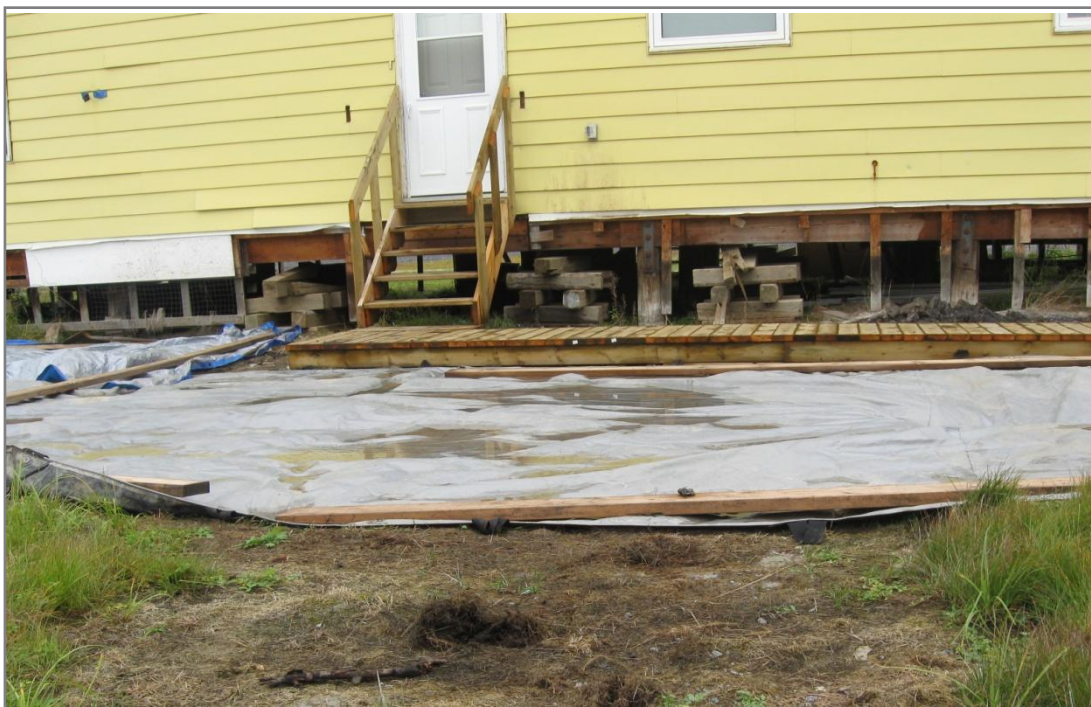
Photograph 1. Facing north over south end of house. Tarps held down by boards over the contamination zone. ↑
