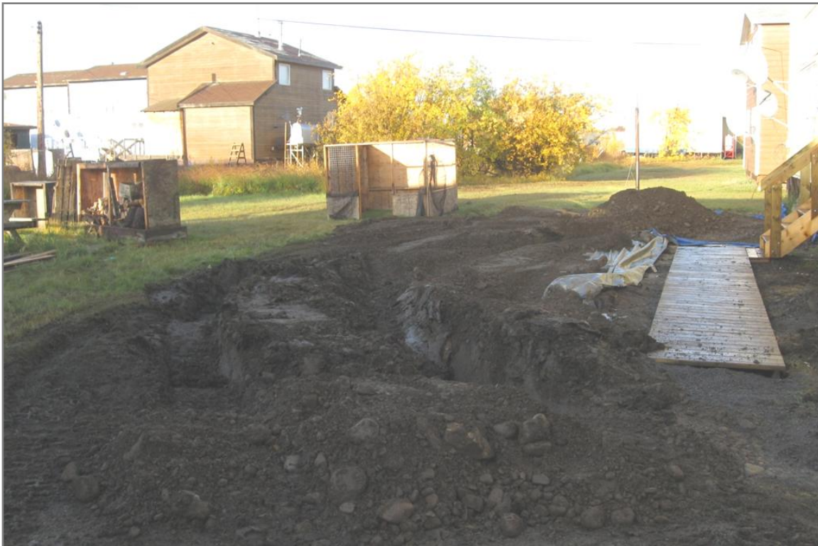
Photograph 13. Ruts remaining from initial attempts to place cover material. Silty soil conditions resulted in heavy equipment getting stuck. ↑
