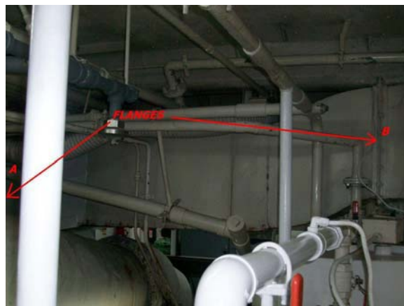
Section of Air Trunk (Flange A & B)
