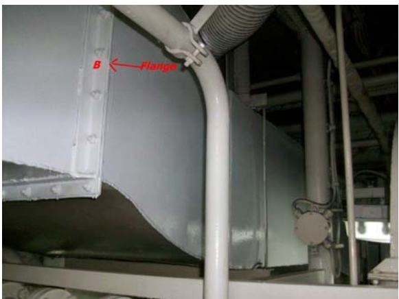
Section of Air Trunk (Flange B)
