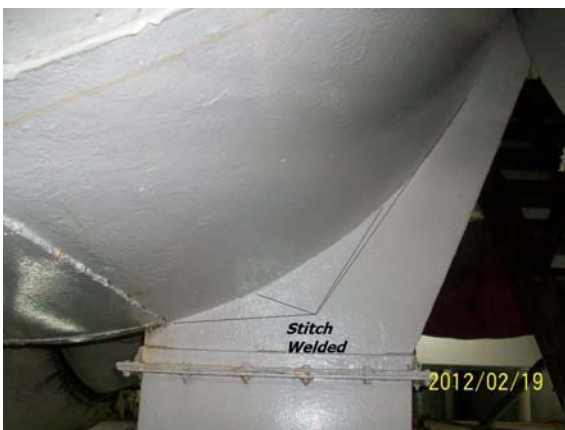
Section of Air Trunk (Flange B)
