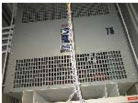
Typical secondary transformer
