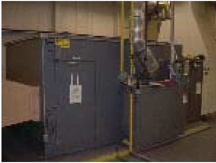
The Engineered Air DJ-100 make-up air unit, located in the east penthouse mechanical room
