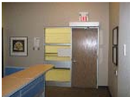
An oak laminated door with a solid softwood core
