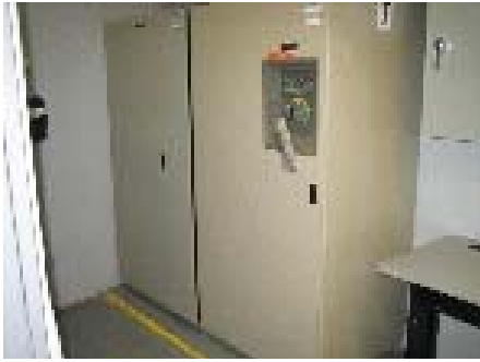
UPS System for emergency lighting
