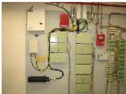
Main telephone termination backboard
