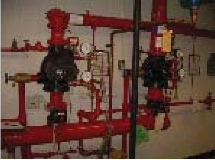
Sprinkler tree located in a basement mechanical room
