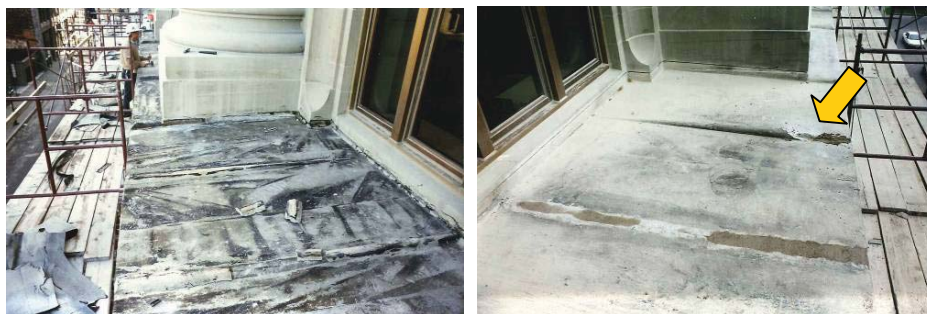
Figures 76 and 77 Removal of the stone “strips” on the deep cornice at the base of the columns, patching the surfaces damaged in the process, here along Normand Street.
