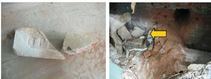
Figures 37 and 38 Brick fragments from the boring drilled on the 5 th floor in the southeast corner of 105 McGill, metal tie between the solid wall and the interior facing in the same location.
