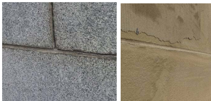
Figures 11 and 12 Existing granite and sandstone claddings.
