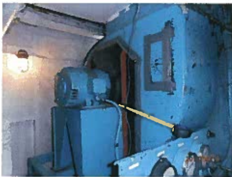
Port HVAC Fan/Motor Assembly 42" Diameter Fan Wheel Housing
