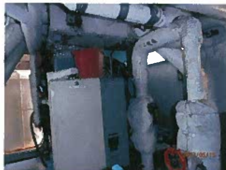
Interferences to Stbd HVAC Fan/Motor access
