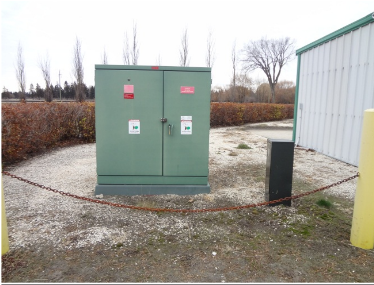
Photo – 7 Transformer TR#1 – 750Kva 12470-347/600V
