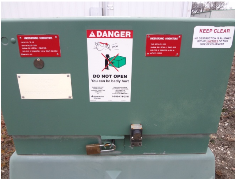
Photo – 8 Transformer TR#2 – 300Kva 12470-347/600V
