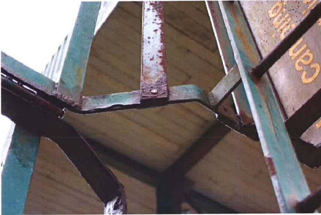
Photo 16: Close up of the rusted cage components
