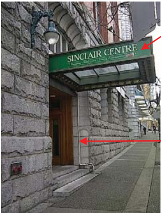
P3. DEMOLISH EXISTING CANOPY DEMOLISH EXISTING RWL, CAP PIPES FOR REUSE
