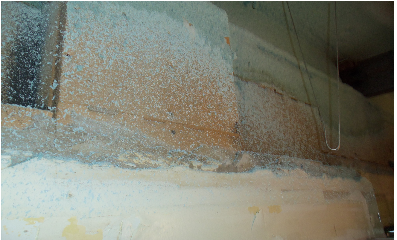
Photo 1 – View in Ceiling Space – Fibreboard, Plaster and New Sprayed Fireproofing.
