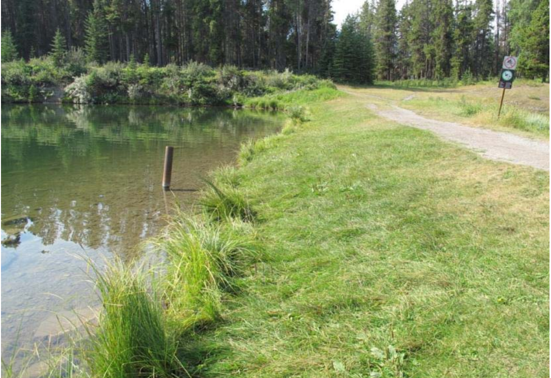
Photo 6 West Dam - Upstream bank looking south
