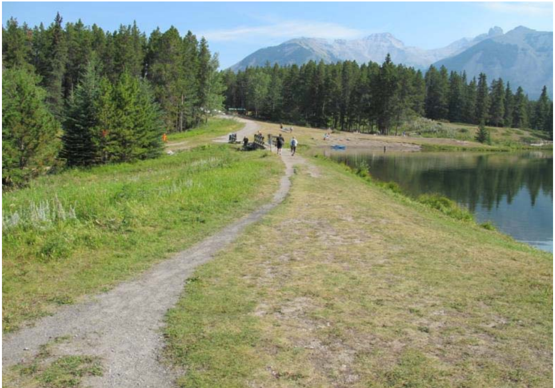
Photo 7 West Dam - Looking north
