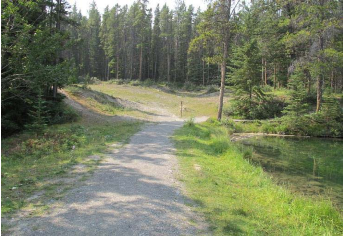
Photo 18 East Dam - Looking towards west abutment
