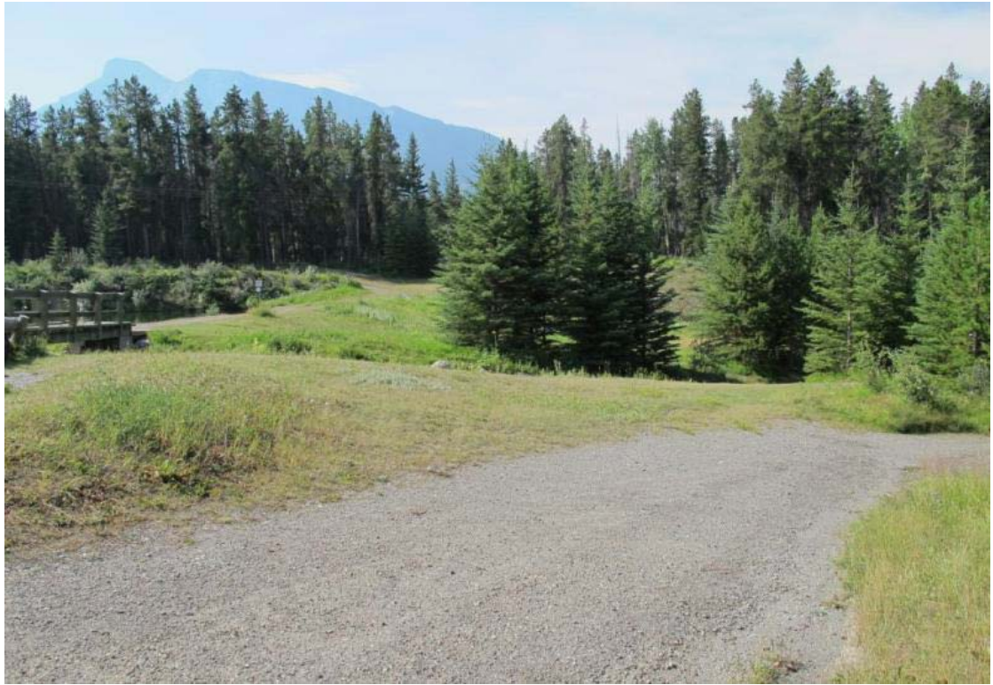
Photo 17 West Dam - Looking south along toe of bank
