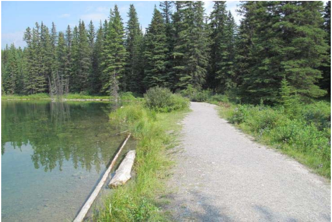
Photo 22 East Dam - Looking towards east abutment
