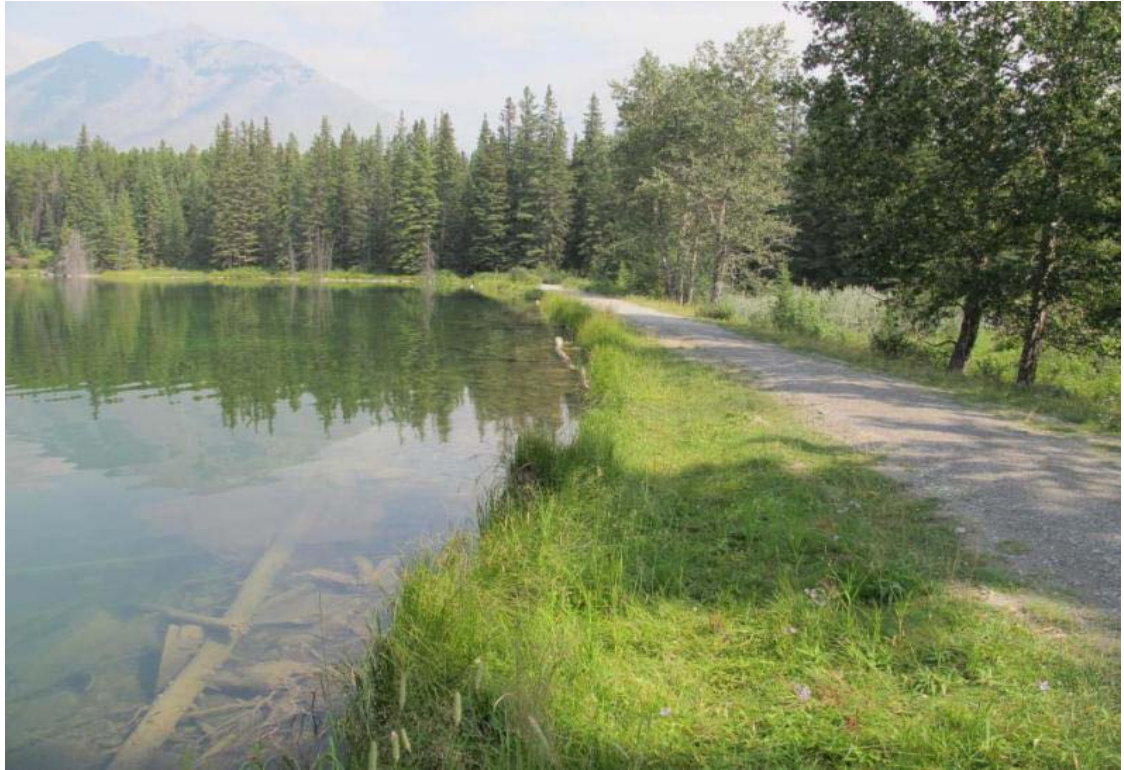
Photo 20 East Dam - Looking towards east abutment
