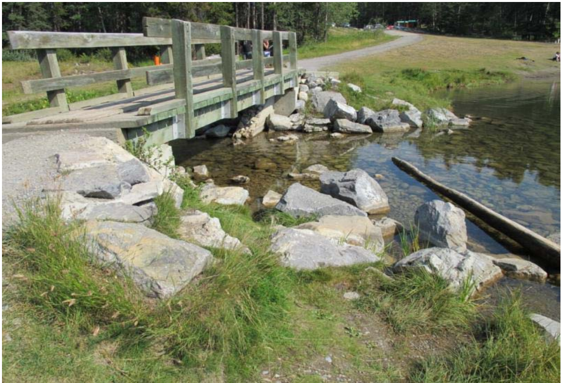
Photo 4 West Dam - South side of spillway
