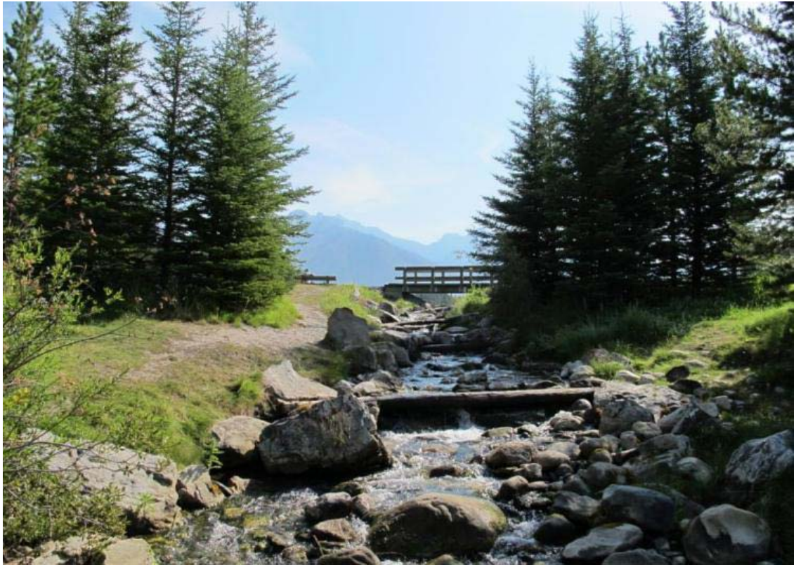
Photo 13 West Dam - Downstream creek looking towards spillway
