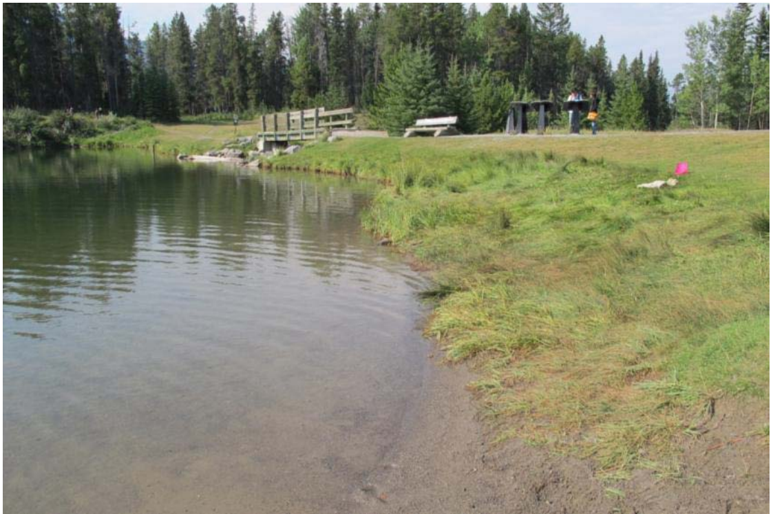
Photo 2 West Dam - looking west from beach
