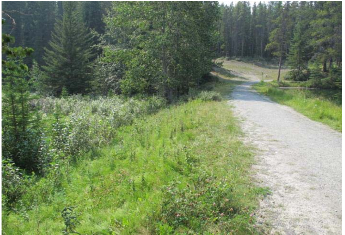
Photo 27 East Dam - West end vegetation on downstream bank
