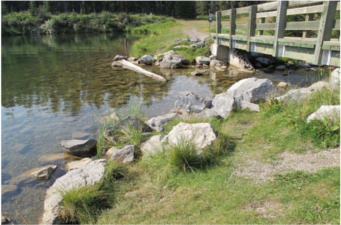
Photo 3 West Dam - North side of spillway
