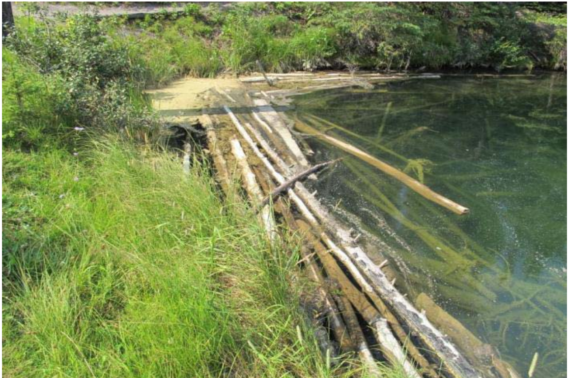
Photo 19 East Dam - Debris accumulating at west end of dam
