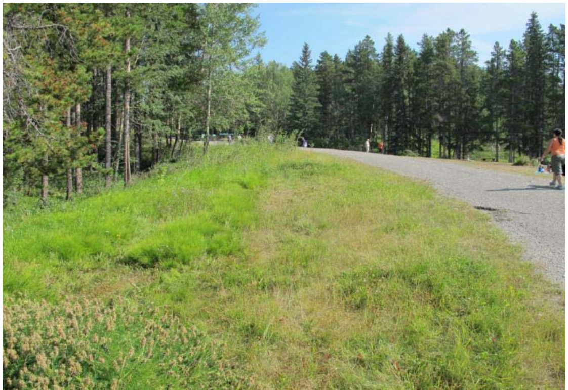
Photo 16 West Dam - Downstream bank looking north
