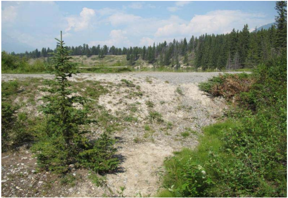
Photo 25 East Dam - Evidence of overtopping
