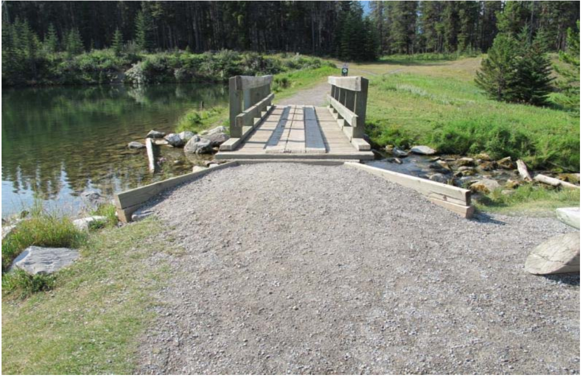
Photo 5 West Dam - Spillway bridge looking south
