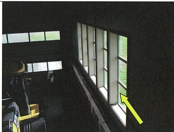
Typical asbestos-containing black window putty applied to the glazing of windows on the North and South facades
