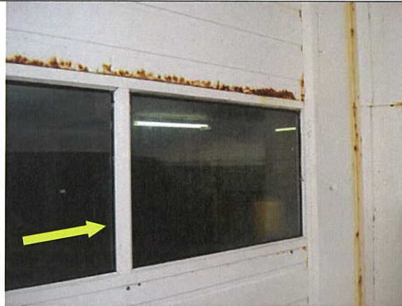
Typical asbestos-containing black window putty applied to glazing of the exterior overhead sectional doors.
