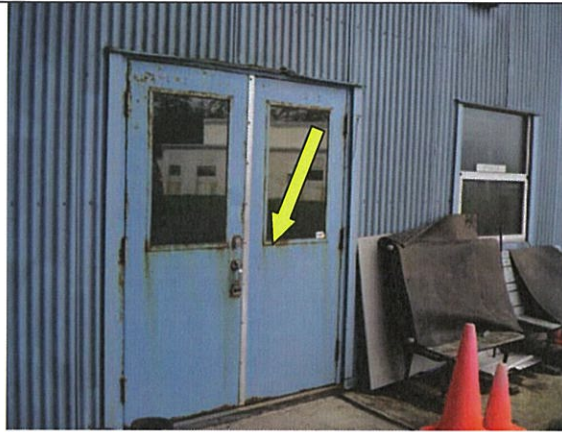
Typical asbestos-containing black window putty applied to glazing of the exterior man doors.
