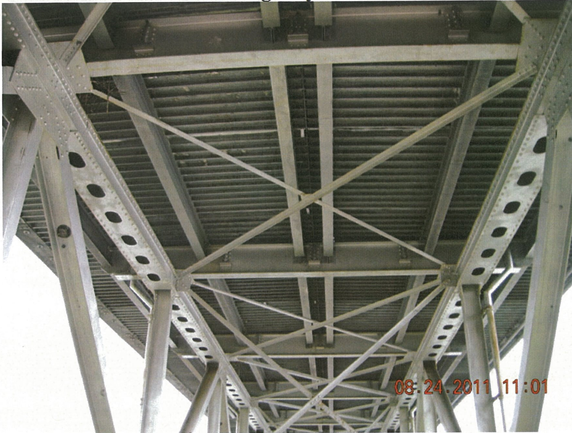
P21 - Span 2 - Floor System - Floorbeams 1, 2 and 3 - Galvanized Stringers
