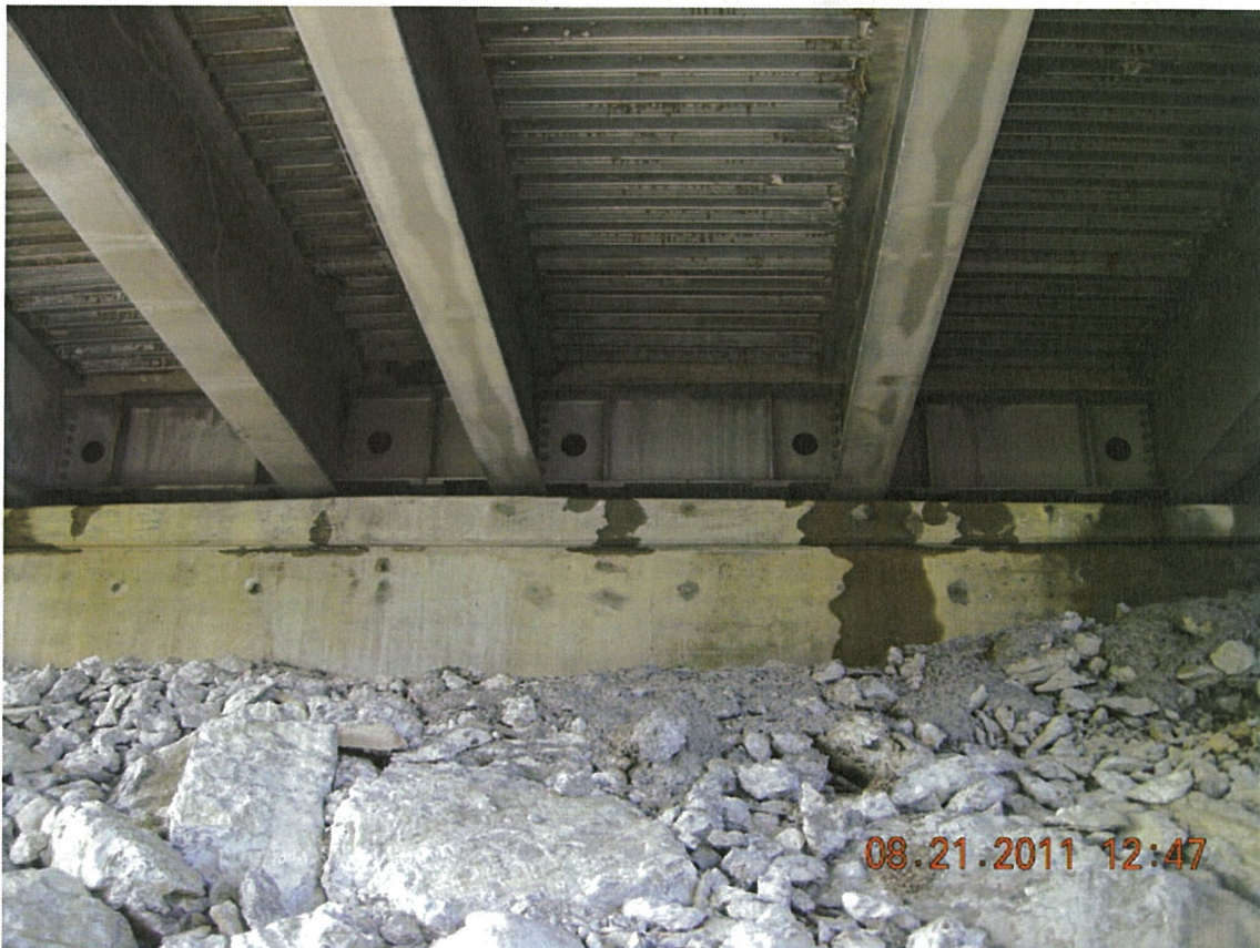
P72 - North Abutment - Moisture Seeping Through North Abutment Deck Joint
