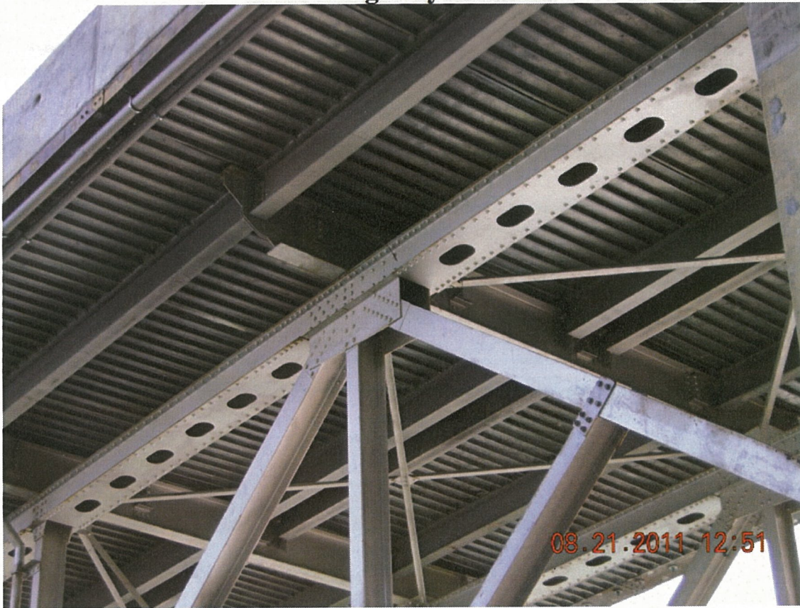
P37 - Span 4 - Orthotropic Steel Deck Panel Soffit
