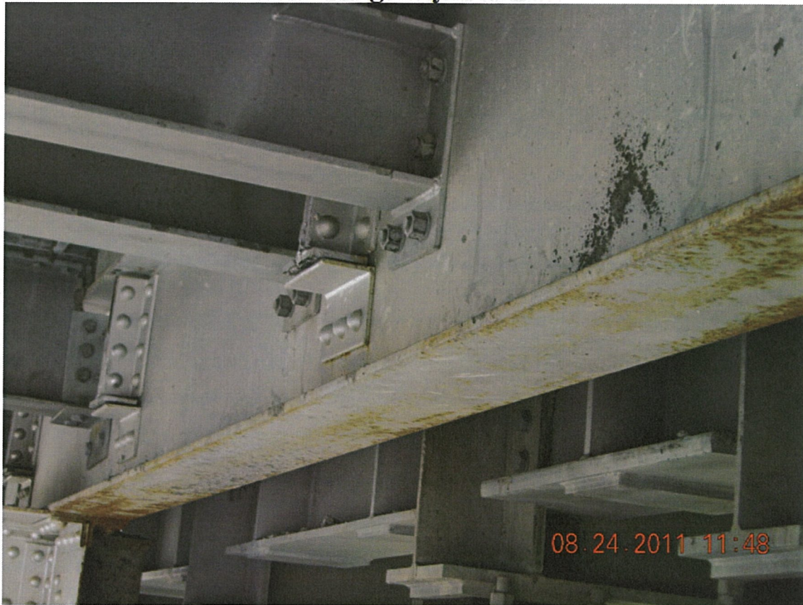
P39 - Span 4 - End Floorbeam below Deck Joint - Light Surface Corrosion on Bottom Flange
