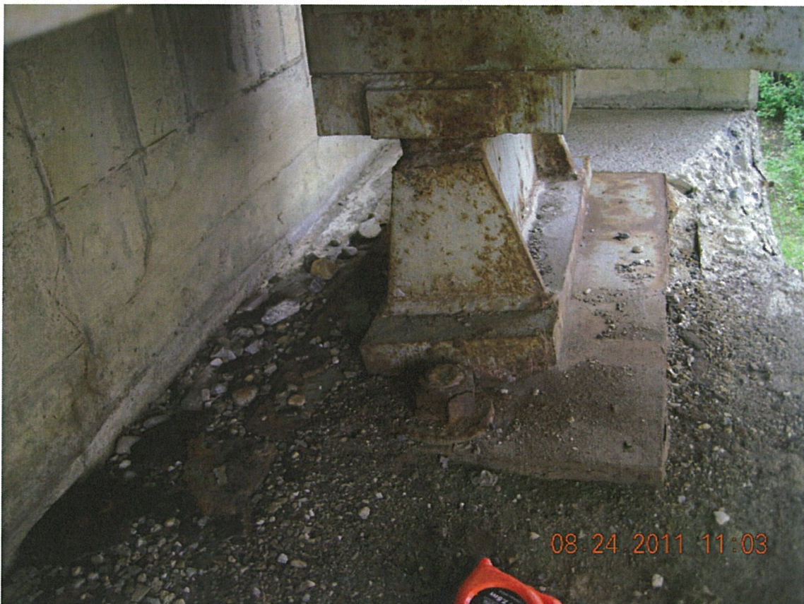
P56 - Pier 1 - Span 2 - West Rocker Bearing - Bearing Seat Dirty - Spalling in Seat Adjacent to Bearing
