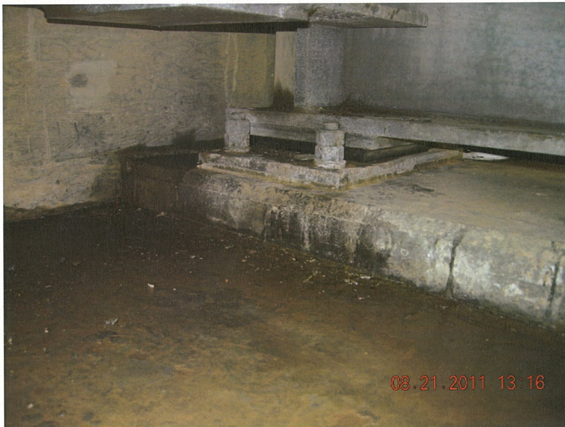
P50 - South Abutment - Neoprene Bearing 5 - Moisture on Bearing Seat
