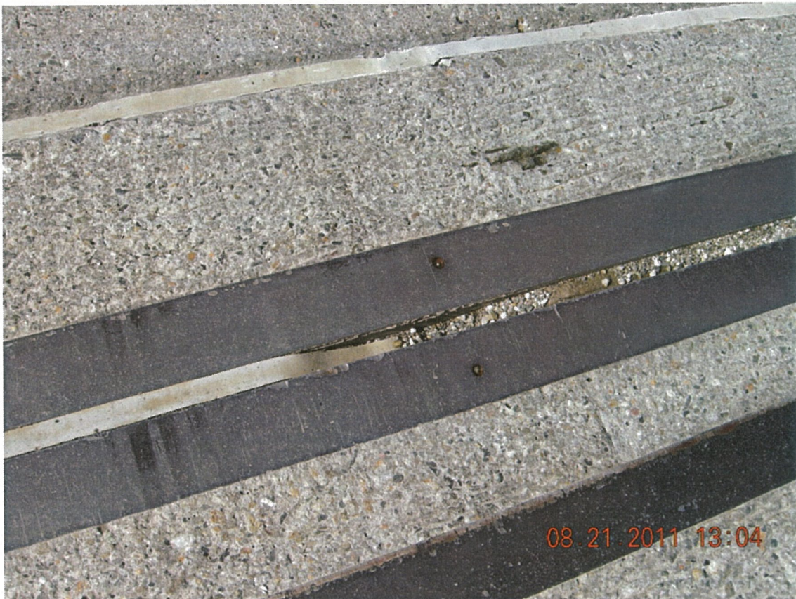
P14 - North Abutment Deck Joint - Joint Seal has Failed
