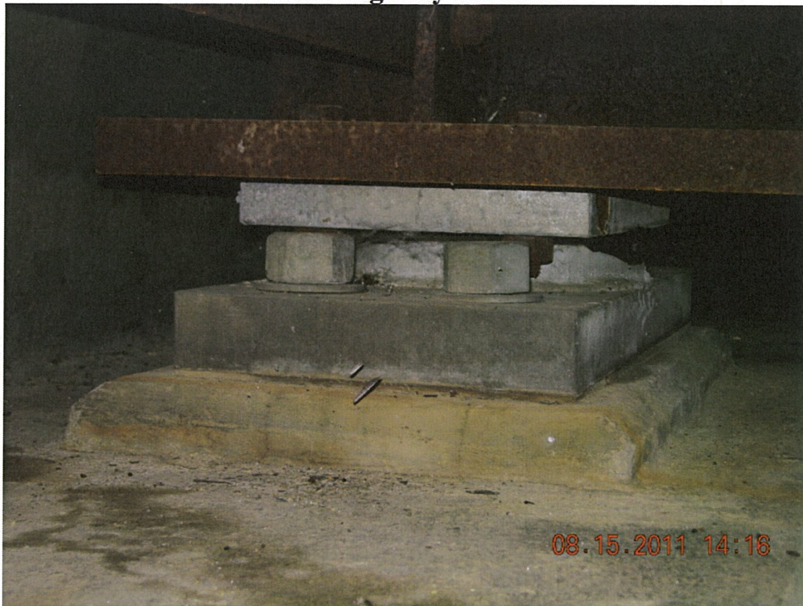
P31 - North Abutment - Fixed Pot Bearing 3 - Neoprene Pads Squeezing Out
