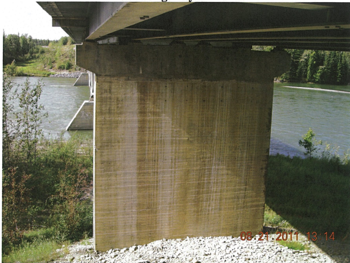
P51 - Pier 1 - South Face - Pier Cap Replaced in 2004
