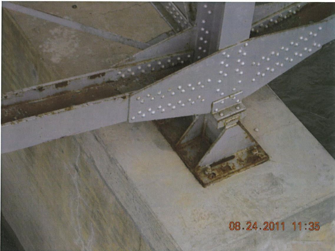
P64 - Pier 3 - East Fixed Bearing - Pier Cap Repaired in 2004
