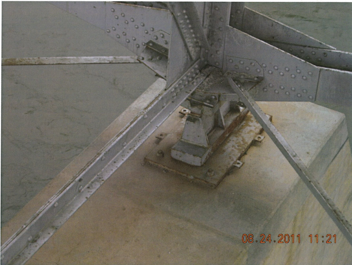
P60 - Pier 2 - West Rocker Bearing - Pier Cap Repaired in 2004
