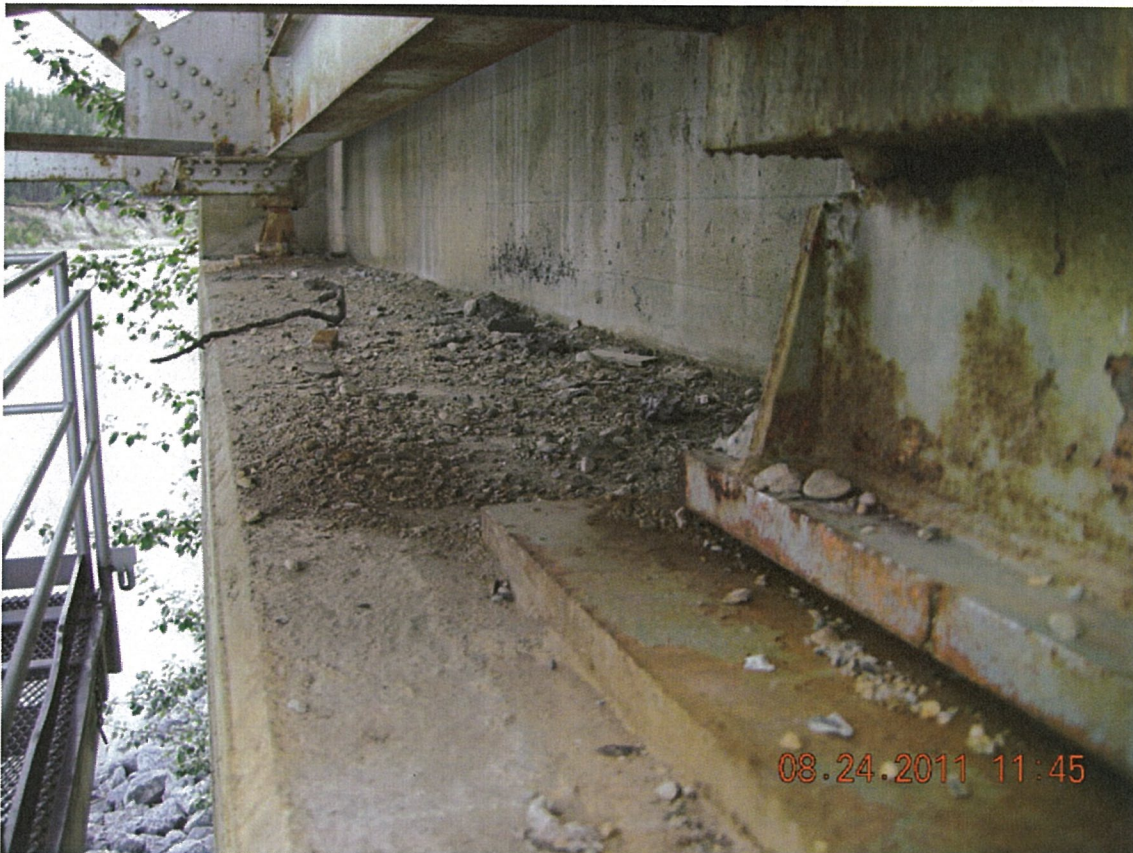
P68 - Pier 4 - Span 4 - Bearing Seat Dirty
