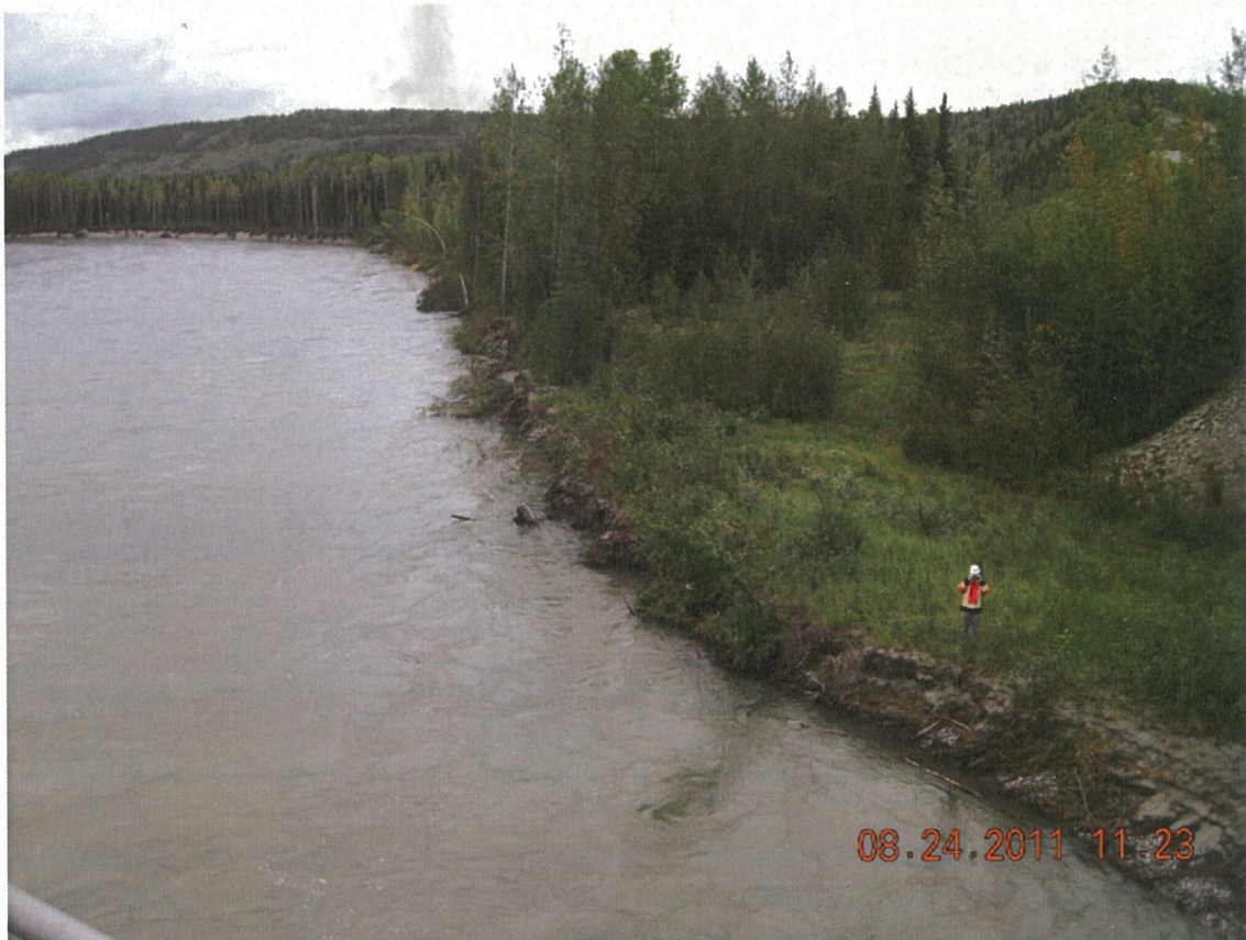
P74 - SE Shoreline - Undergoing Significant Scour - Many Trees Going into Water
