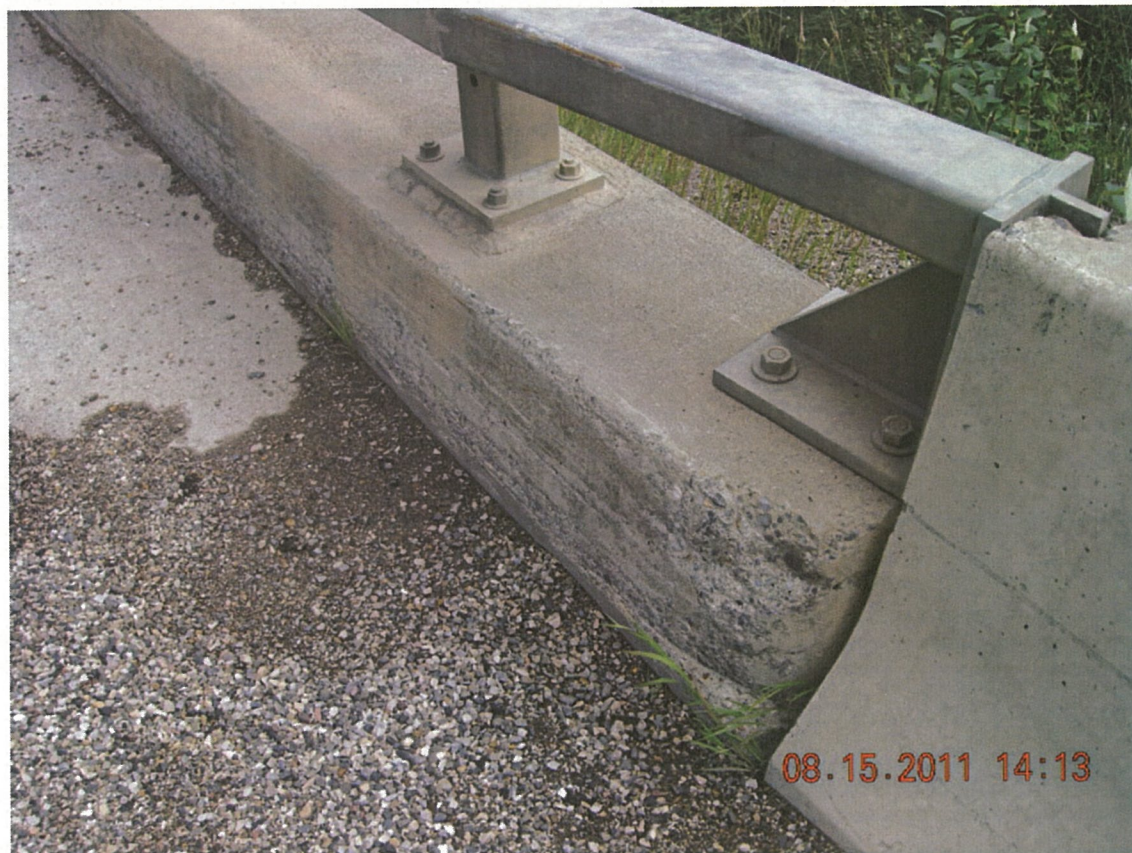
P14 - Curb at NW Corner - Minor Snow Plow Abrasion on Concrete Curb - Narrow Shrinkage Cracks at ~2 m Spacing
