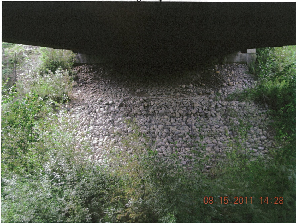
P27 - North Abutment and Embankment - Slope Protected with Gabions
