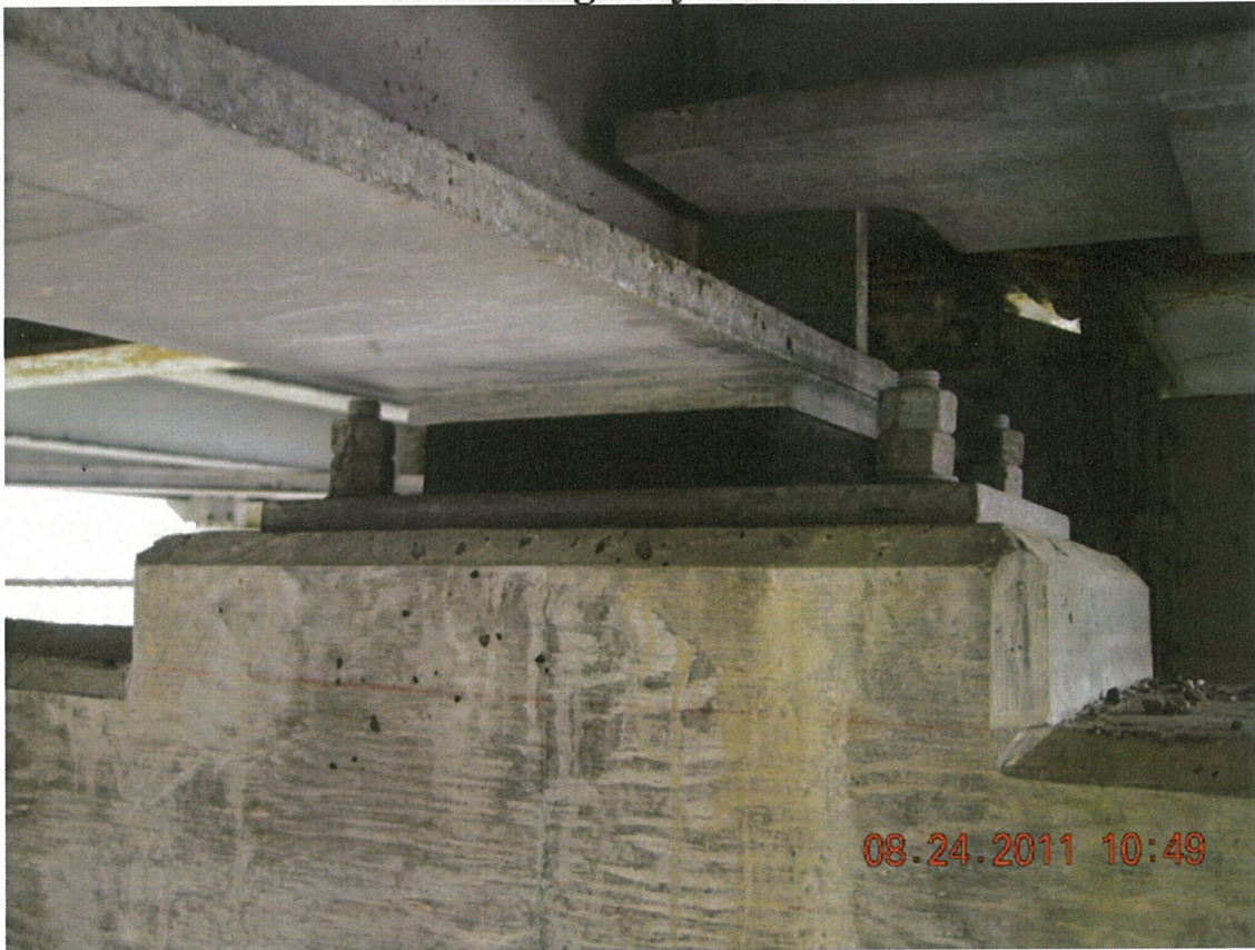
P53 - Pier 1 - Span 1 - Neoprene Bearing 2
