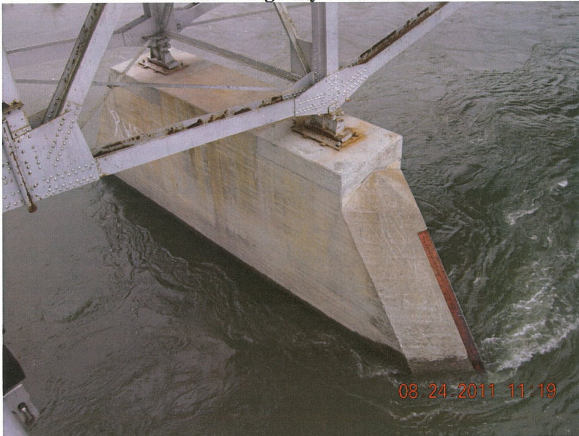
P57 - Pier 2 - East Nosing - Now Completely Surrounded by Water - River has Moved Significantly - In 2007 Pier 2 was Not in Water
