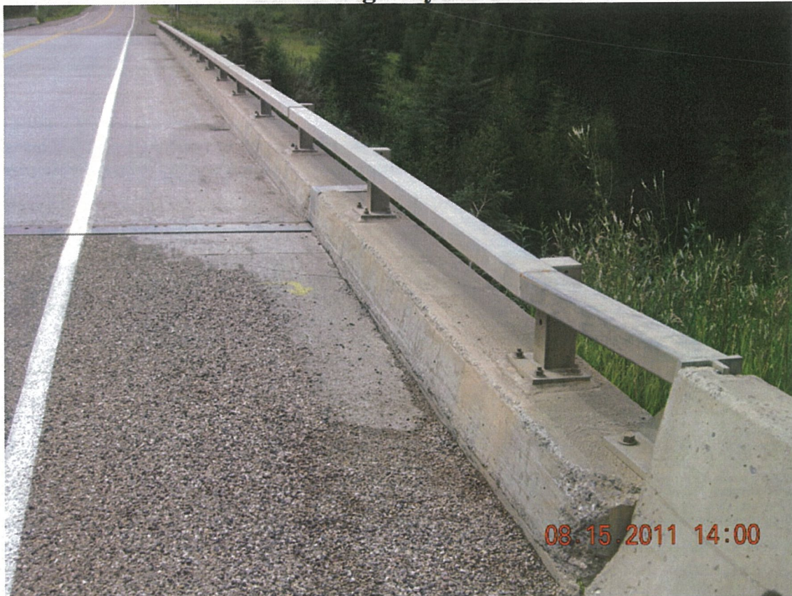
P13 - East HSS Railing Transition to SE Concrete Approach Barrier - Minor Snow Plow Abrasion on Concrete Curb
