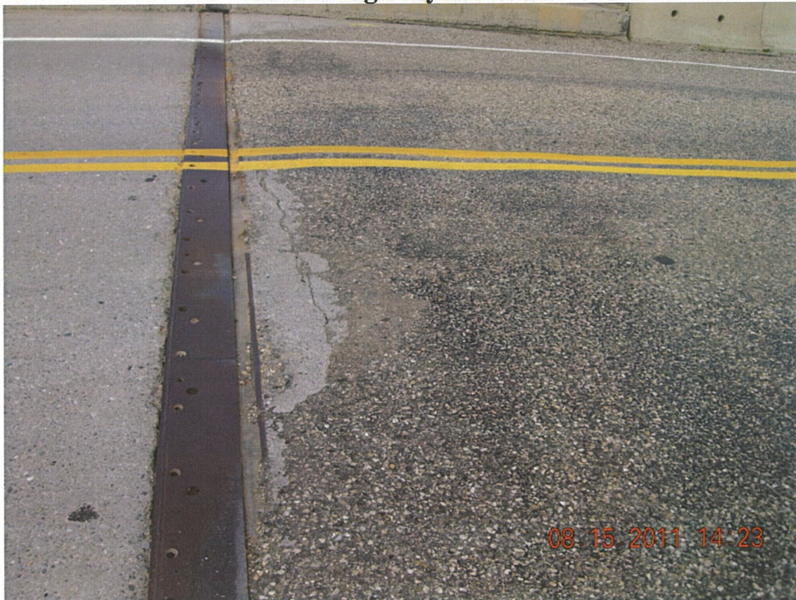
P09 - South Expansion Joint and South Approach Slab - Approach Slab Covered in BST - Wide Transverse Crack Exposed in Approach Slab
