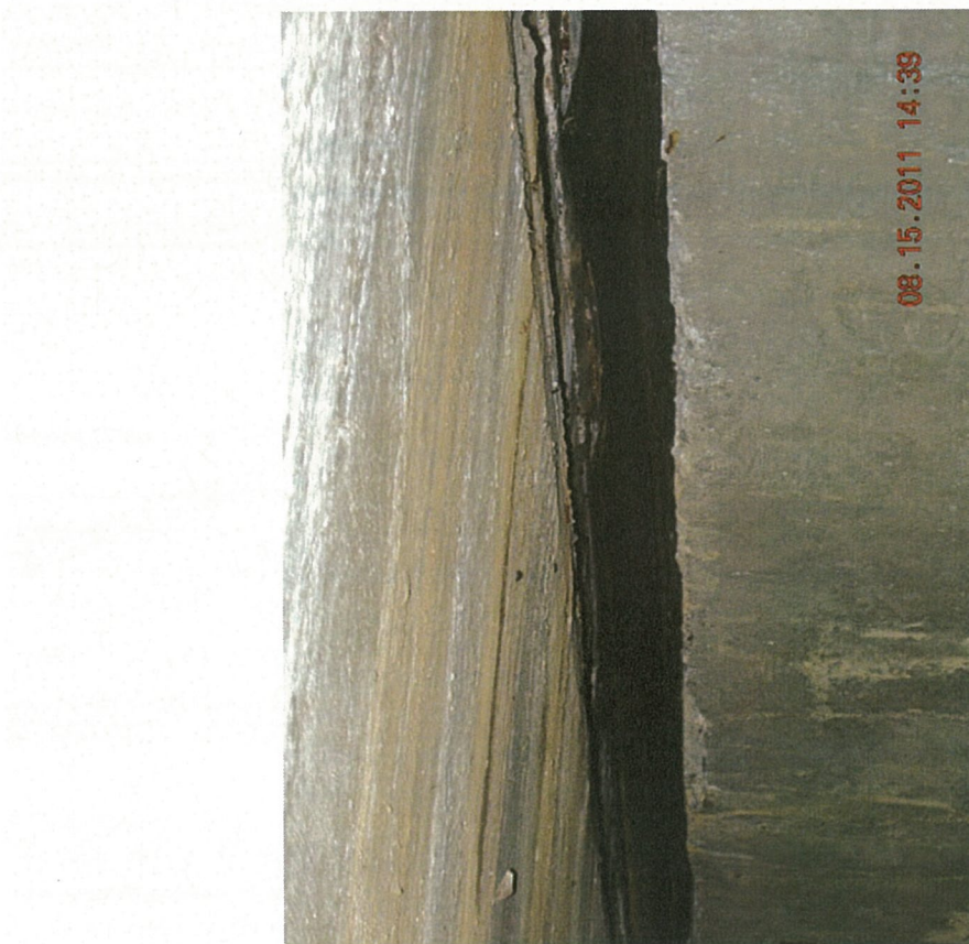
P10 - South Abutment - Bearing Seal - From Below - Torn in Several Locations - Leaking Full Length
