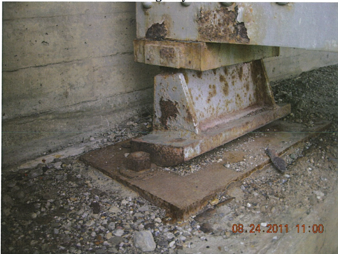
P55 - Pier 1 - Span 2 - East Rocker Bearing
