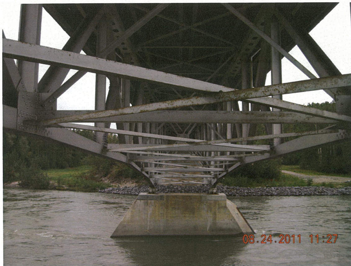
P34 - Span 3 - Deck Truss - Looking North - Bottom Chords and Sway Bracing
