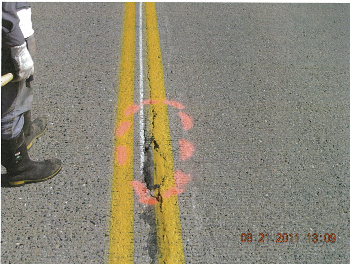
P08 - Span 1 - Longitudinal Crack in Deck at Centreline between Deck Panels - Present Since 2004 Deck Replacement
