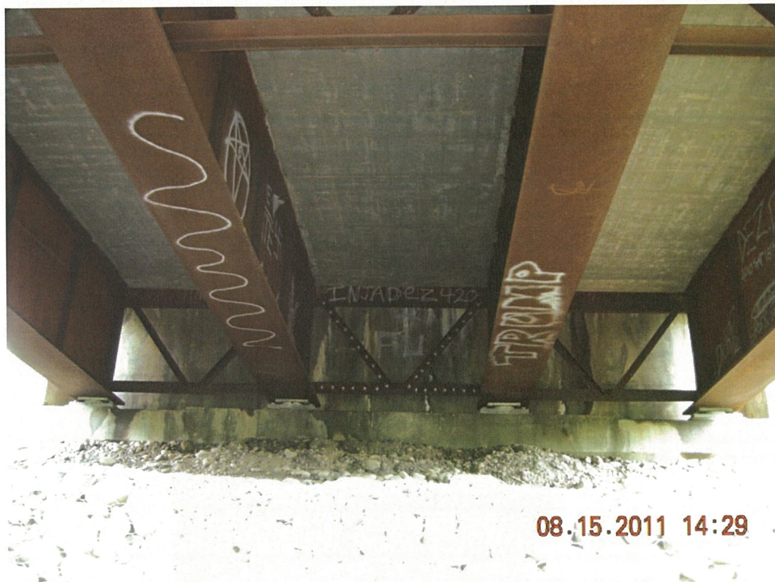
P22 - South Abutment - Moisture Staining from Leaking Deck Expansion Joint
