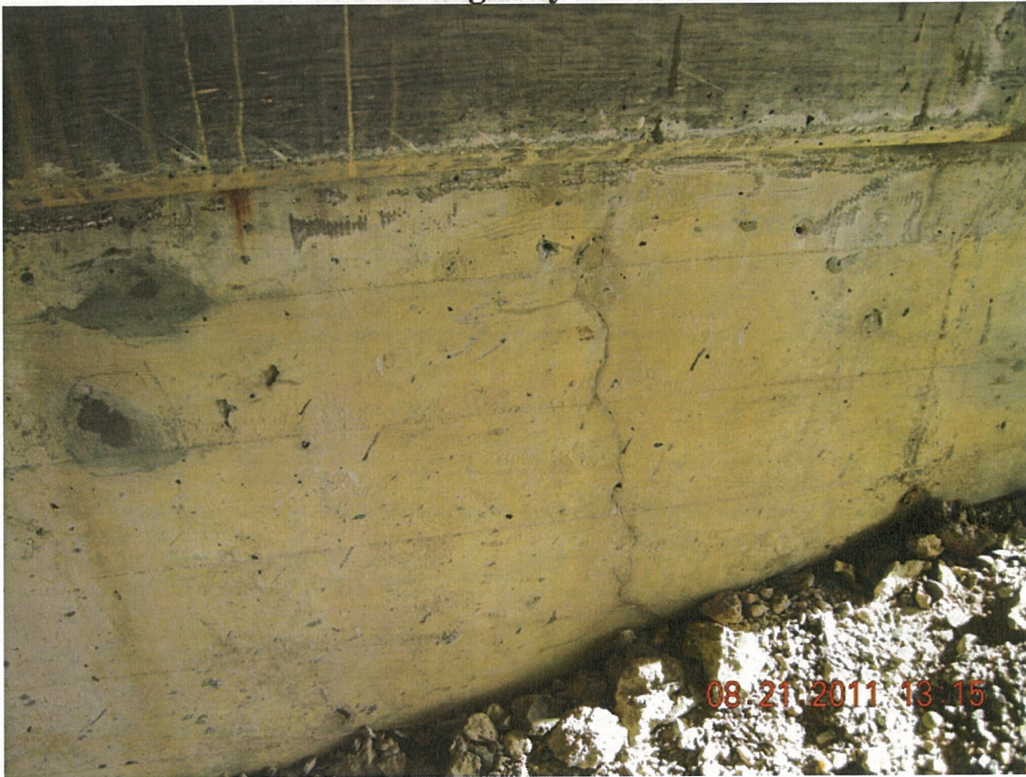
P49 - South Abutment Wall - Hairline Vertical Crack near West End
