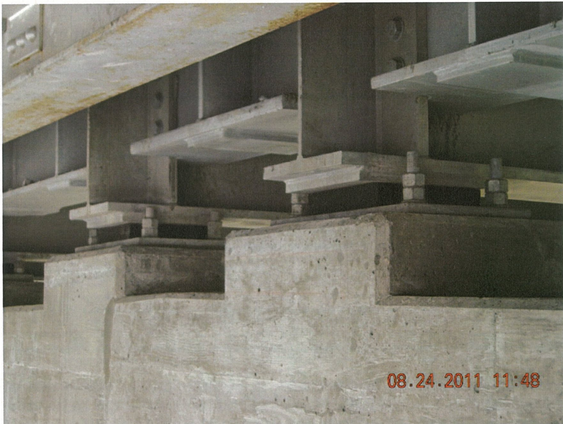
P66 - Pier 4 - Span 4 - Neoprene Bearings
