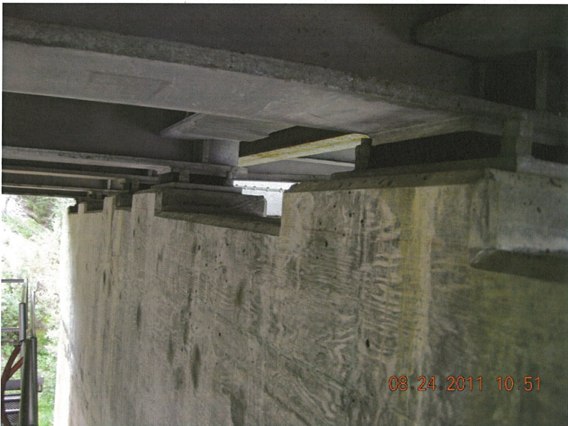
P52 - Pier 1 Bearing Seat - Span 1 Neoprene Bearings
