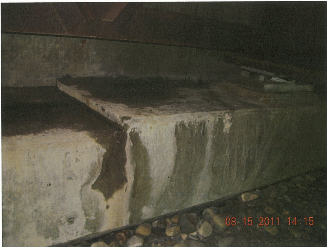
P30 - North Abutment - Bearing Seats Wet
