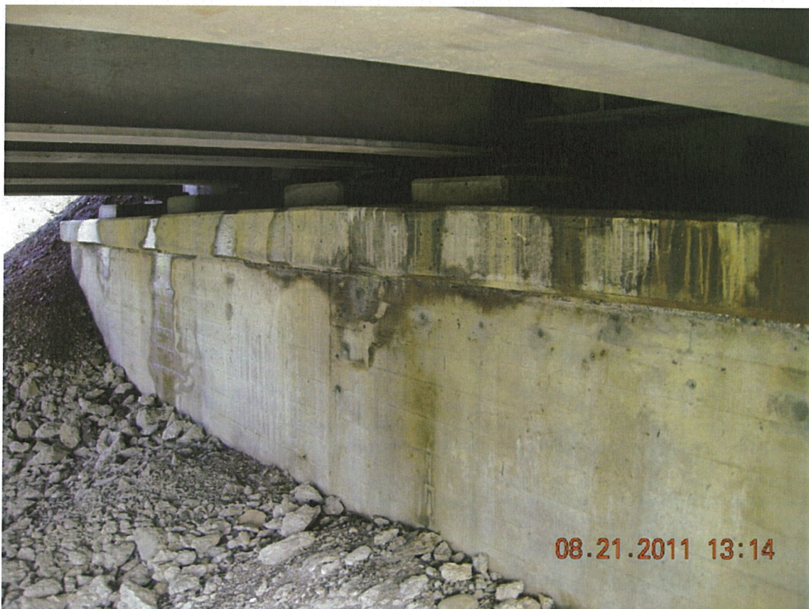
P48 - South Abutment and Bearing Seat - Water Seeping through Deck Joint
