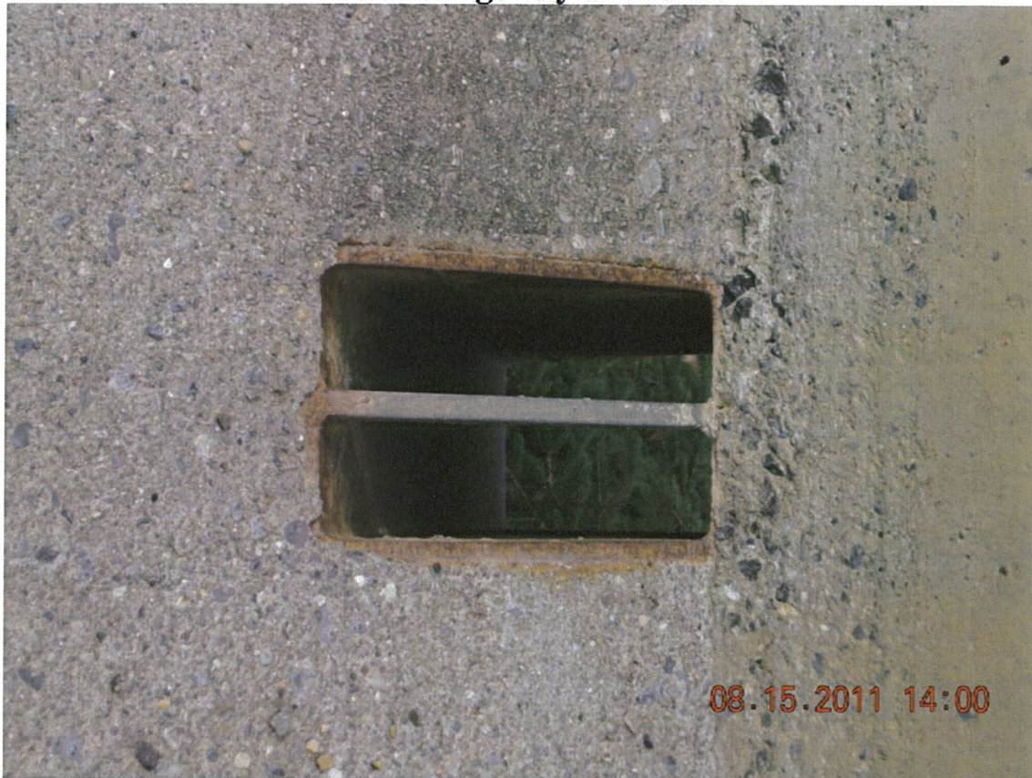
P15 - All 6 Deck Drains Clear and Functioning Properly - Typical
