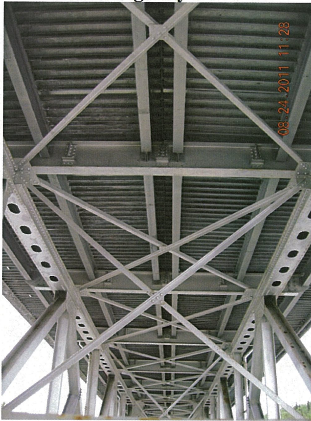
P31 - Span 3 - Orthotropic Deck Soffit - Looking North from Midspan
