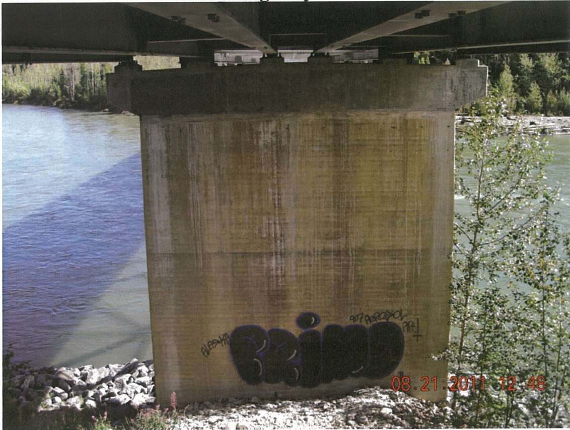
P65 - Pier 4 - North Face - Pier Cap Rebuilt in 2004
