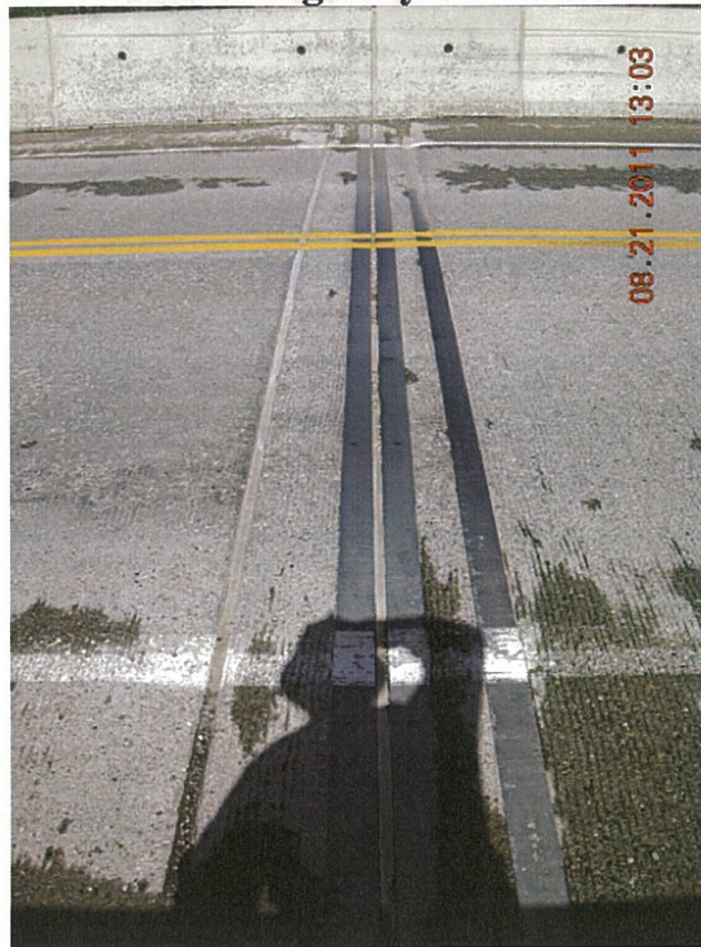
P13 - North Abutment Deck Joint - Joint Seal has Failed
