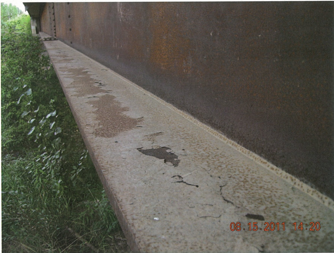
P18 - Exterior Girder 1 - Minor Scaling of Patina on Bottom Flange
