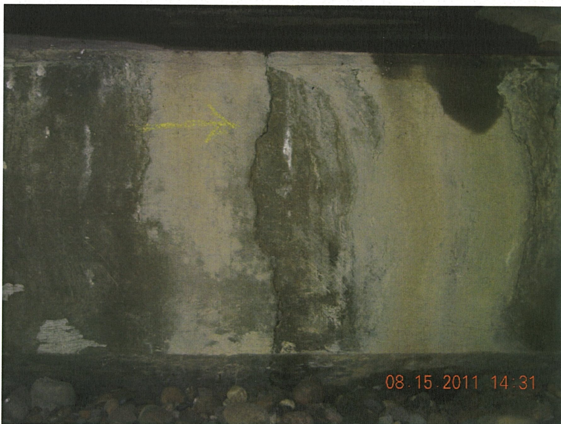
P24 - South Abutment Wall - Narrow Vertical Crack between Girders 1 and 2
