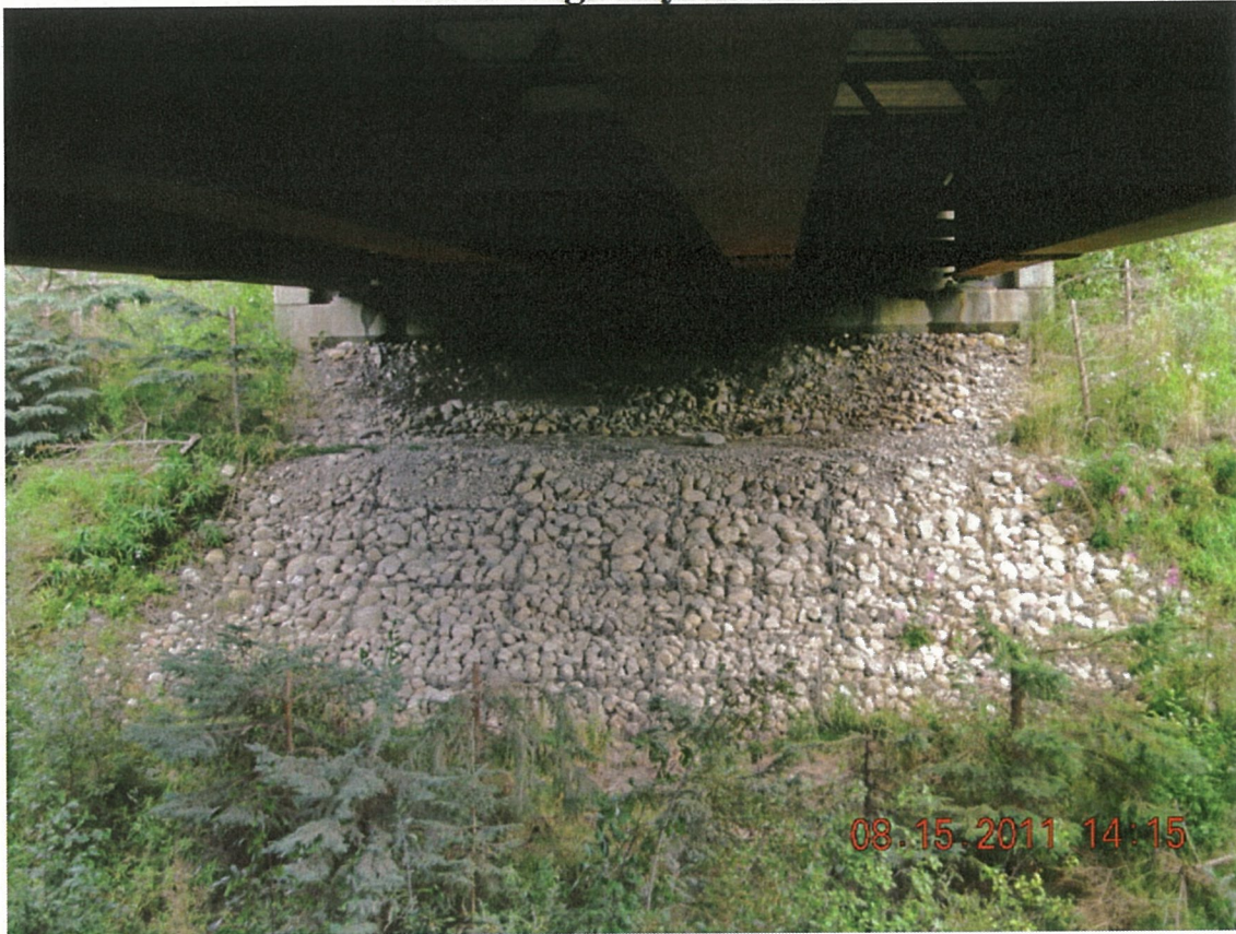
P21 - South Abutment and Embankment - Gabion Slope Protection
