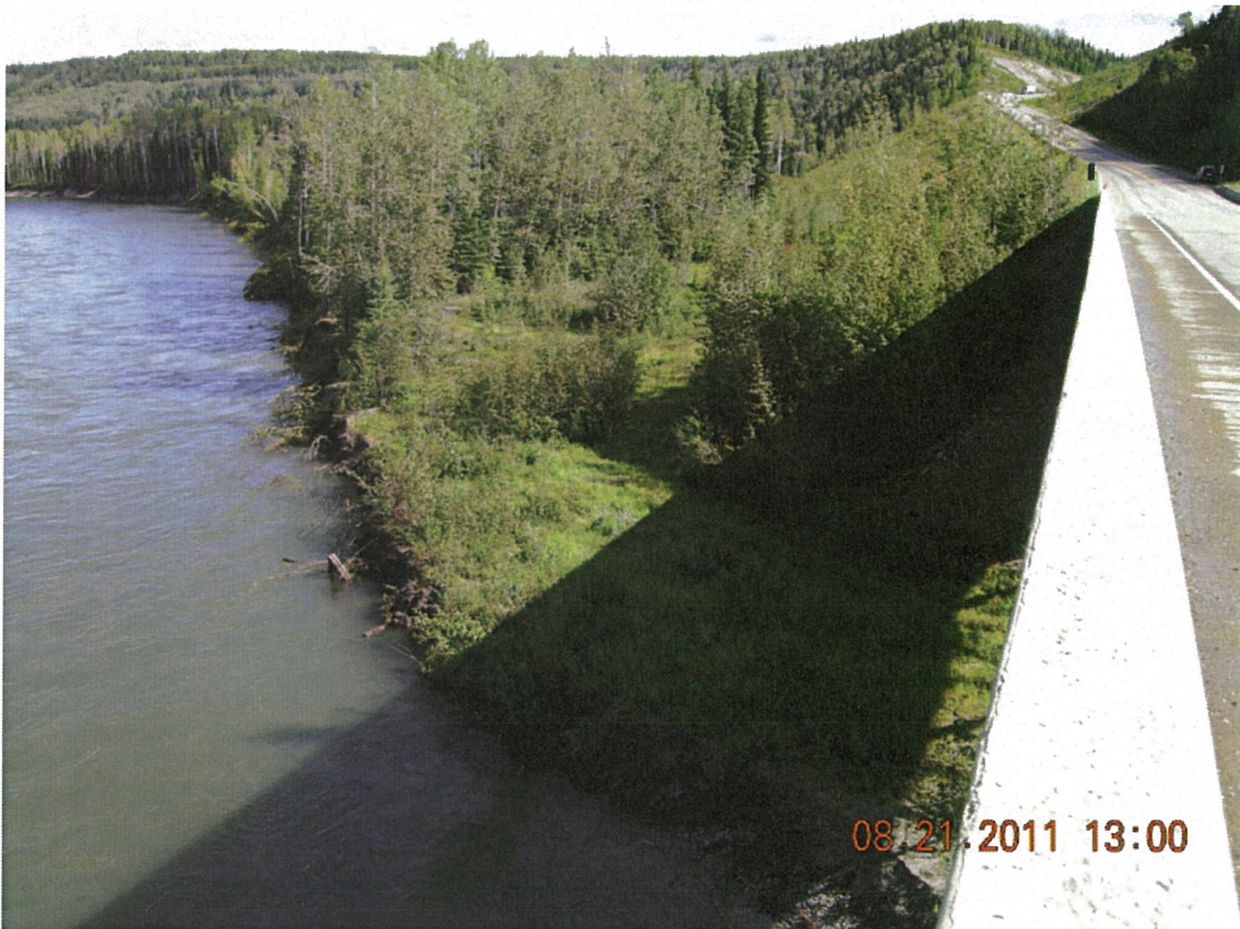
P04 - NE Shoreline - Active Scour - Shoreline has Moved South by ~10 m Since 2009 Inspections - South Approach Embankment will soon be Threatened
