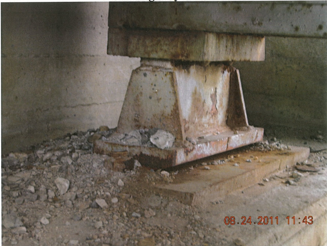
P69 - Pier 4 - Span 4 - East Rocker Bearing - Bearing Seat Dirty
