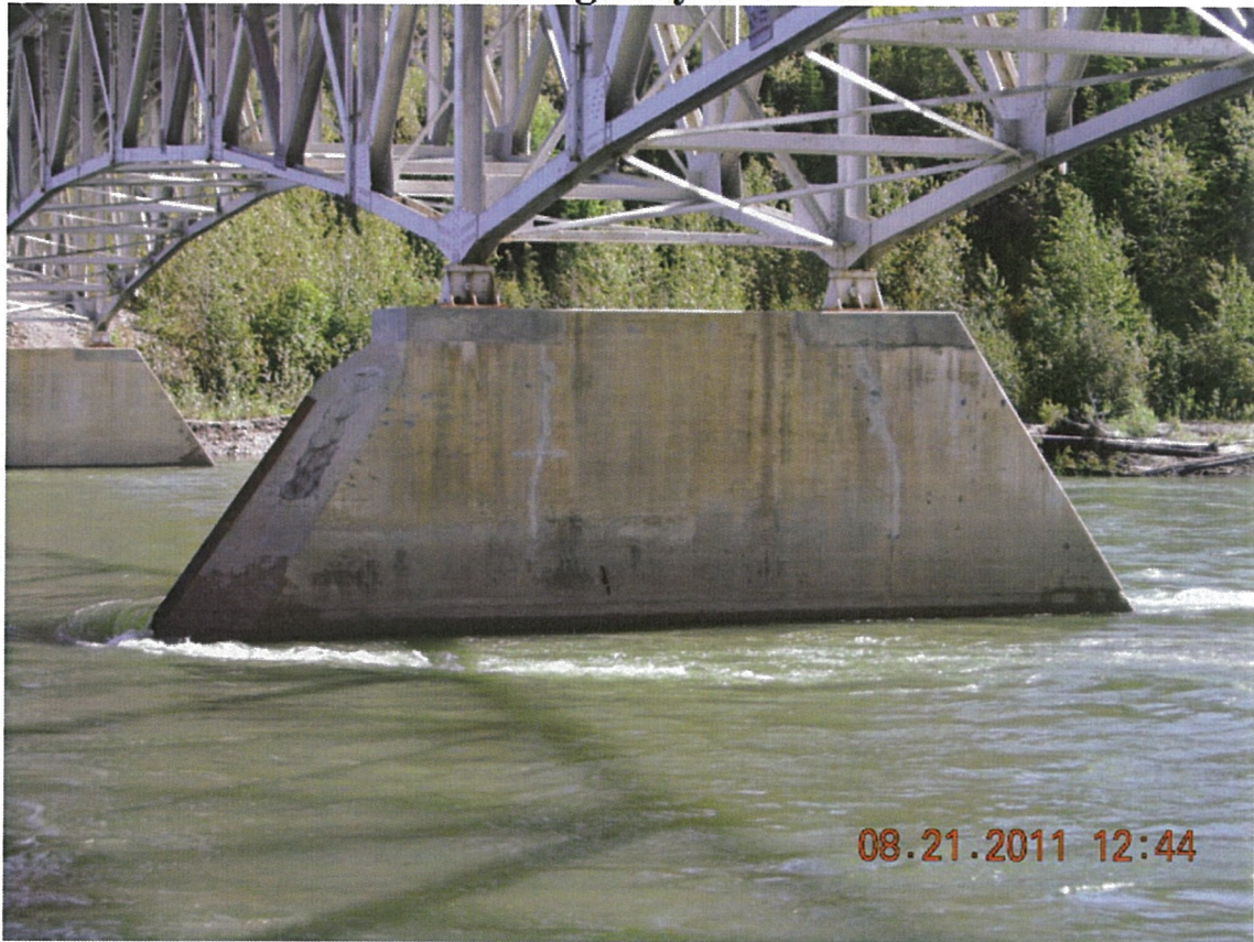
P63 - Pier 3 - North Face - Pier Cap Repaired in 2004
