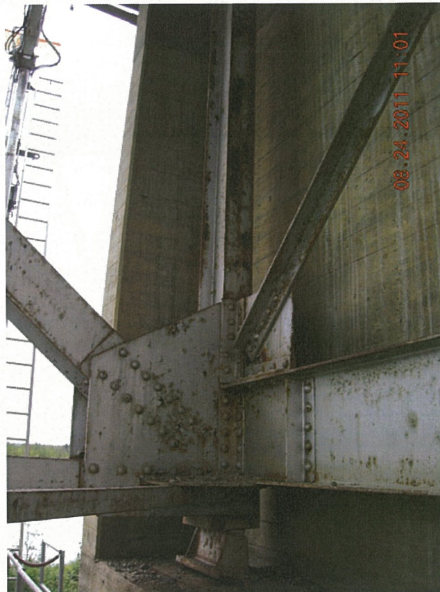
P22 - Span 2 - L0-U0 East - Vertical - Paint System Falling Below Deck Joint - Light Surface Corrosion - Negligible Section Loss
