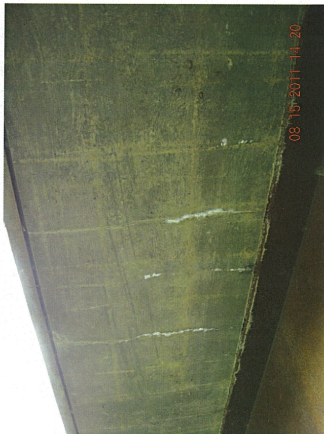
P20 - Cantilever Soffits have Hairline Transverse Shrinkage Cracks with Efflorescence at ~500 mm Spacing
