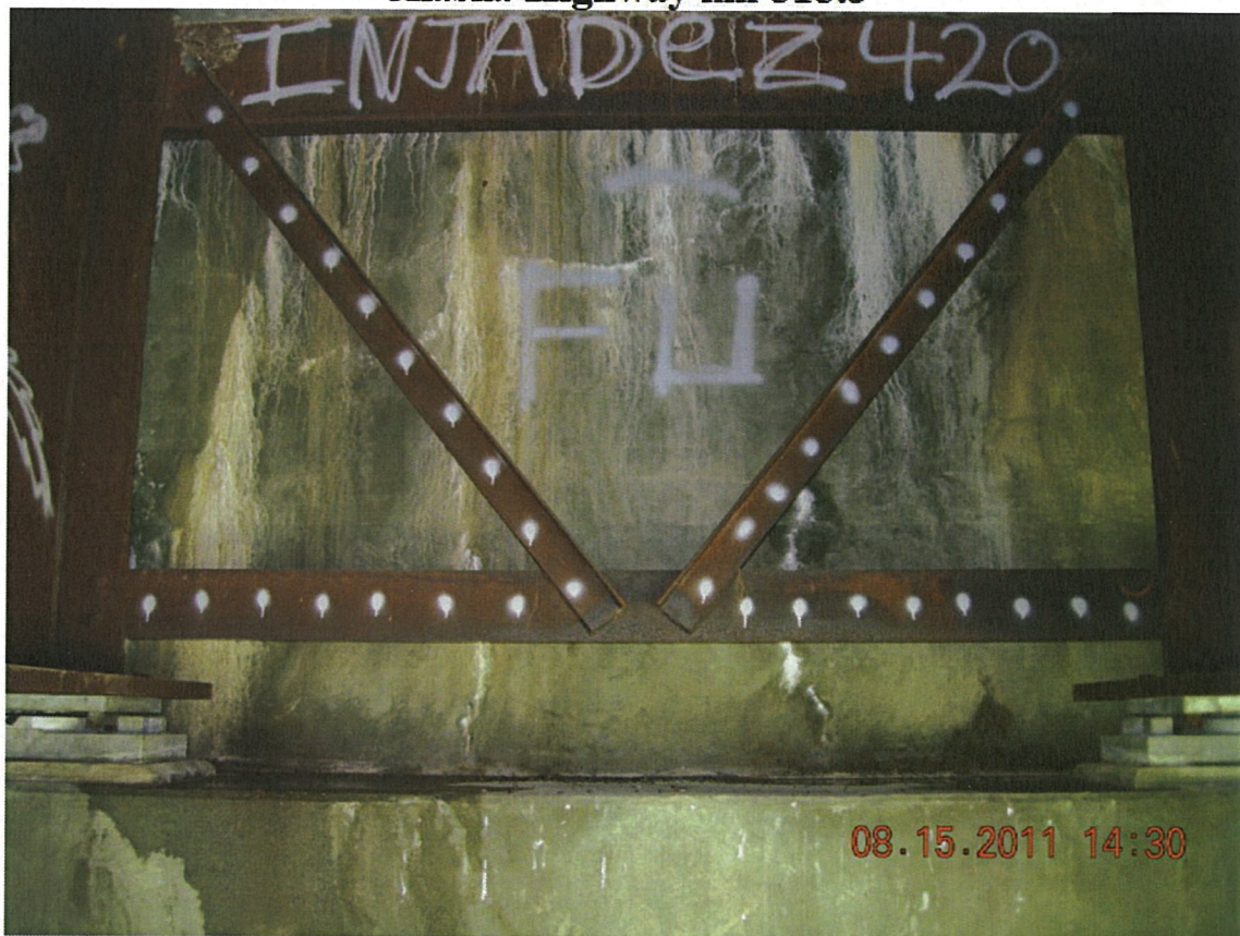
P23 - South Abutment - Backwall - 4 Leaching Narrow Vertical Cracks
