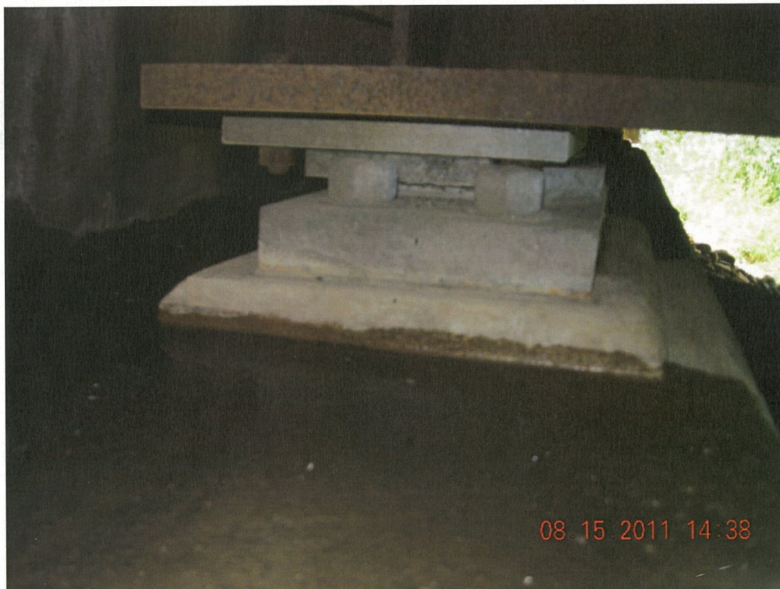
P26 - South Abutment - Expansion Pot Bearing 2 - Water Ponding on Bearing Seat
