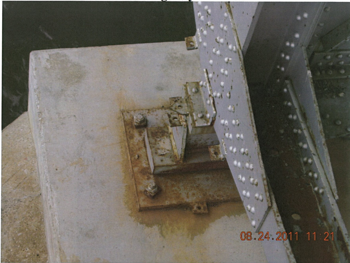
P59 - Pier 2 - East Rocker Bearing - Pier Cap Repaired in 2004 - Light Surface Corrosion Typical
