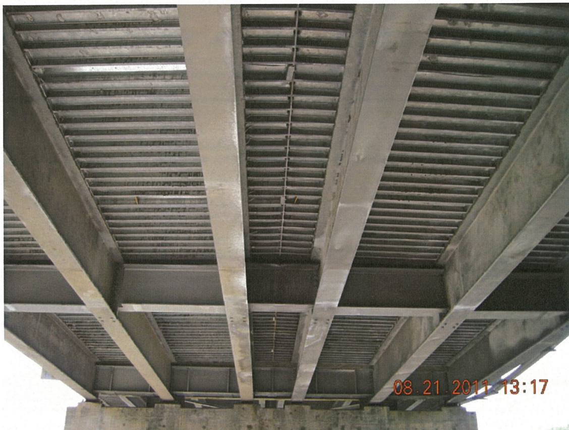
P18 - Span 1 - 6 Galvanized Steel Girders and Orthotropic Steel Deck Soffit
