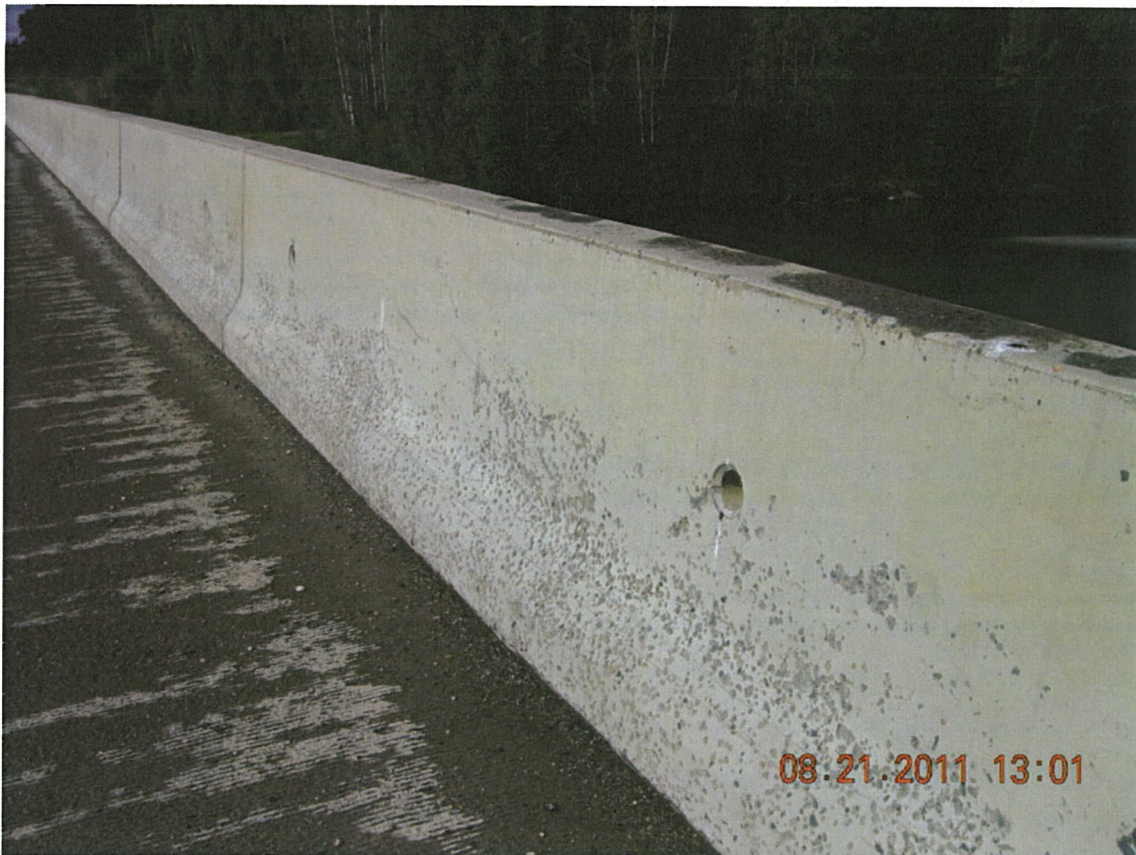
P16 - Concrete Bridge Barriers - Light Scaling in Spray Zone
