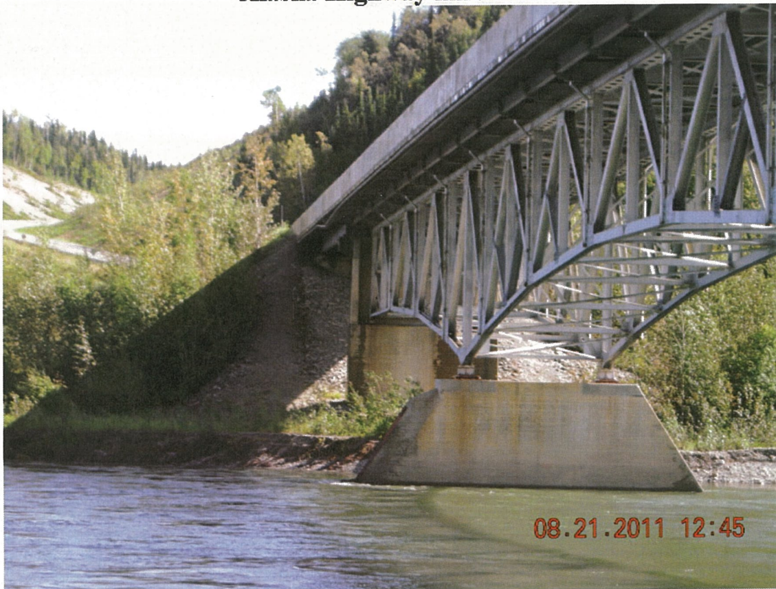
P45 - South Abutment and Embankment - Active Scour on SE Embankment
