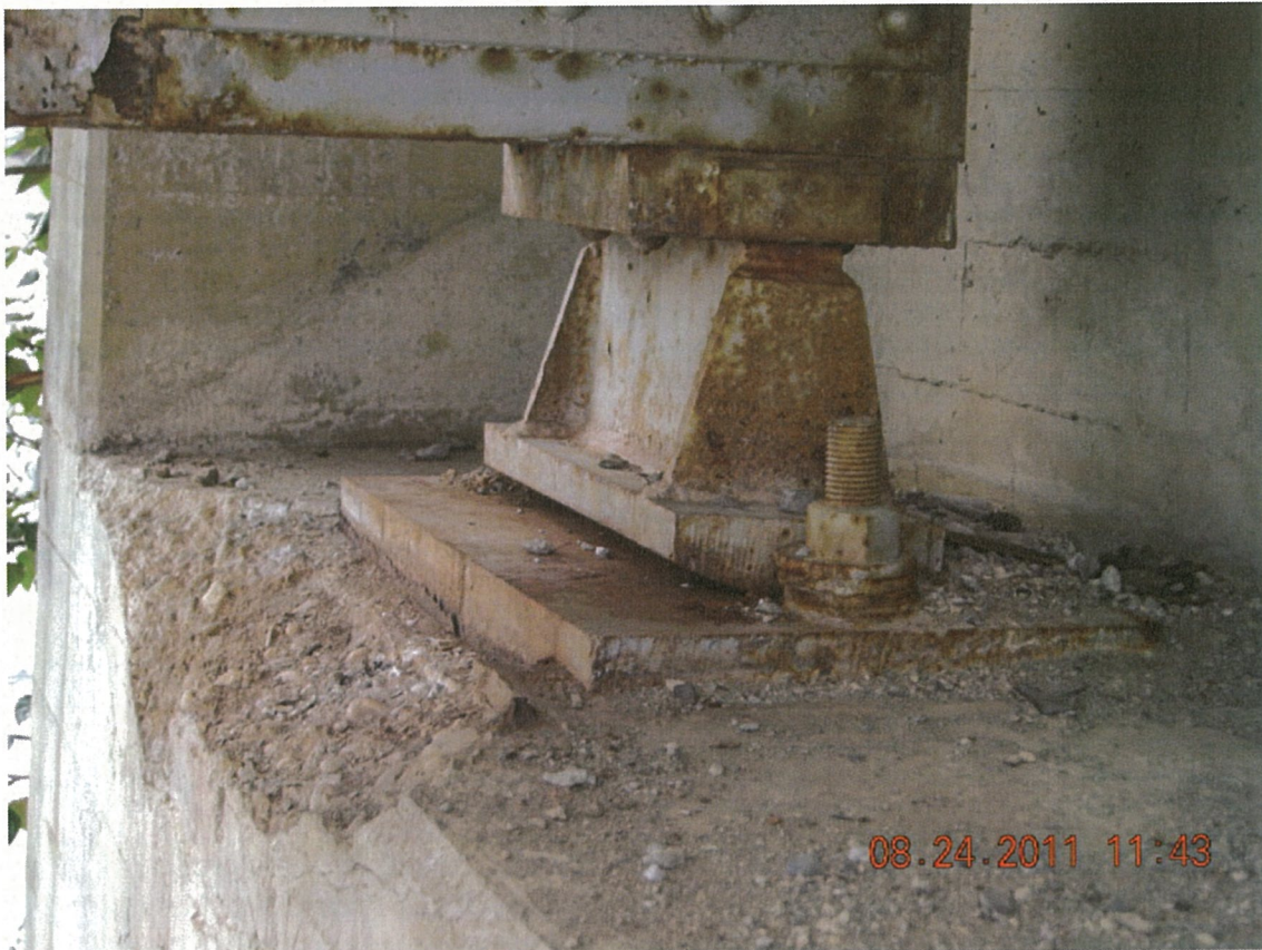
P70 - Pier 4 - Span 4 - West Rocker Bearing - Spalling in Seat Adjacent to Bearing
