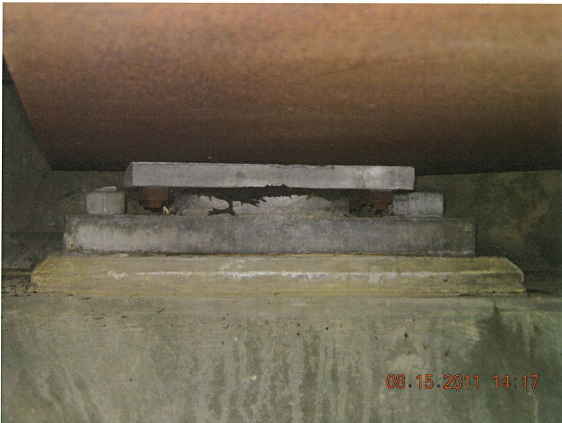
P32 - North Abutment - Fixed Pot Bearing 2 - Neoprene Pads Squeezing Out
