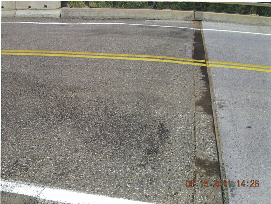
P12 - North Deck Joint - Partially Covered in BST - North Approach Slab Covered in BST
