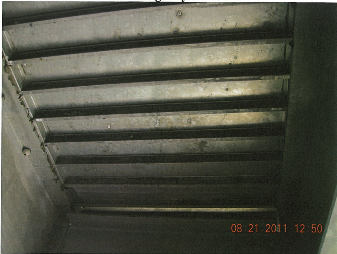
P43 - Galvanized Steel Orthotropic Steel Deck Panel Soffit
