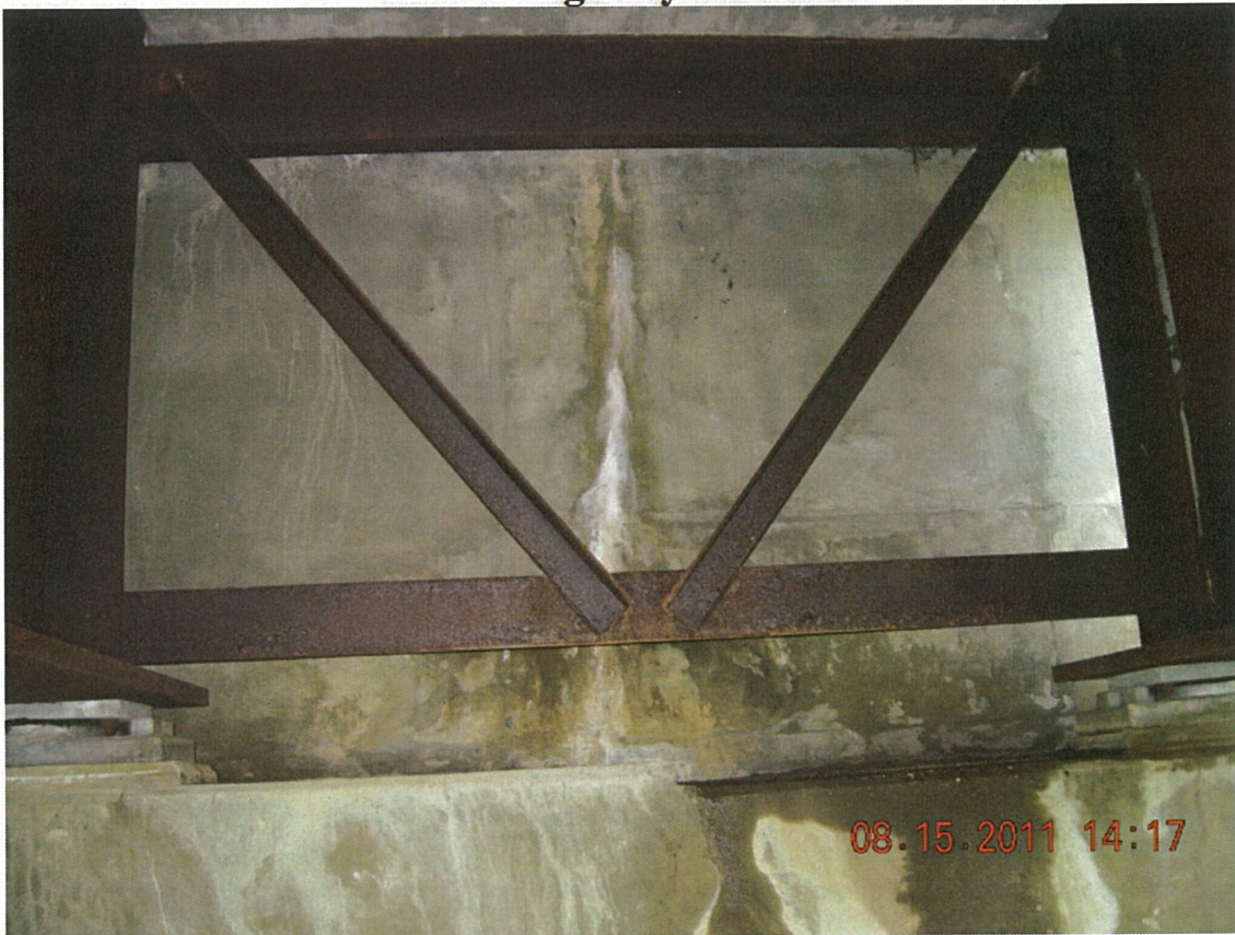
P29 - North Abutment - Backwall - Narrow Vertical Crack Leaching Efflorescence between Girders 1 and 2
