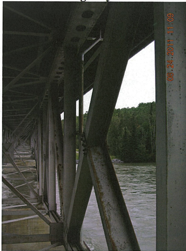
P27 - Span 2 - East Truss - Bay 4 Diagonal and Brace - Light Surface Corrosion Showing Through Paint - Typical
