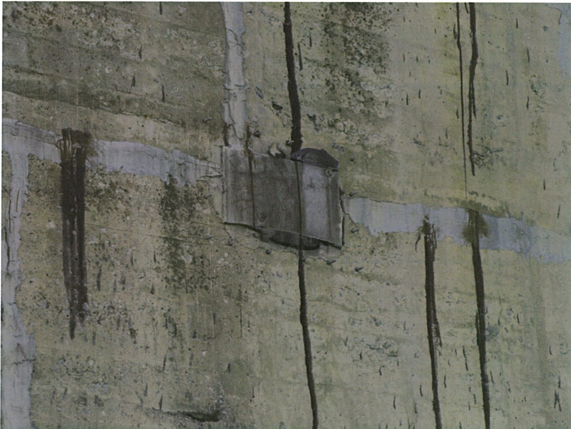
UW04 - Pier 1 Spall repair HC face
