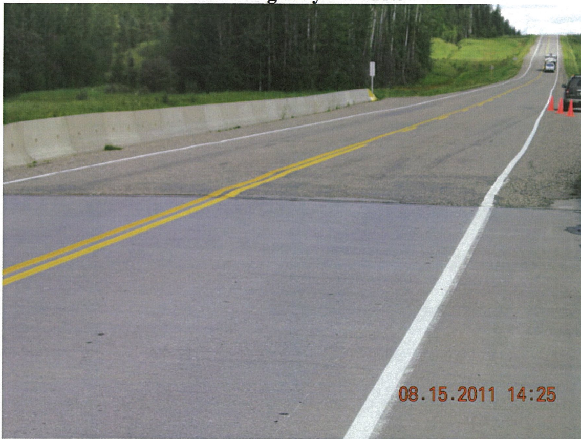
P07 - South Approach Uneven at Bridge
