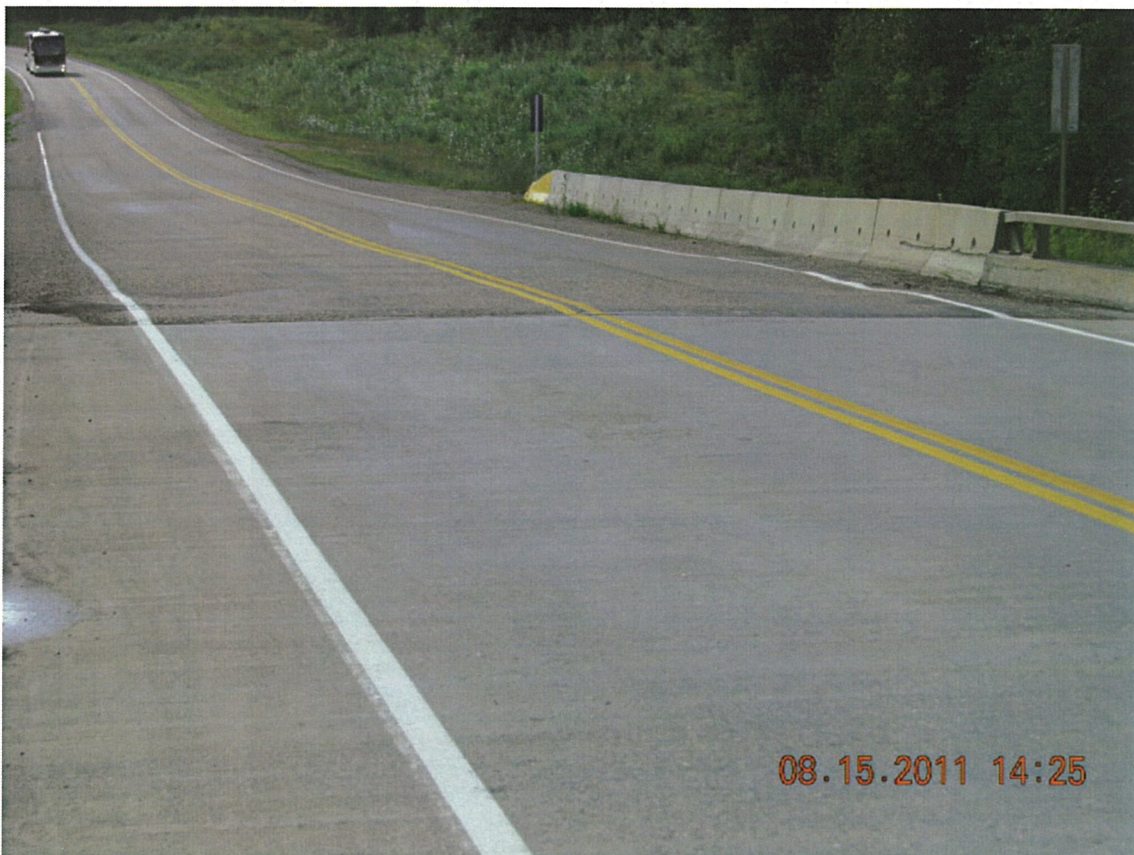
P08 - North Approach Uneven at Bridge
