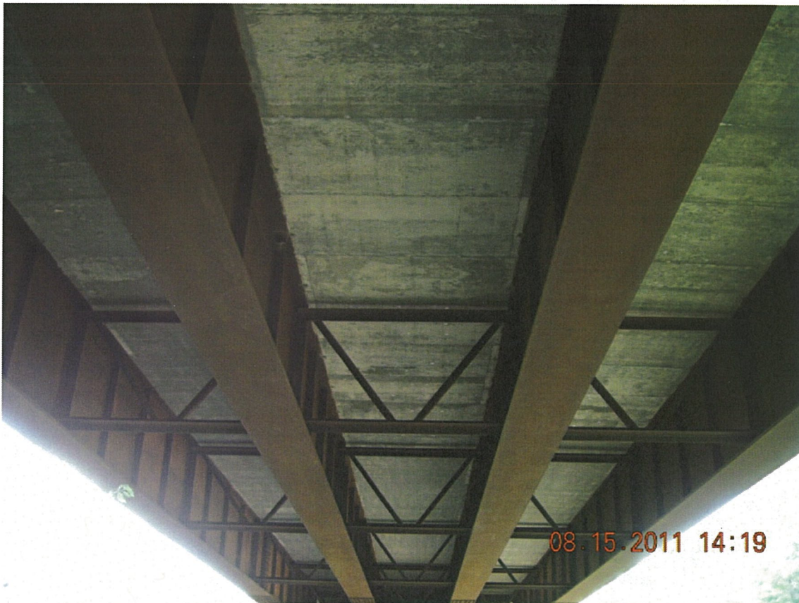
P16 - Soffit and 4 Weathering Steel I Girders - No Staining on Soffit - Looking North
