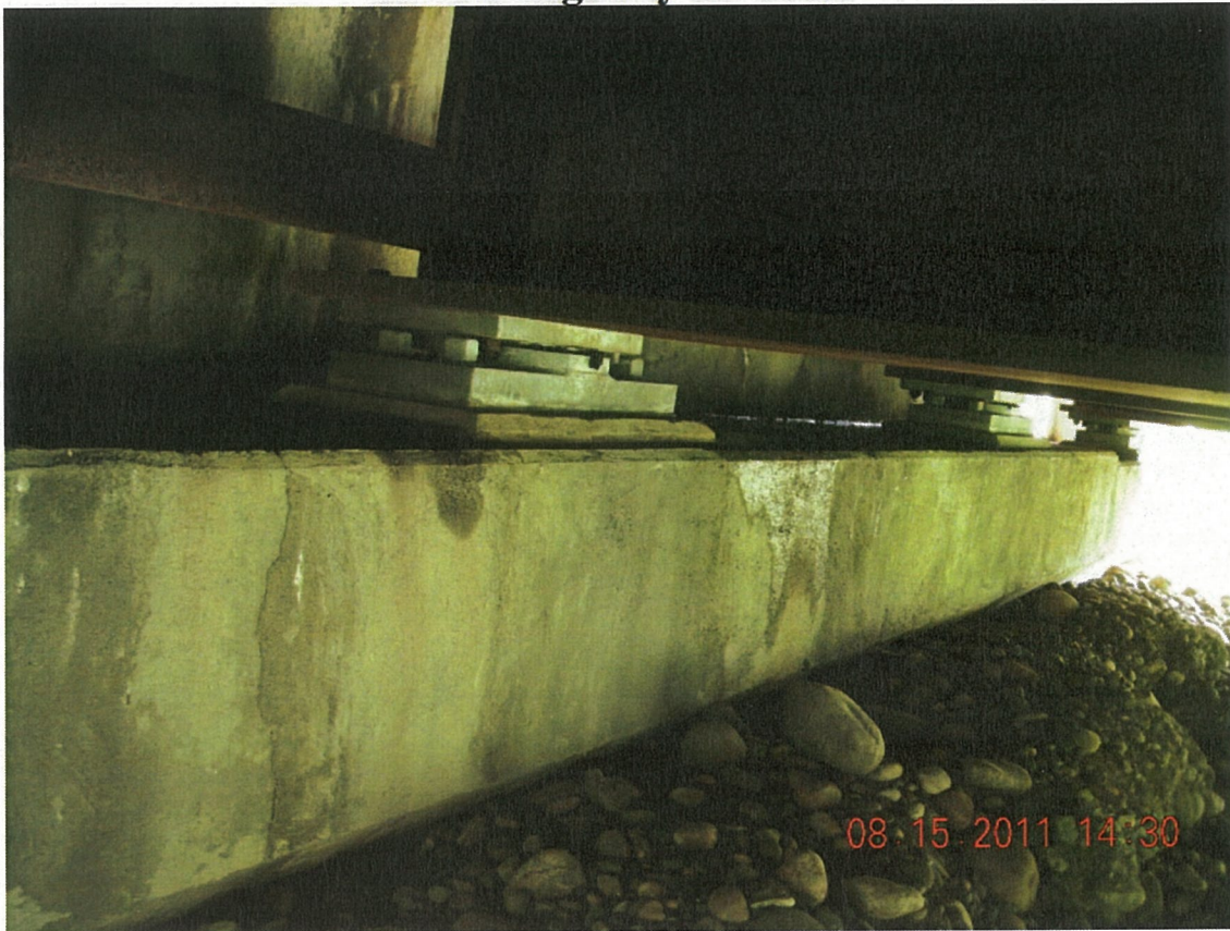
P25 - South Abutment - Bearing Seat Wet - Expansion Pot Bearings
