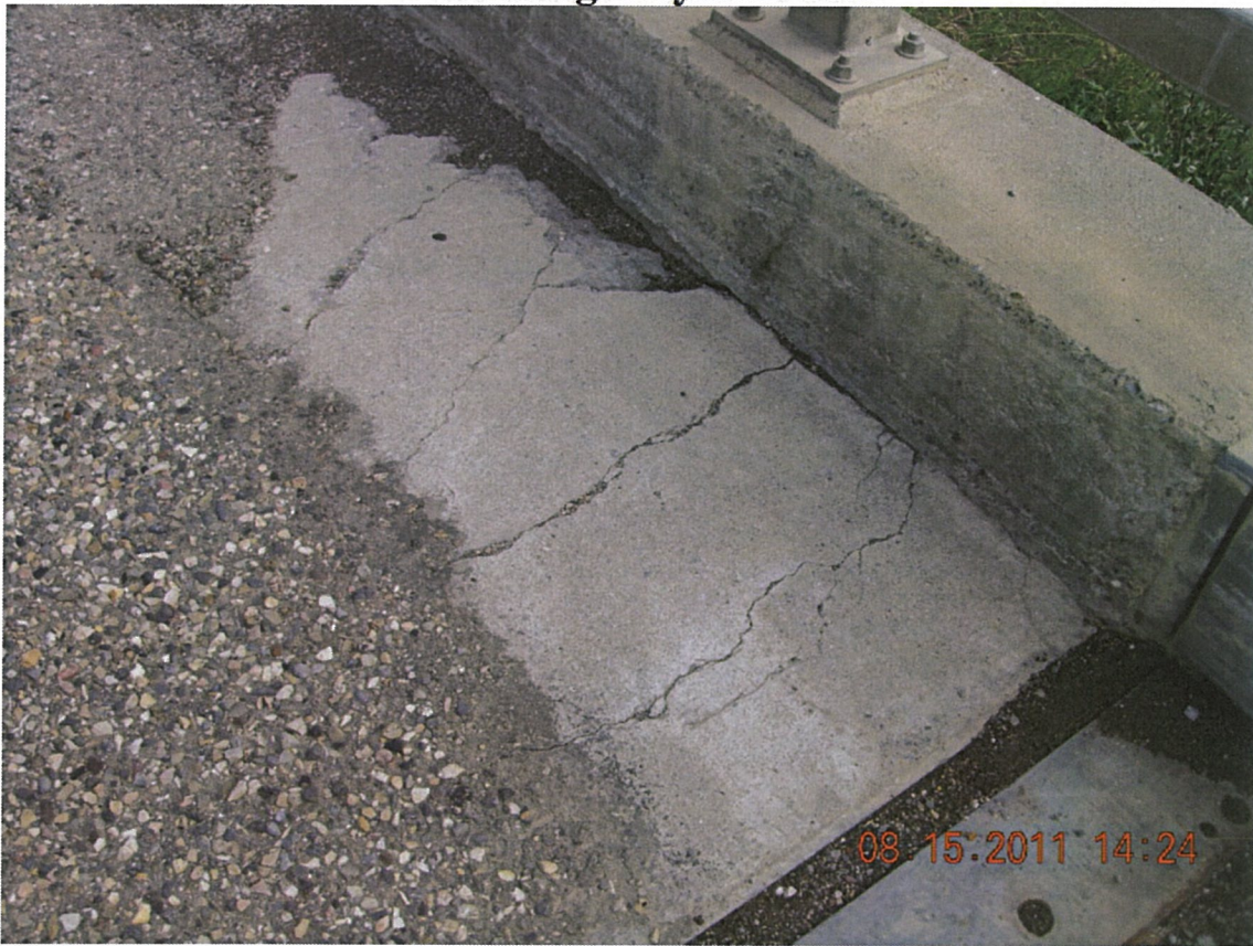
P11 - South Approach Slab - Wide Transverse Cracks in Approach Slab where Exposed at Both Curbs
