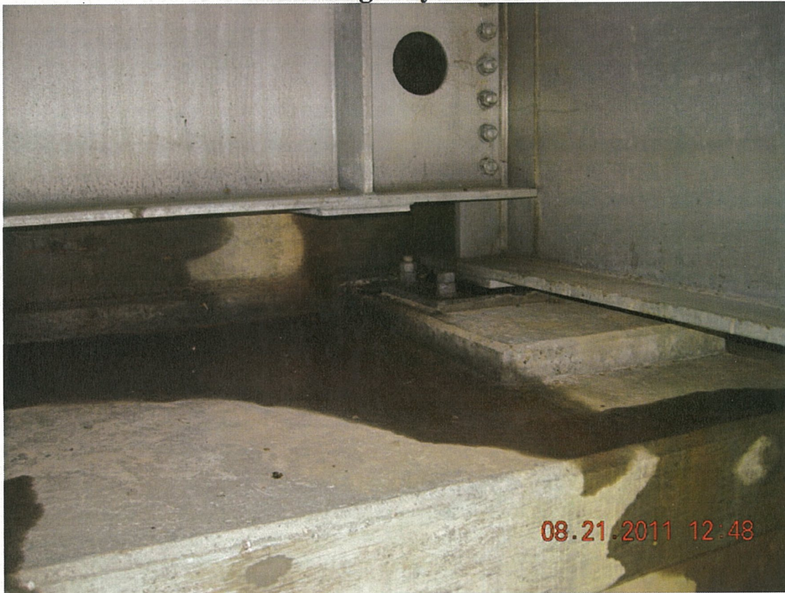
P73 - North Abutment - Span 5 - Neoprene Bearing 2 - Moisture Seeping Through Deck Joint
