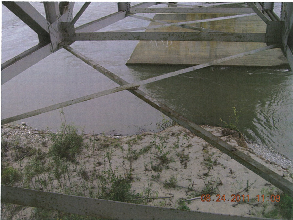
P24 - Span 2 - Bay 2 - Lower Sway Bracing
