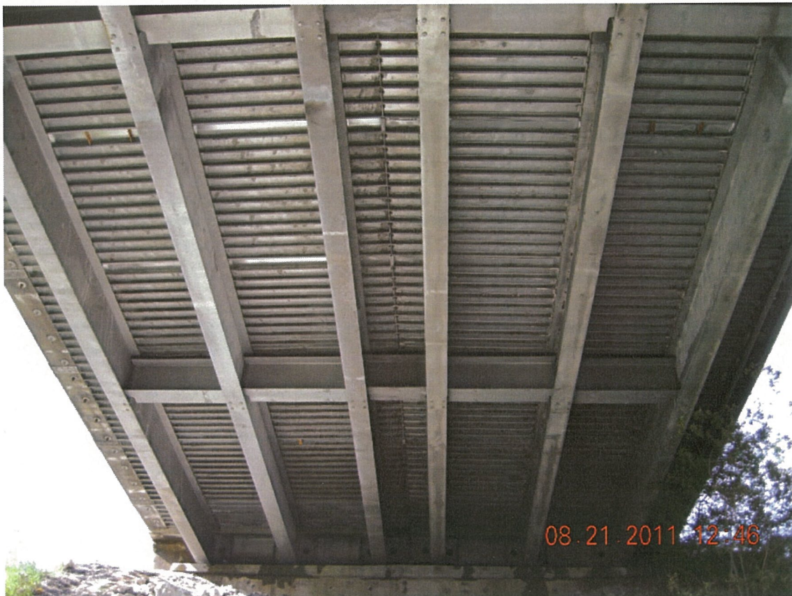
P42 - Span 5 - 6 Galvanized Steel Girders and Orthotropic Steel Deck Soffit
