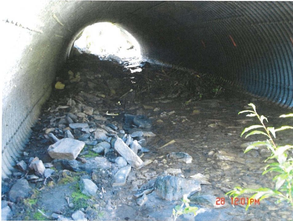
20.1 – Clean the Tree Debris and Branches Inside of Barrel, at Outlet and in the Creek
