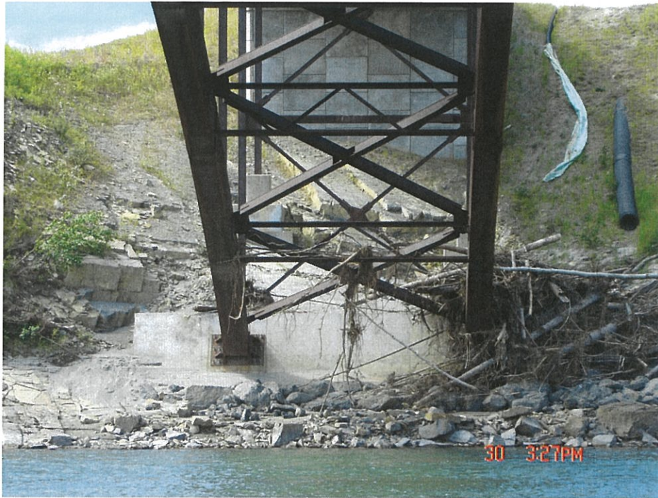
32.1 – Clear Debris and Branches from the Blocks and Bracing
