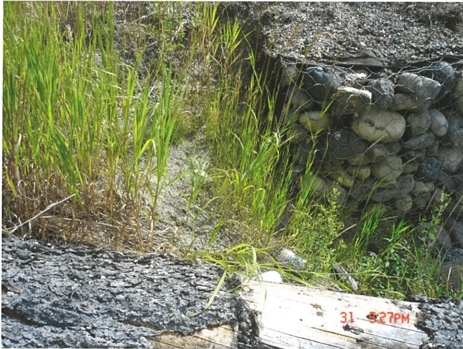
37.1 – Repair Erosion Above Gabion Walls
