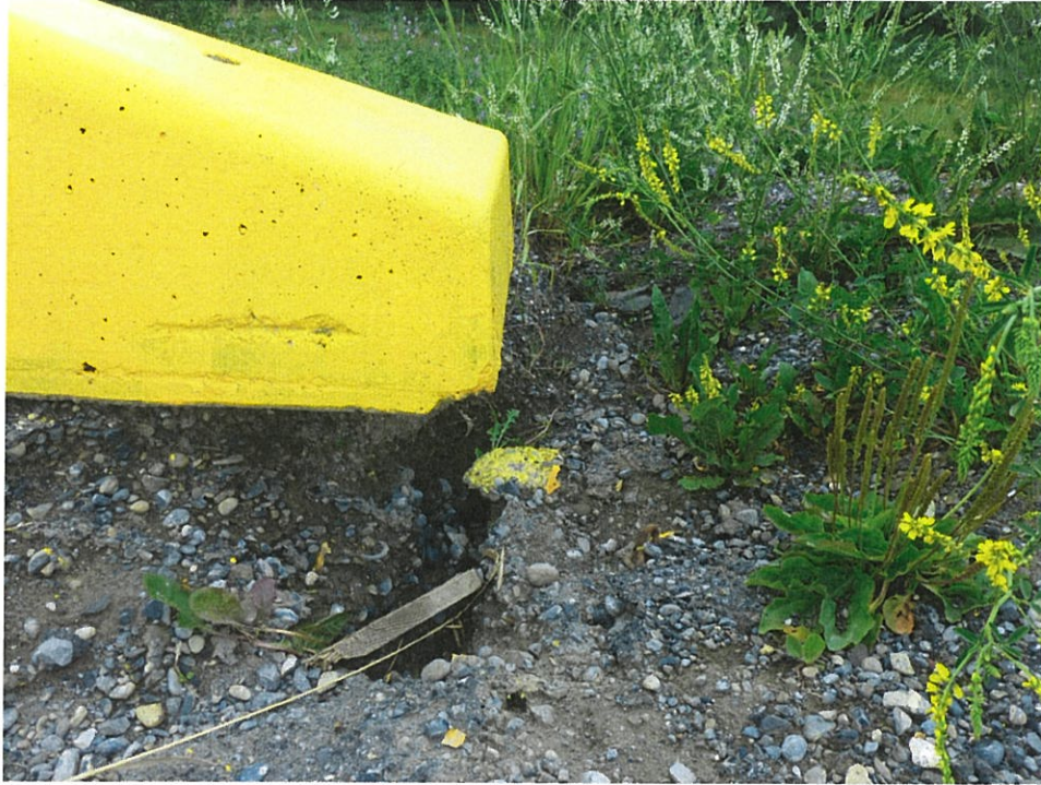
1.1 - Repair Embankment Erosion at NW Corner
