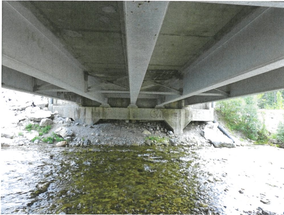
18.1 – Place RipRap in Front of South Abutment
