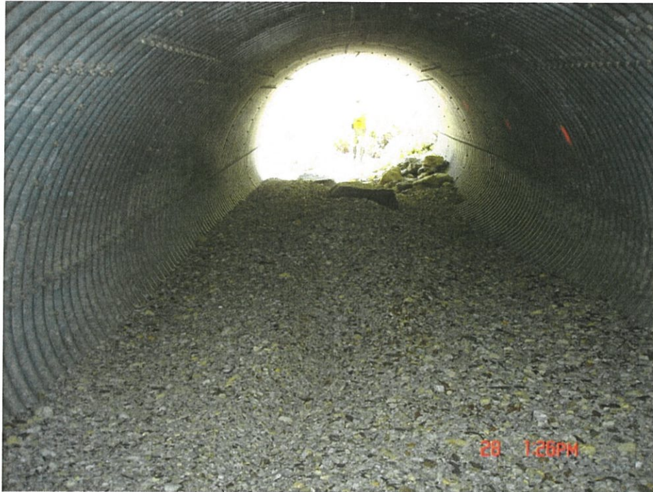
23.1 – Remove Large Rock from Culvert
