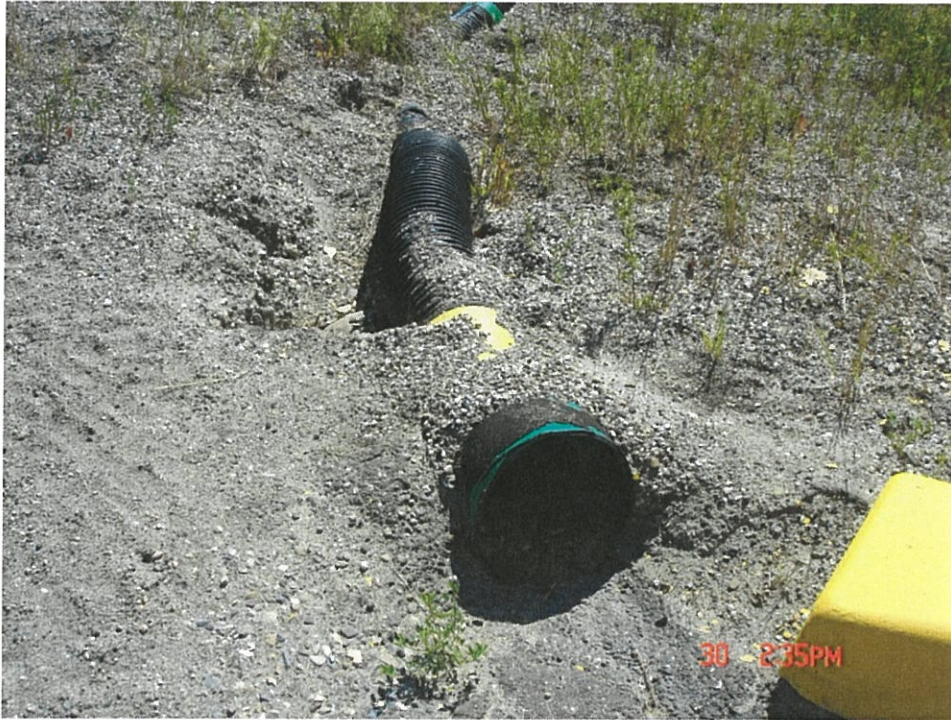
32.3 – Install RipRap at SW Embankment Drain Area
