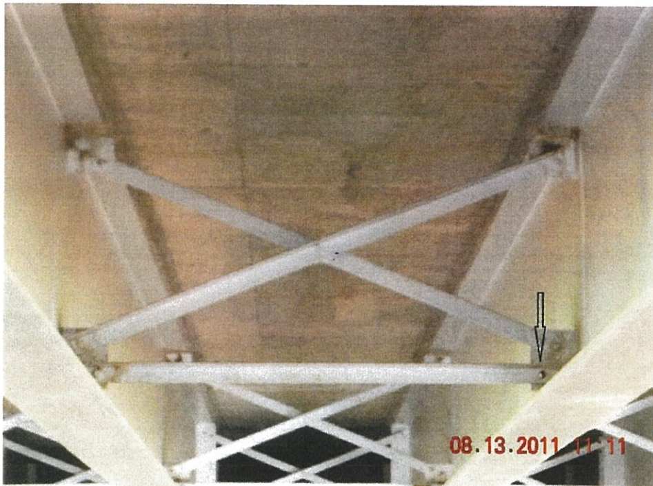
1.2 - Install Missing Diaphragm Bolt
