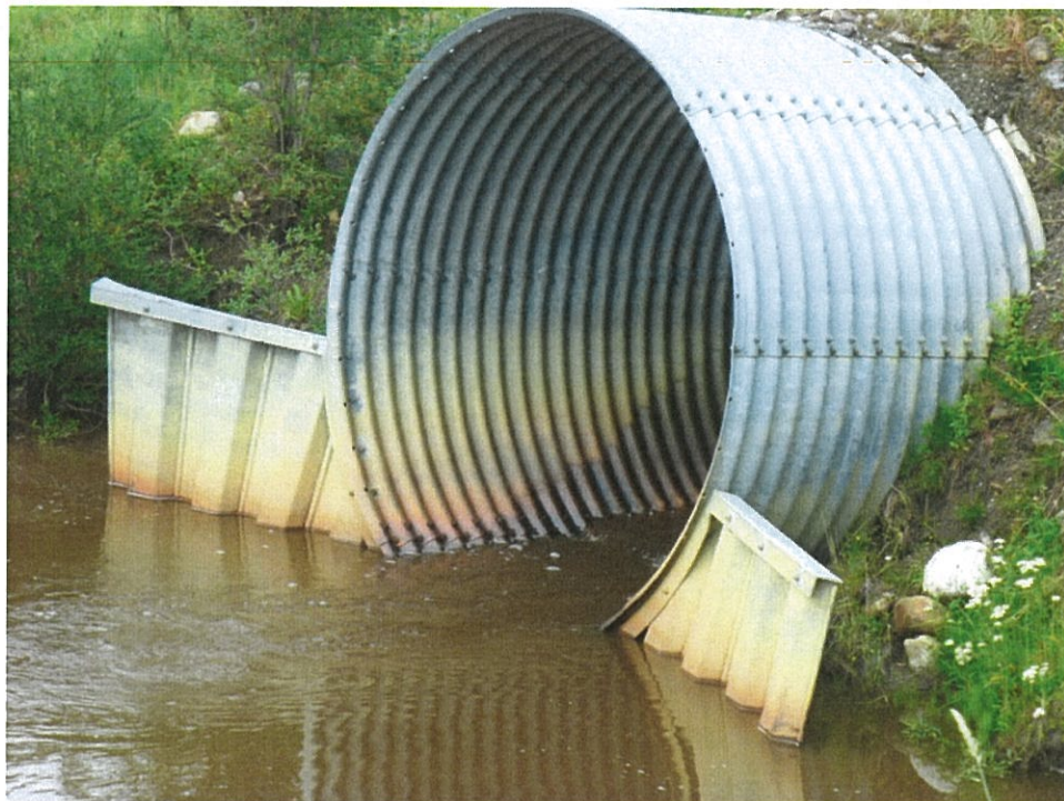
2.2 - Backfill the Outlet Binwalls
