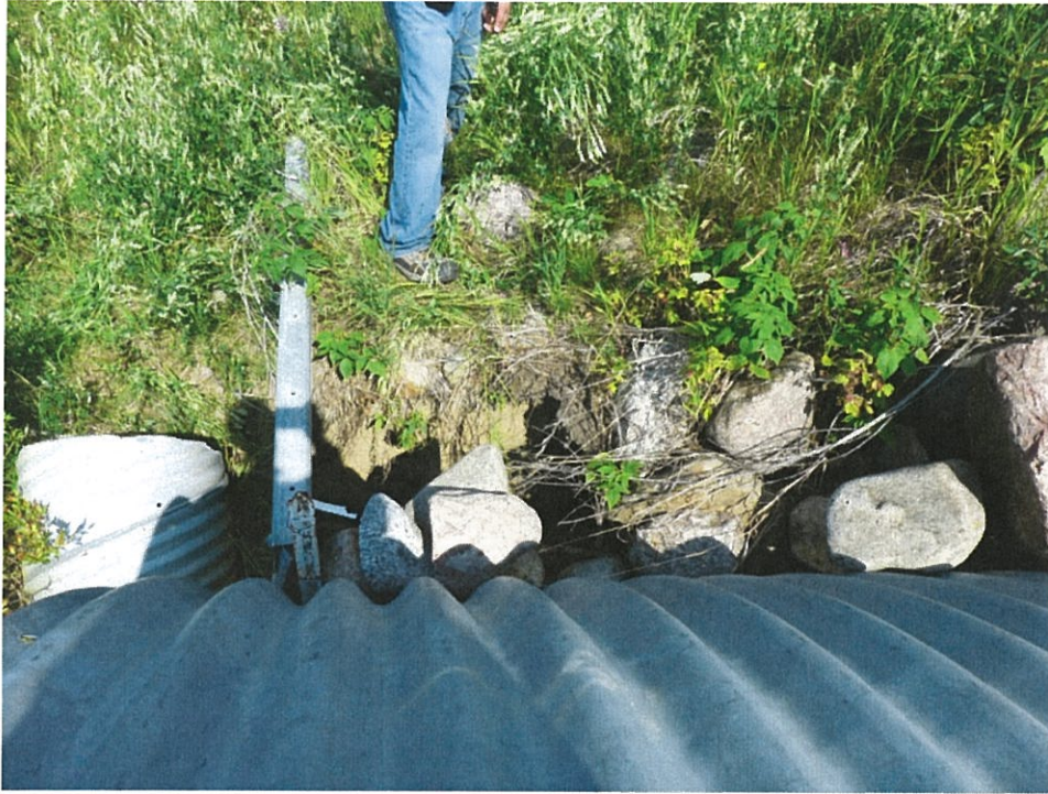
8.3 – Backfill Behind the Binwalls of the Inlet and Outlet
