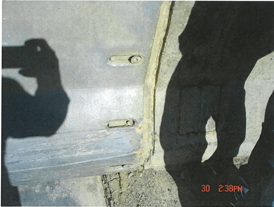
33.1 – Replace Broken Bolt in Barrier Cover Plate
