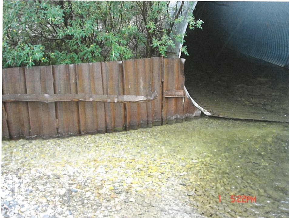
17.1 – Place Fill and RipRap Around the Outlet of the Pipe
