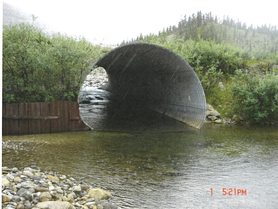
17.2 – Place Fill and RipRap Around the Outlet of the Pipe
