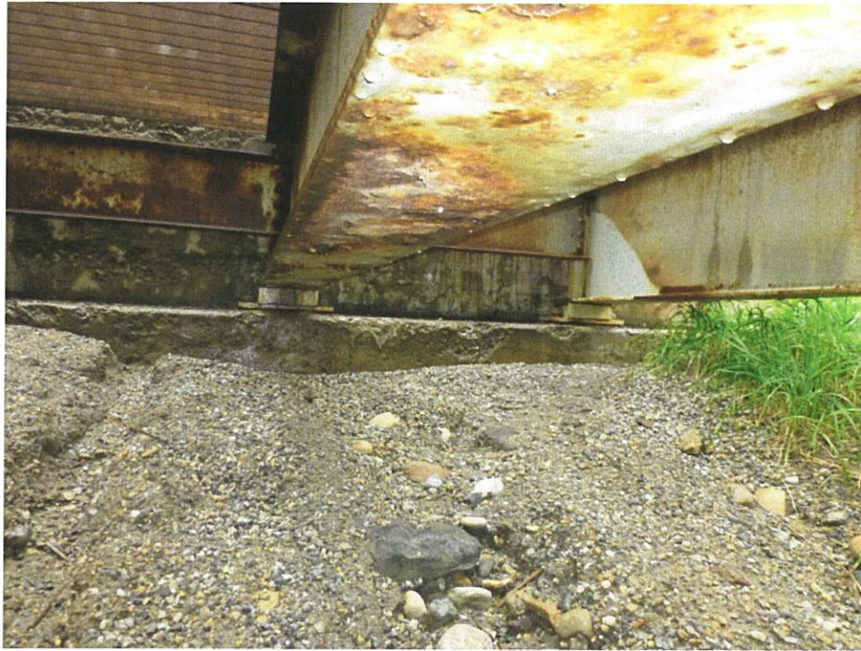
15.1 – Repair Spalling on South Abutment (Details located in Appendix B)
