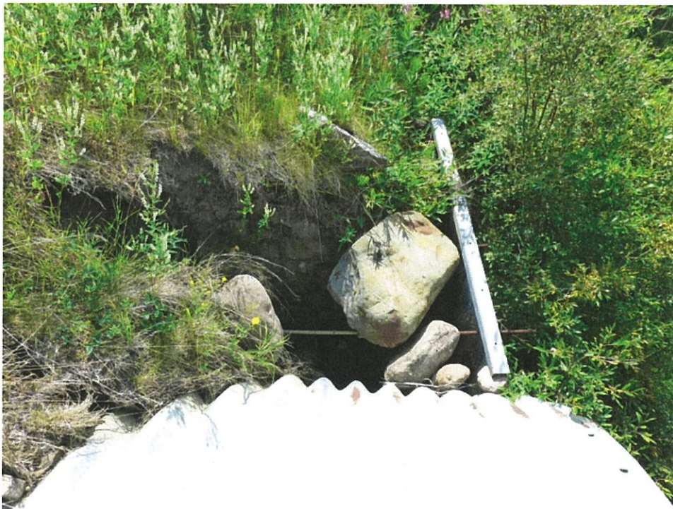
8.4 – Backfill Behind the Binwalls of the Inlet and Outlet
