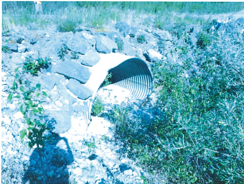
23.2 – Remove Bushes in Front of Inlet
