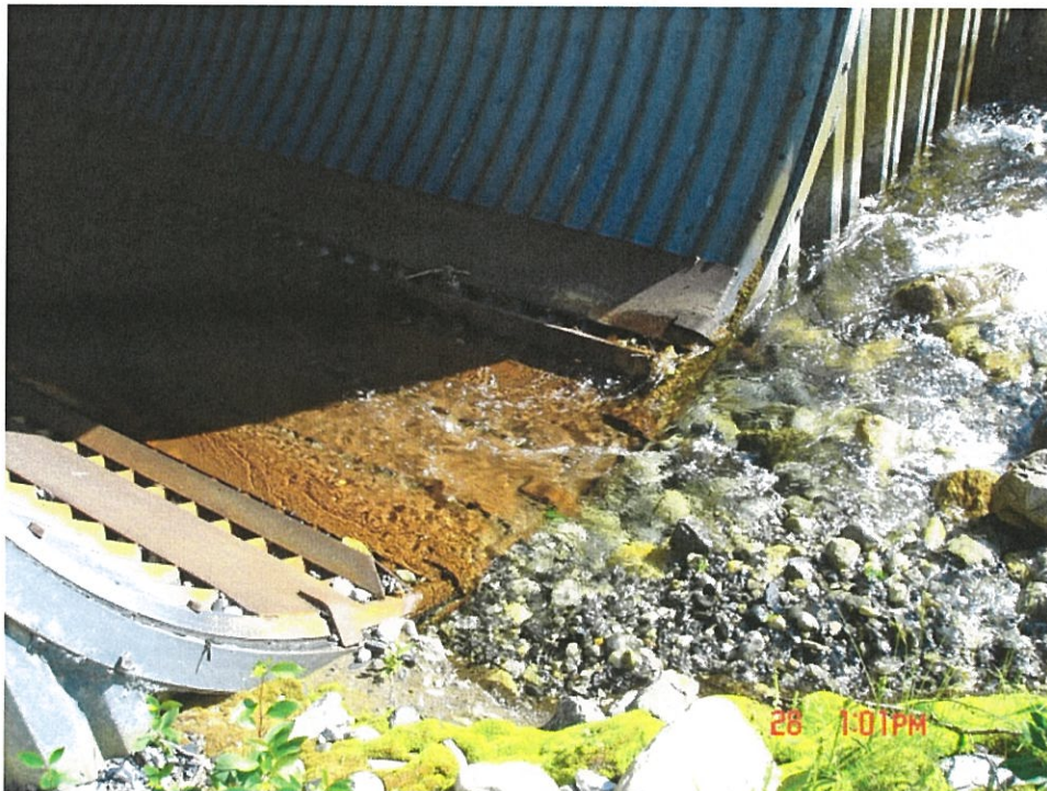
22.2 – Align Stream with Culvert Inlet
