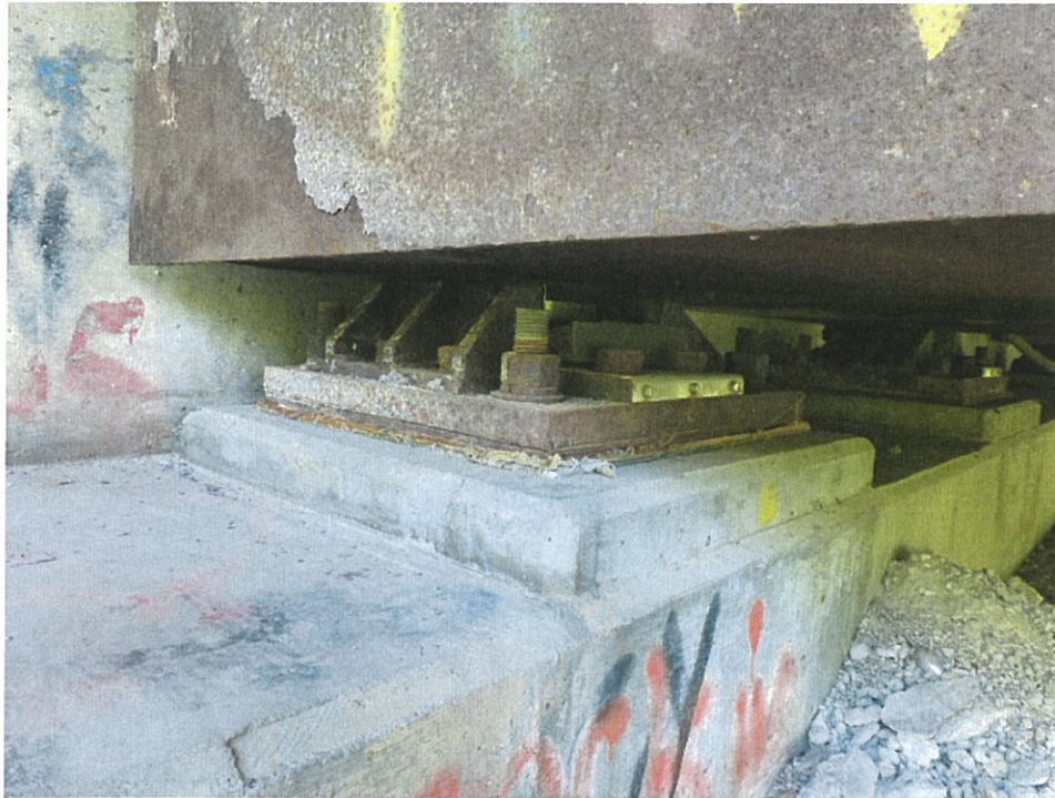
11.3 – Replace Bearing Covers, to match existing
