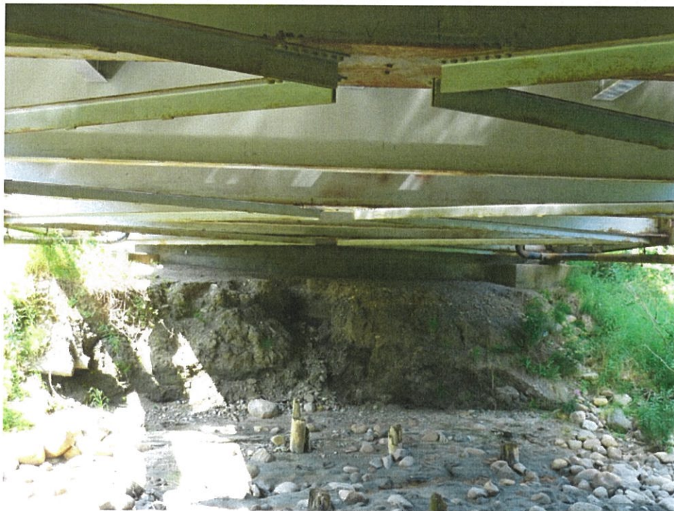
10.2 – Fill Gulleys in Embankment under North Abutment
