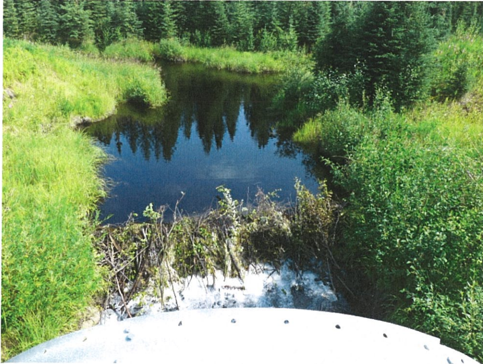
7.1 – Remove Beaver Dam Upstream of Inlet
