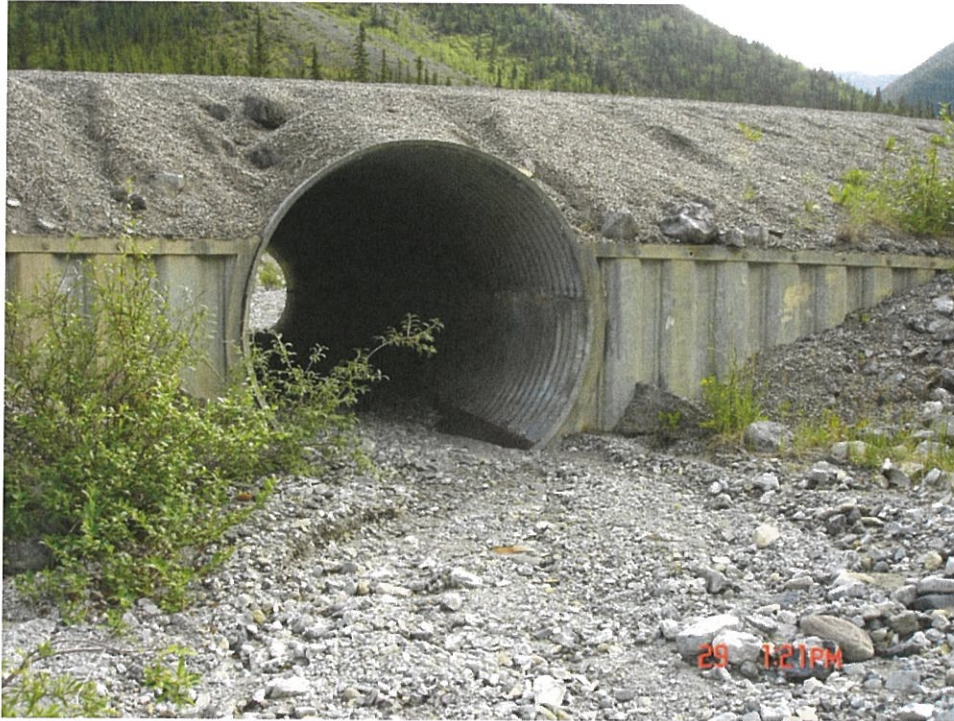
28.1 – Repair Shoulder Erosion
