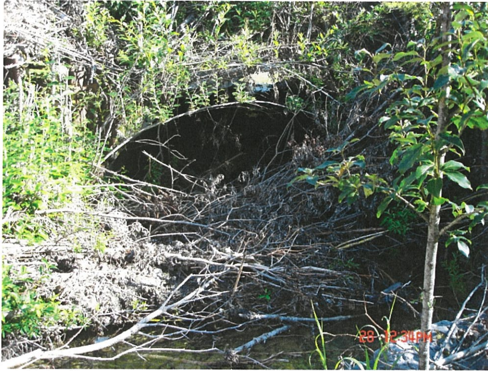
21.1 - Clear Larger Branches and Debris in the Inlet and on Embankment
