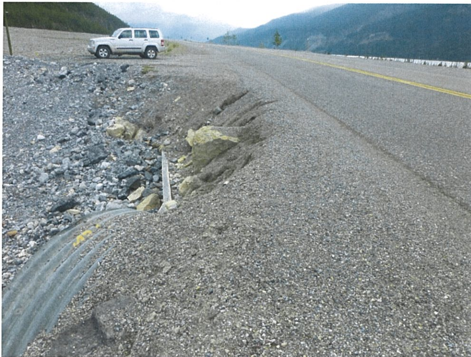
25.2 – Repair Embankment at the SE Shoulder
