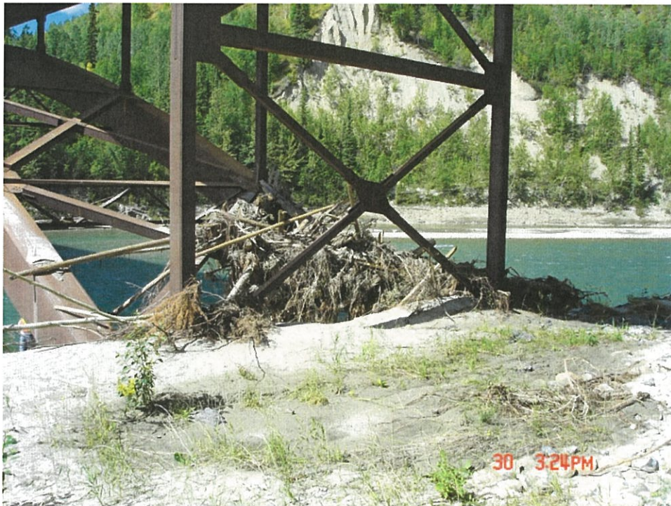
32.4 – Clear Sand Drift from Both Arch Legs
