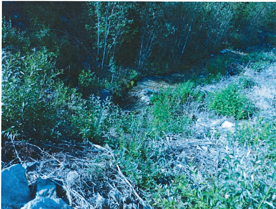
21.2 - Clear Larger Branches and Debris in the Inlet and on Embankment
