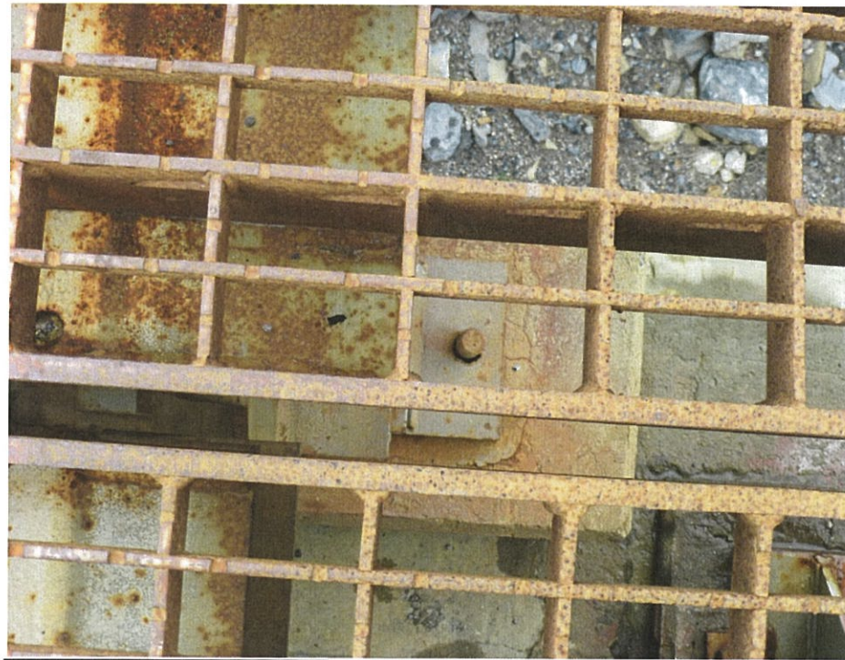
19.2 – Replace Missing Bearing Anchor Nuts
