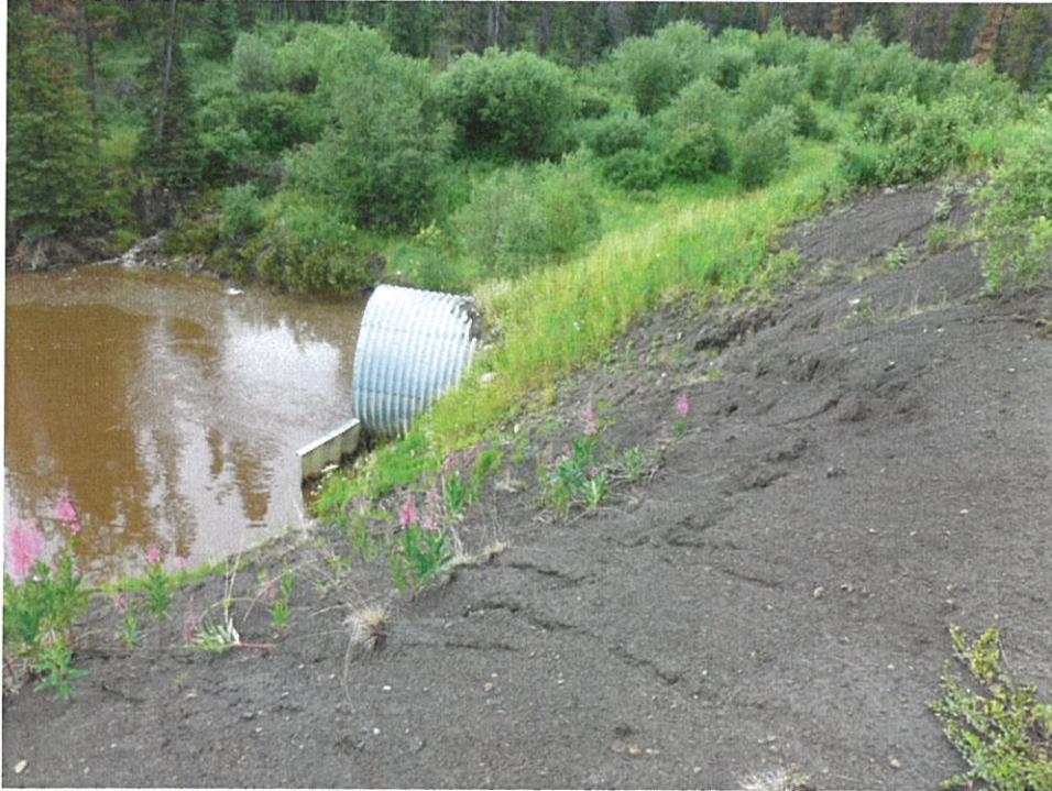
2.1 - Backfill the Outlet Binwalls
