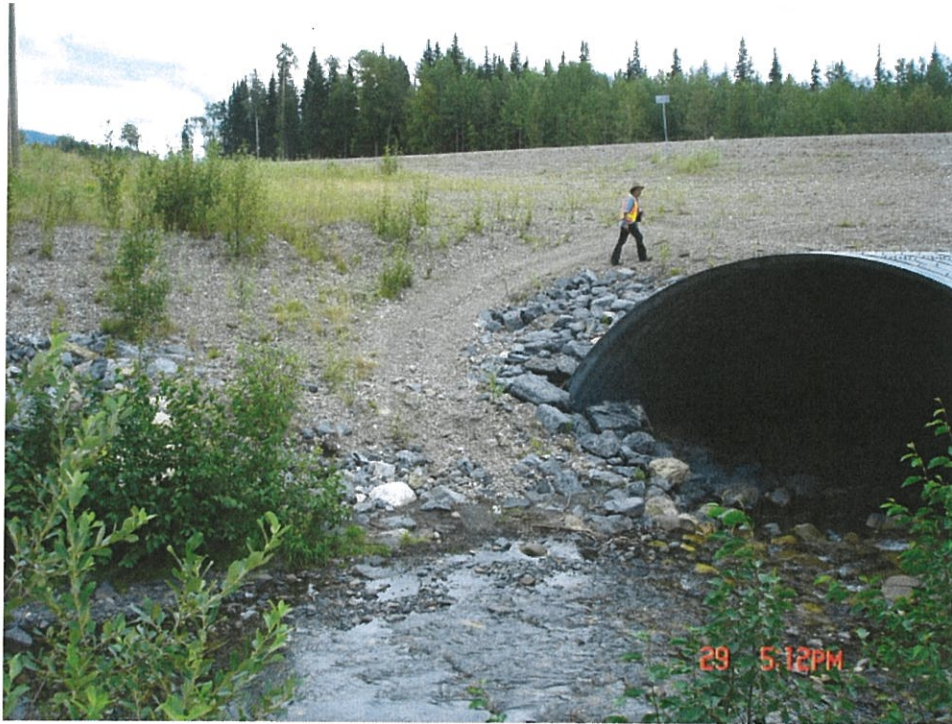
30.1 – Install RipRap at SE of Inlet to Protect the Inlet
