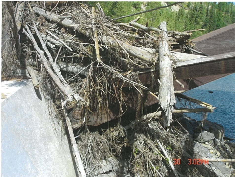
32.2 – Clear Debris and Branches from the Blocks and Bracing
