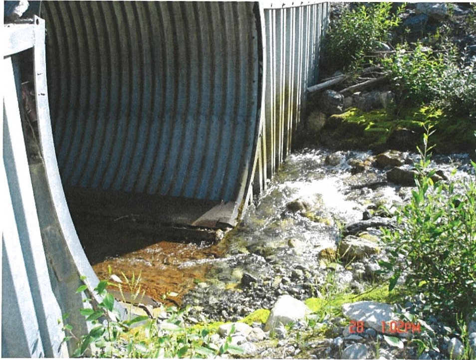
22.1 – Align Stream with Culvert Inlet
