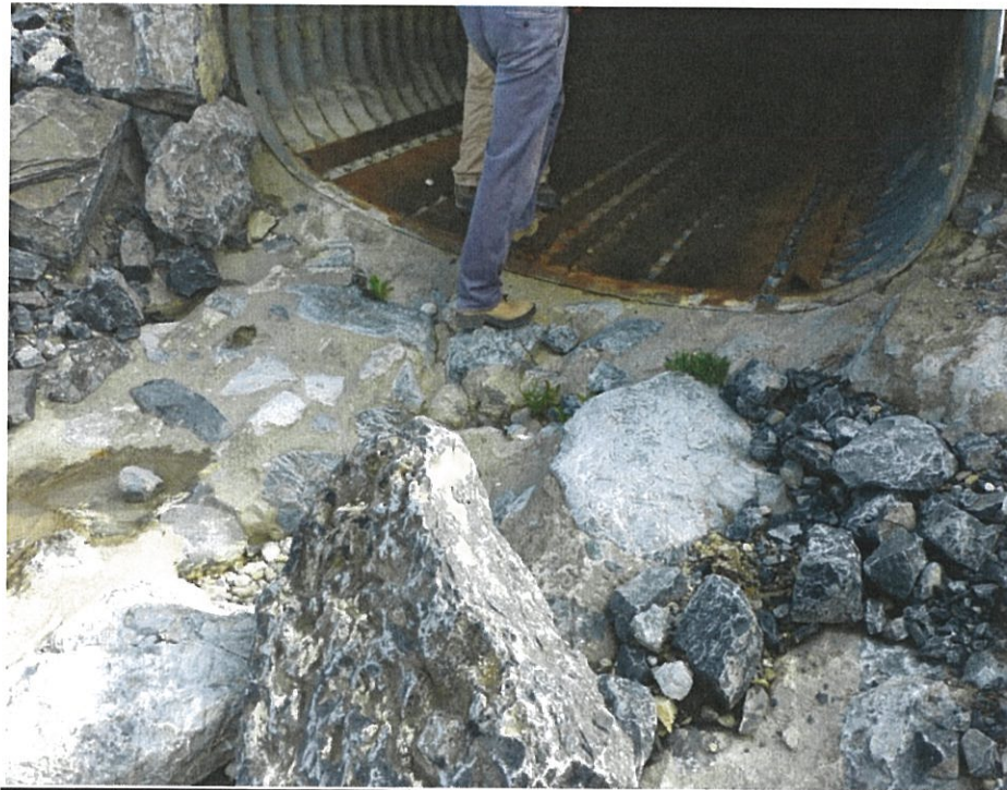
27.2 – Fill Scour Hole at Outlet with Concrete
