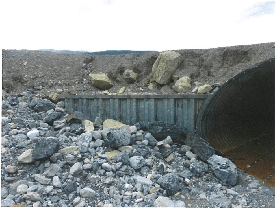
25.1 – Repair Embankment at the SE Shoulder
