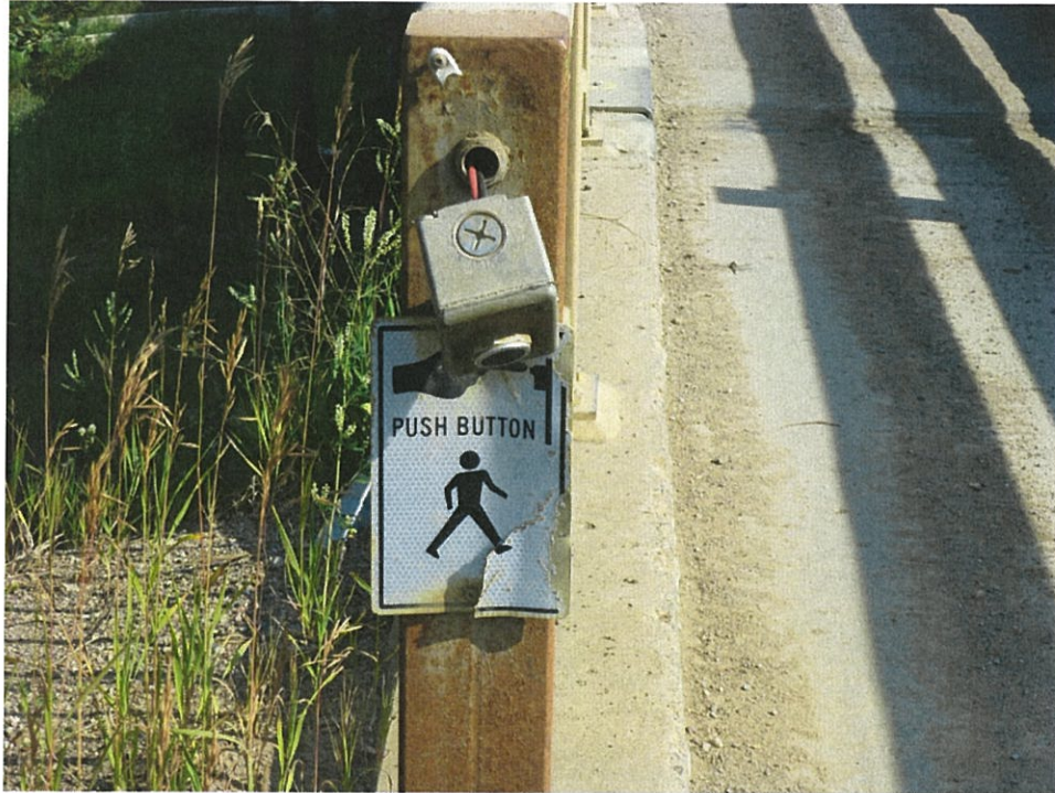
11.1 – Repair Pedestrian Switch
