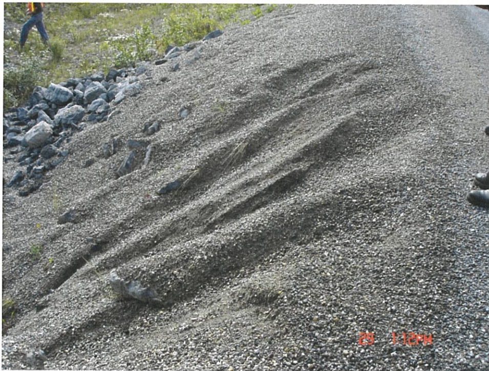
28.2 – Repair Shoulder Erosion
