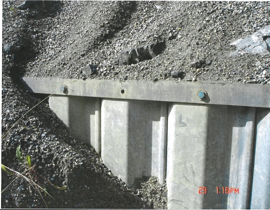
28.3 – Replace Missing Binwall Bolts
