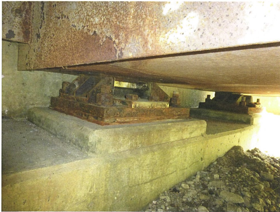
11.4 – Replace Bearing Covers, to match existing
