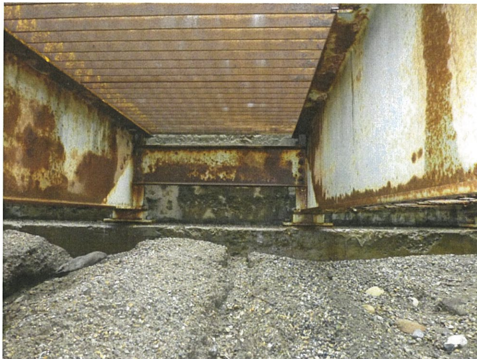
15.2 – Repair Spalling on South Abutment (Details located in Appendix B)
