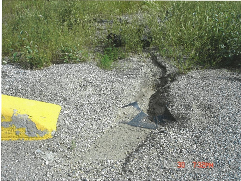
36.1 – Repair NW Erosion and Embankment Drain
