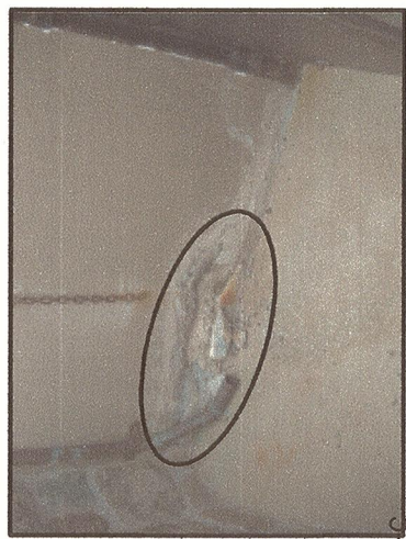
PHOTO 8: CONCRETE REPAIR (± 0.028 M²)
