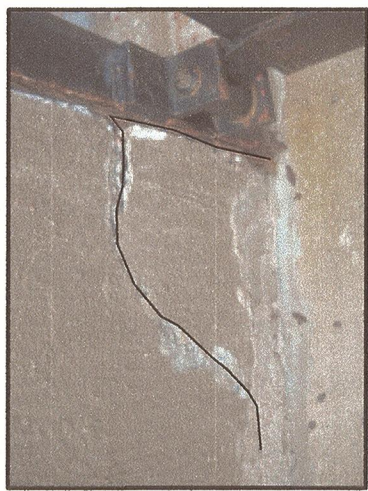
PHOTO 7: SURFACE CRACK (± 0.400 LM)
