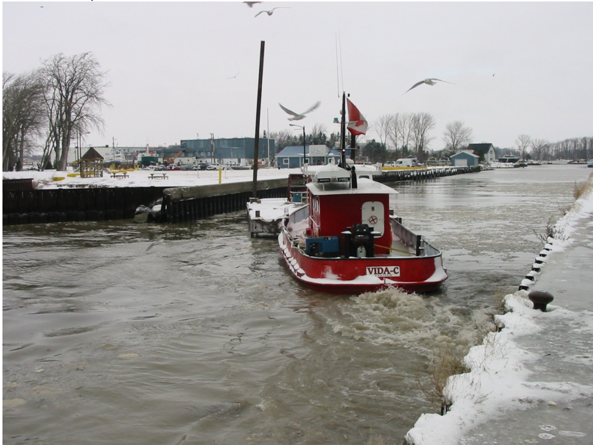
Photo 1 Propeller Wash Dredging within the Entrance Channel December 17, 2008
