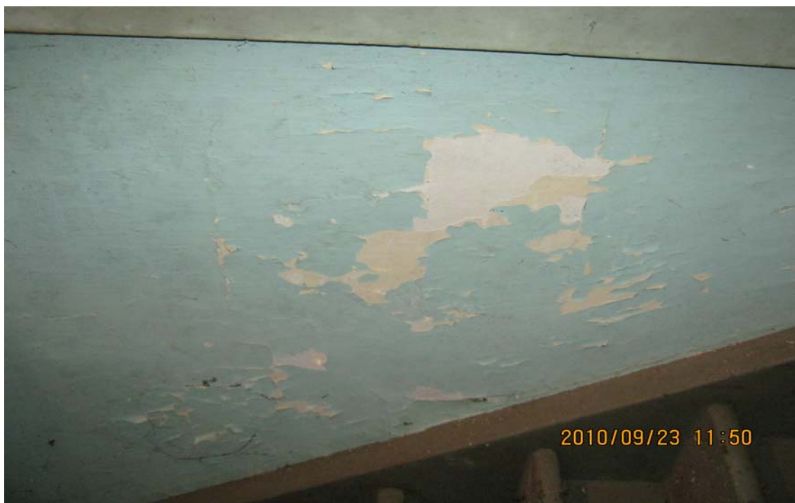
Photo 5: View of teal paint in main floor stairwell, sample L.H LS-3 was found to be above criteria and is considered lead based.
