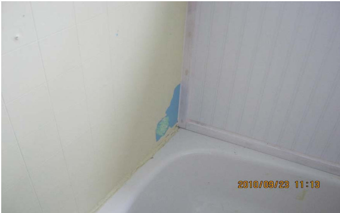
Photo 7: View of peeling paint in bathroom in residence building, sample R.B LS-8 was found to be below criteria and is considered non-lead based.
