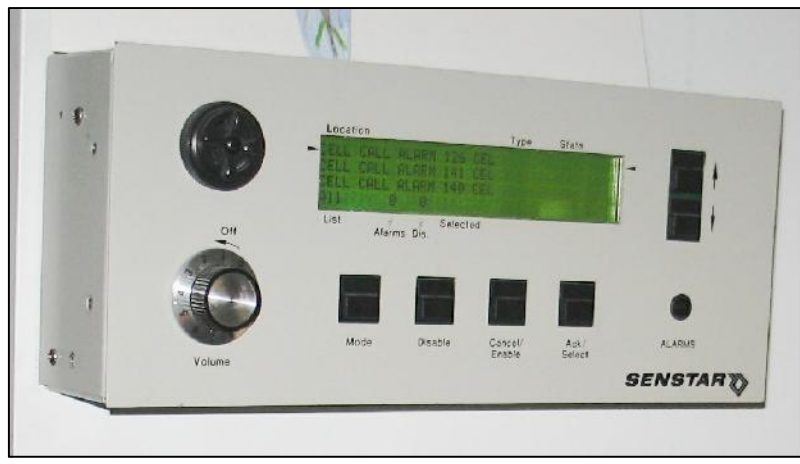
SENSTAR REMOTE DISPLAY & CONTROL PANEL (RCP) (STAFF AREA 117)
