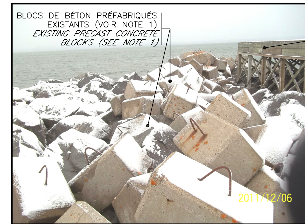
STRUCTURE DE L'HELIPORT EXISTANT A DEMOLIR EXISTING HELIPORT STRUCTURE TO BE DEMOLISHED LOCS DE BTON PREFABRIQUES EXISTANTS (VOIR NOTE 1) EXISTING PRECAST CONCRETE BLOCKS (SEE NOTE 1)
