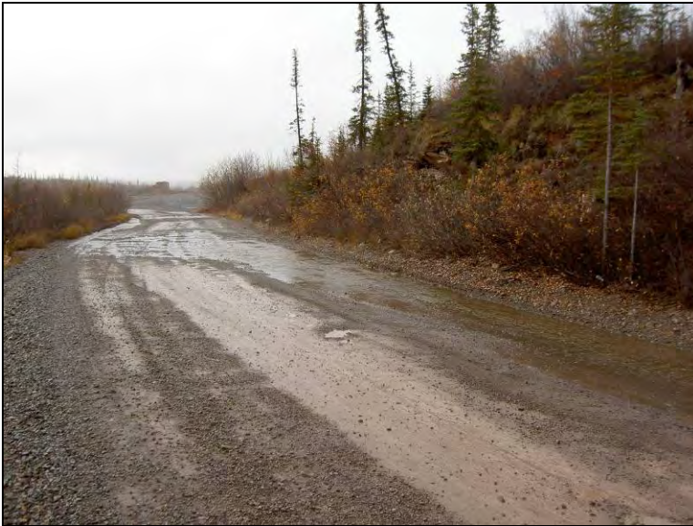
Photo 1.3: Section with potholes, just north of quarry.
