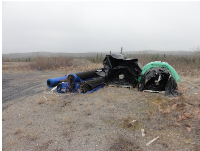
Photograph 5 - Rolls of Enviro-liner and thicker geo-textile
