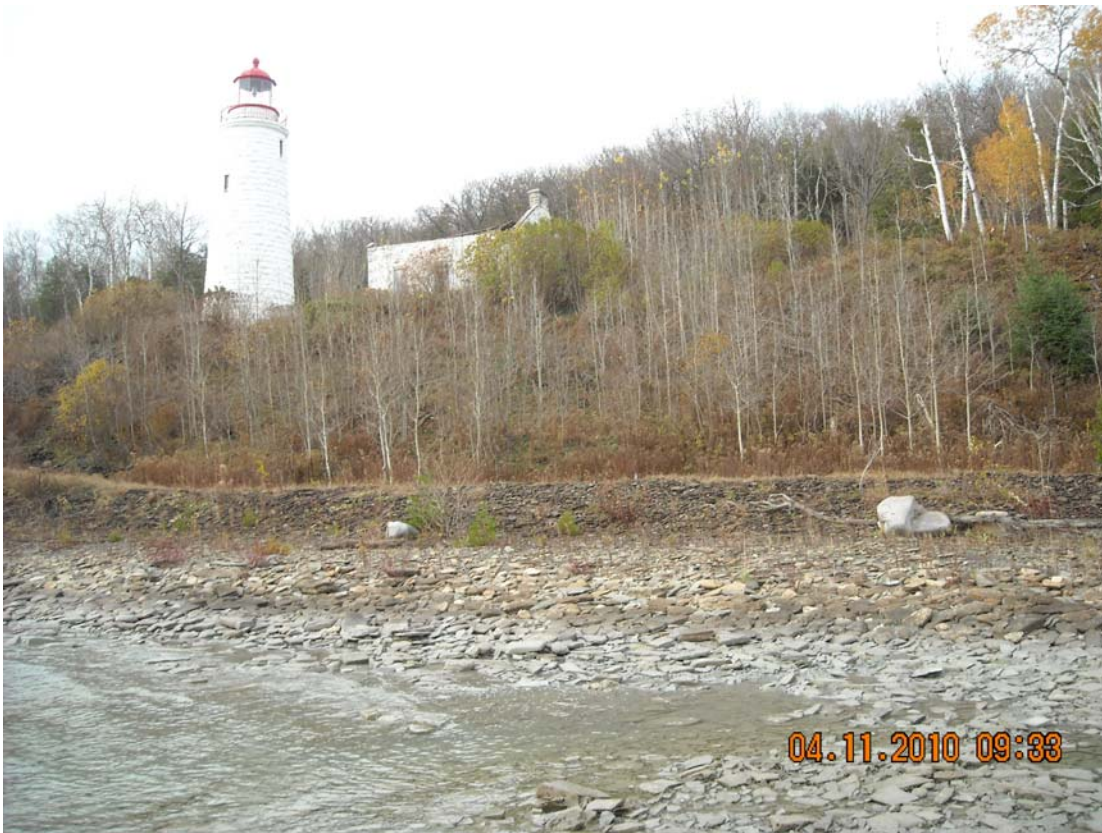
Photograph No. 11 – View of site facing southwest.
