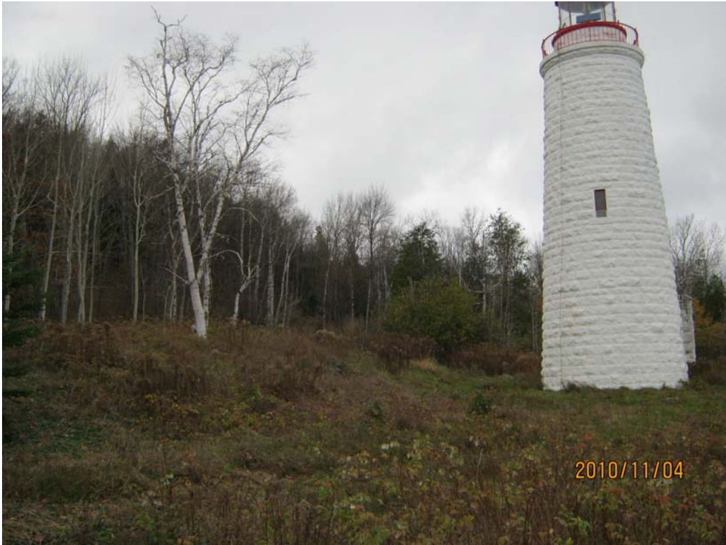
Photograph No.1 – View of light tower facing northwest.
