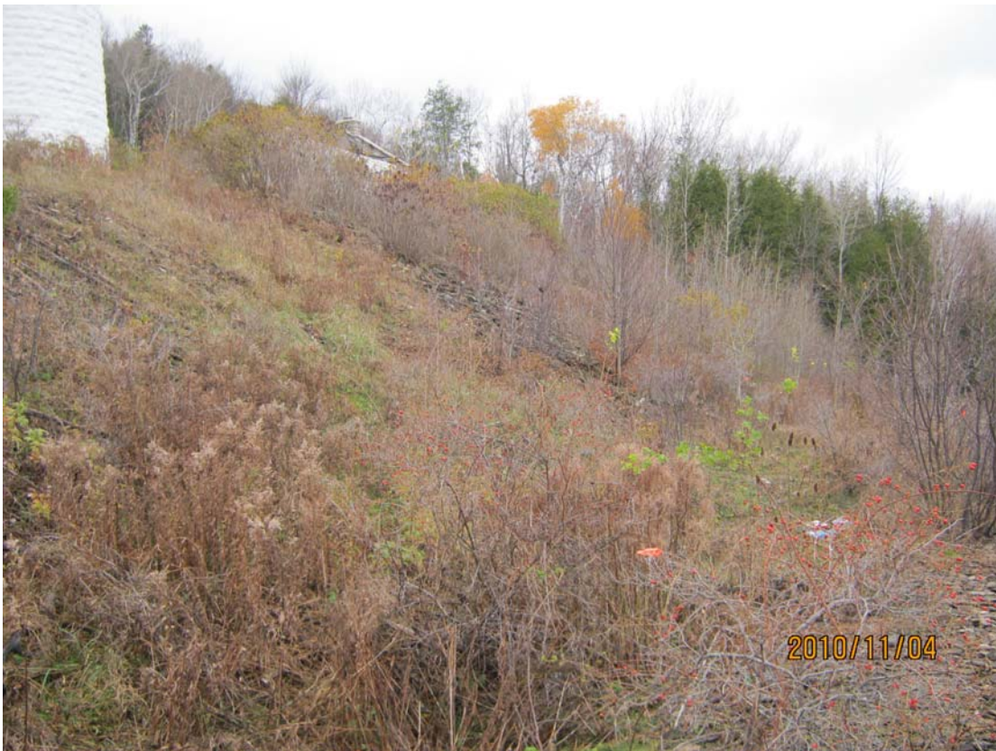
Photograph No.7 – View of slope facing north-northwest
