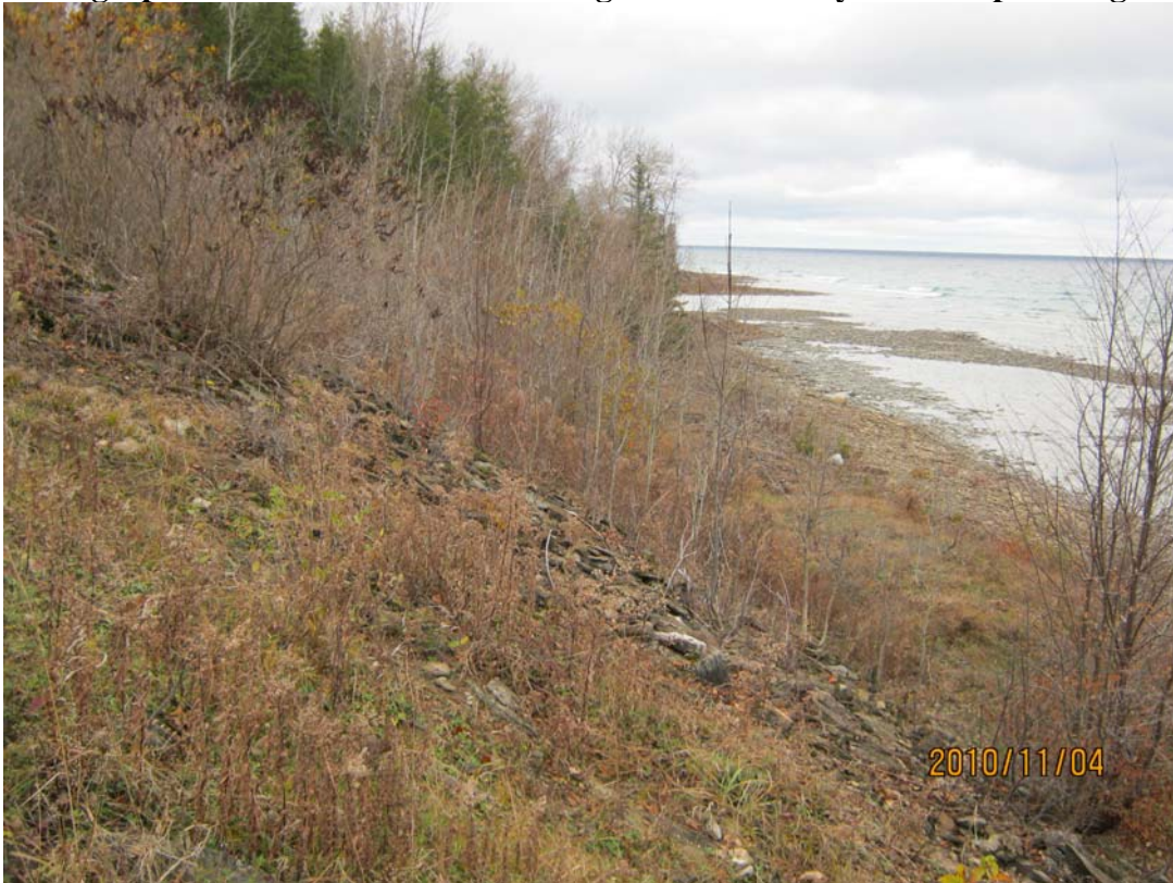
Photograph No.6 – View of slope facing north.
