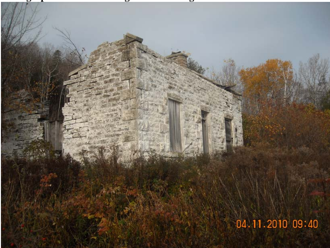
Photograph No.2 – View of former light keepers dwelling facing northwest.
