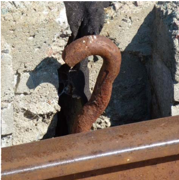
Figure 2 - Damaged deck anchor. Photo shows only one of the two damaged anchors. It is given for information only and may not be entirely representative of the other damaged anchor.
