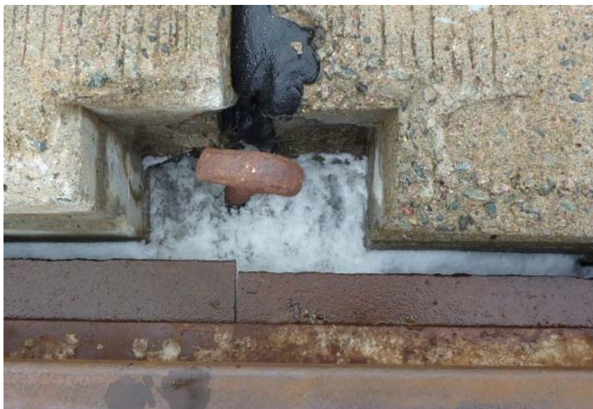
Figure 3 - Damaged deck anchor, top view. Photo shows only one of the two damaged anchors. It is given for information only and may not be entirely representative of the other damaged anchor.
