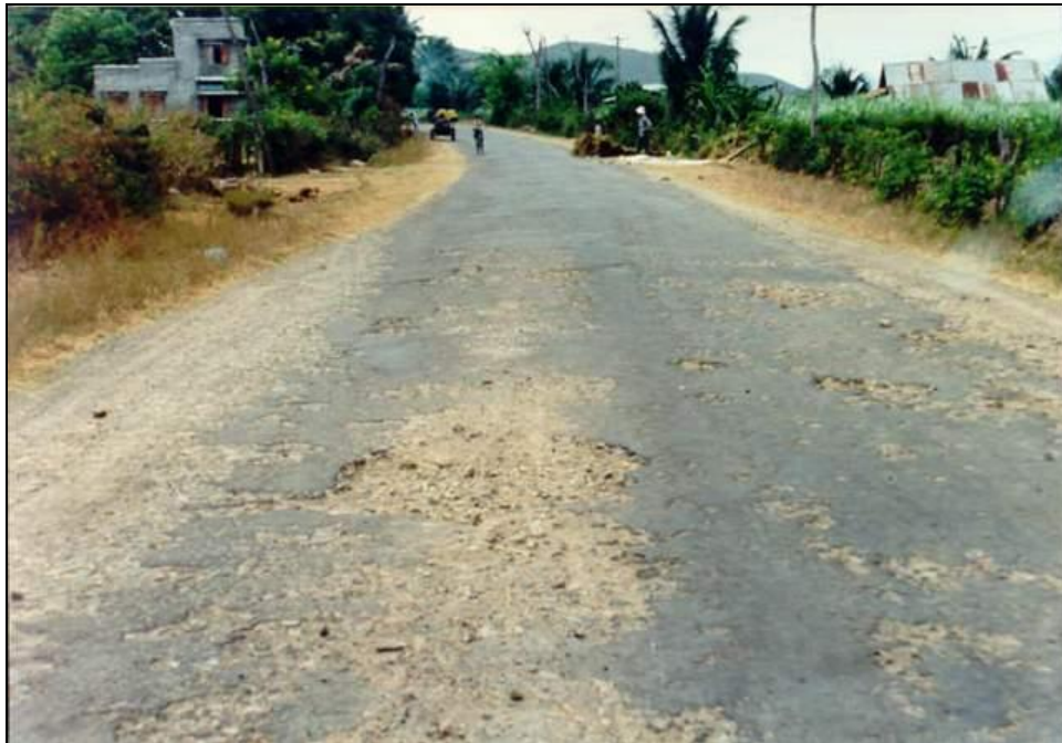
Figure C.2 Secondary Surface: Severely Degraded Pavement
