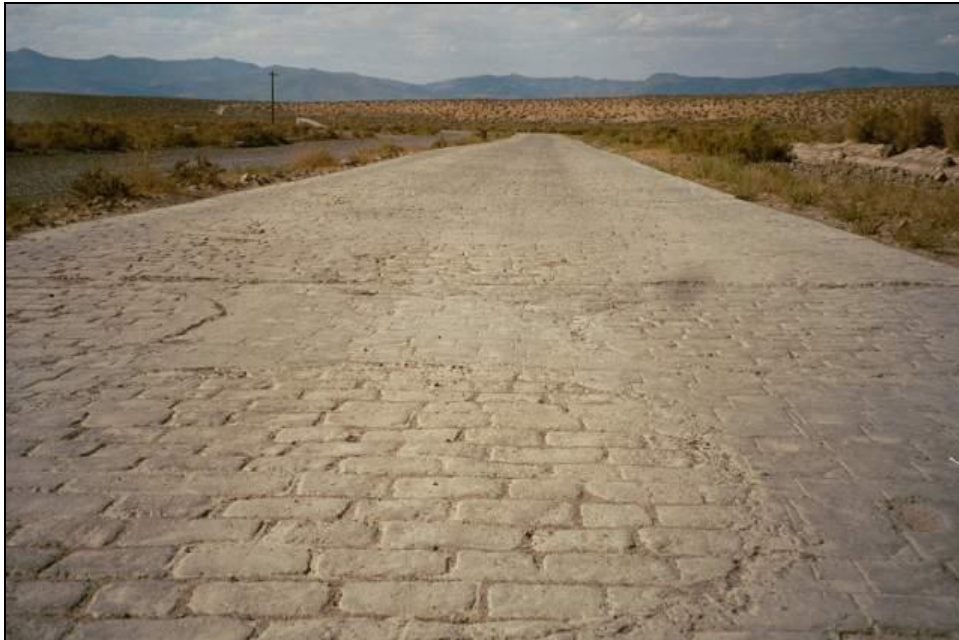
Figure C.4 Secondary Surface: Belgian Block
