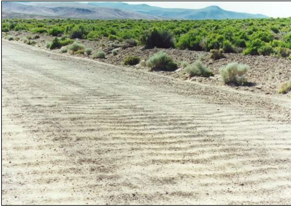
Figure C.3 Secondary Surface: Gravel with Washboard
