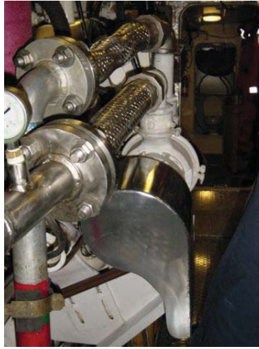
HD-05-Fig. 2 – Fire Pump Piping
