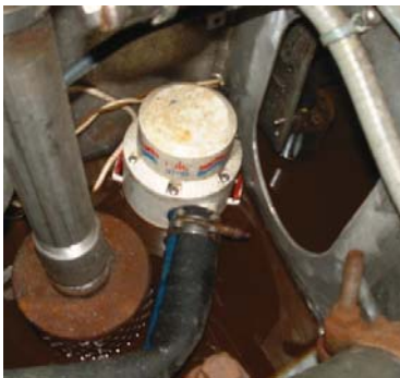
HD-05-Fig. 3&F4 – Engine Room Submersible Pumps (Port Left, Stbd Right)
