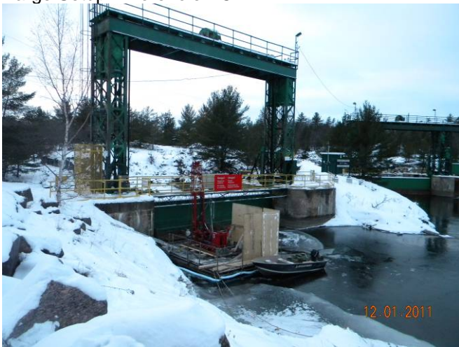
Barge Setup – Borehole BC11-1
