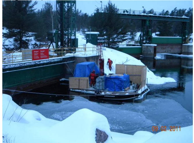
Barge Setup – Borehole BC11-8 -2
