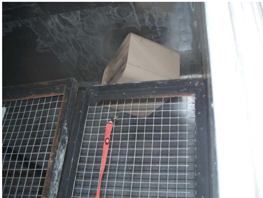
Photograph No. 18 Interior of dog storage building.
