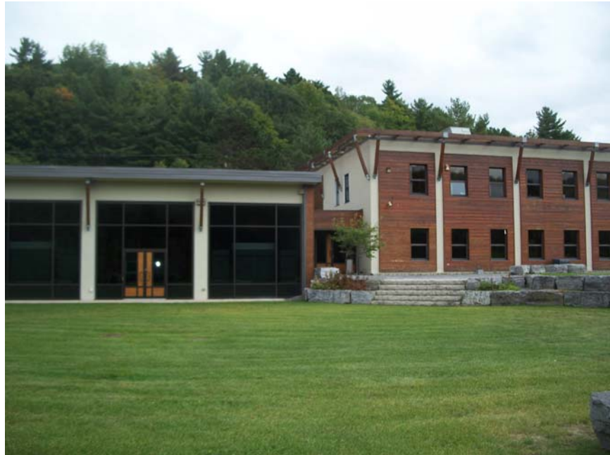
Photograph No. 1 Side view of the Gatineau Visitor Centre
