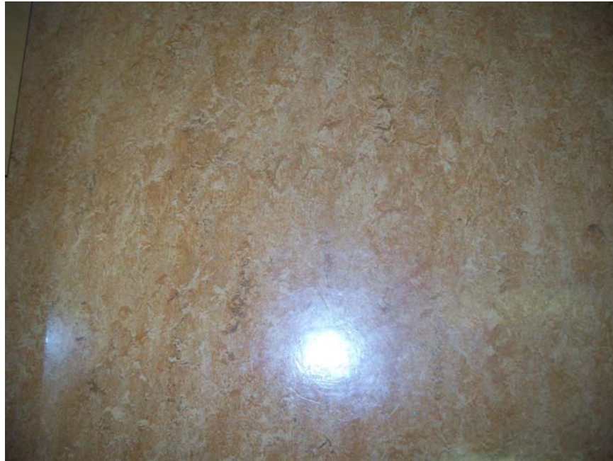
Photograph No. 9 FT3 seamless floor (non-asbestos)
