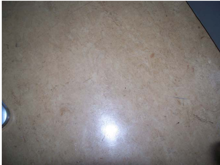
Photograph No. 11 FT2 seamless flooring (non-asbestos)
