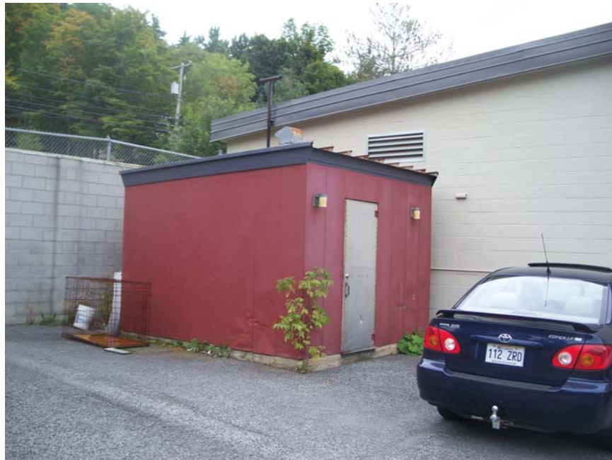
Photograph No. 17 Dog storage building.
