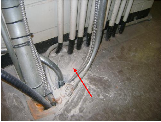
Photograph 1: [Control House Electrical Room - 2 nd Floor] Asbestos-containing grey 9"x9" vinyl floor tile observed to be in fair condition around pipe conduit penetration.
