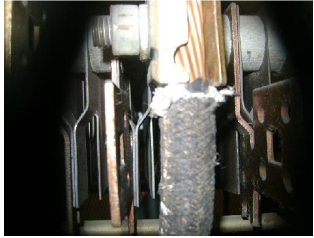
Photograph 2: [Control House Electrical Room (2 nd Floor)] Presumed asbestos-containing electrical cable sheathing observed to be in fair condition.
