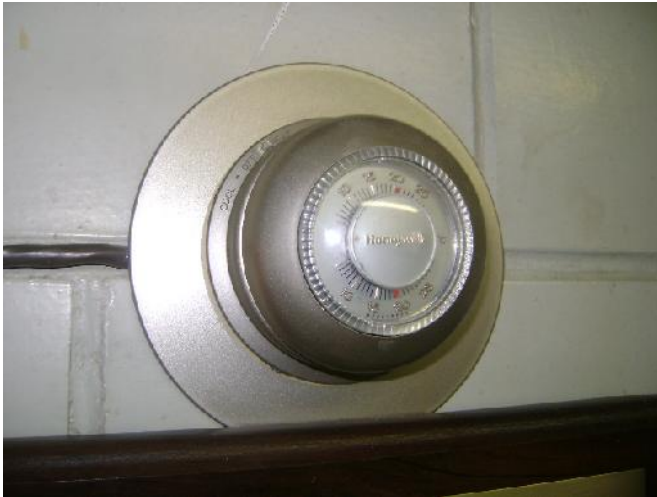
Photograph 11: [Control House – Electrical Room] Mercury-containing thermostat.
