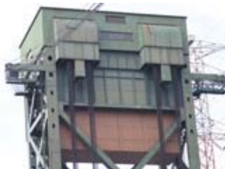
Figure 1: South side of north tower. Nest site is usually on ledge (just above brown counterweight).
