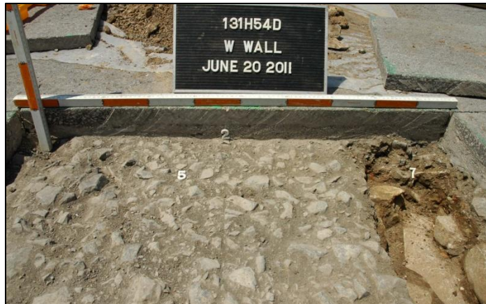
Figure 28: West profile of 131H54D, showing the shallow, macadamized surface laying directly above rubble from the demolition of the officers' barracks (photograph by B. Leskovec; 131H2533E).
