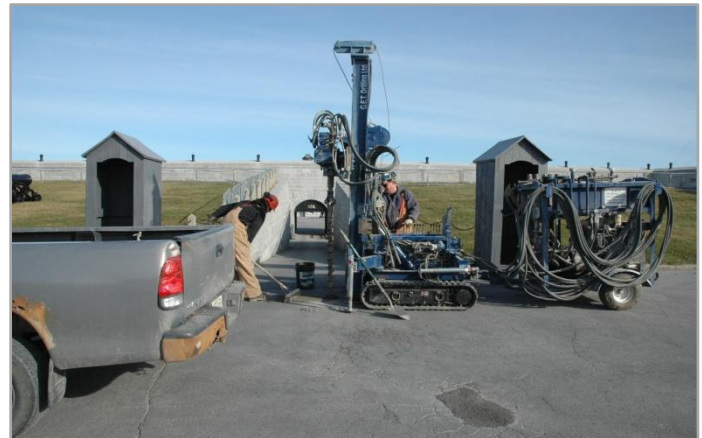
Figure 3: Continuous flight hydraulic auger advancing 131H54L
