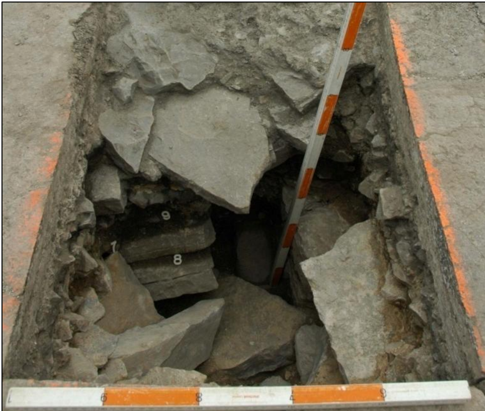
Figure 20: South profile of the officers' barracks in 131H54A. Lot 8 is part of the foundation and the gap to the left of it is the drain feature (photograph by H. Tulloch; 131H2539).
