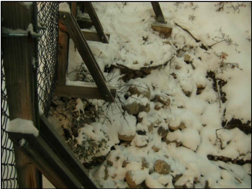
4. Minor Erosion on Downstream Side of Left Abutment.
