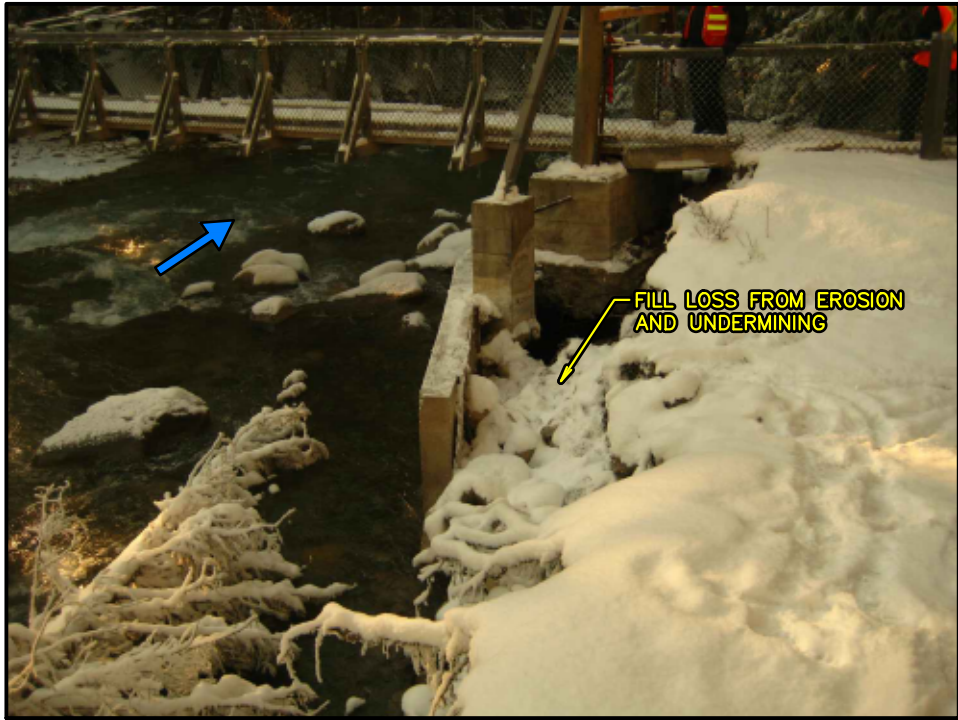
3. View of Existing Right Abutment. Note Fill Loss Behind Abutment Wall.
