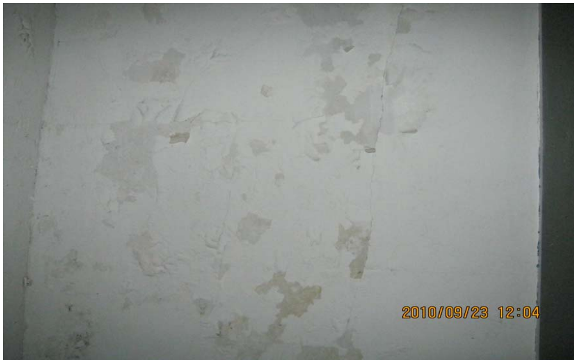
Photo 4: View L.H LS-6 sample location from lighthouse third floor interior wall. Sample was found to be above criteria and is considered lead based.
