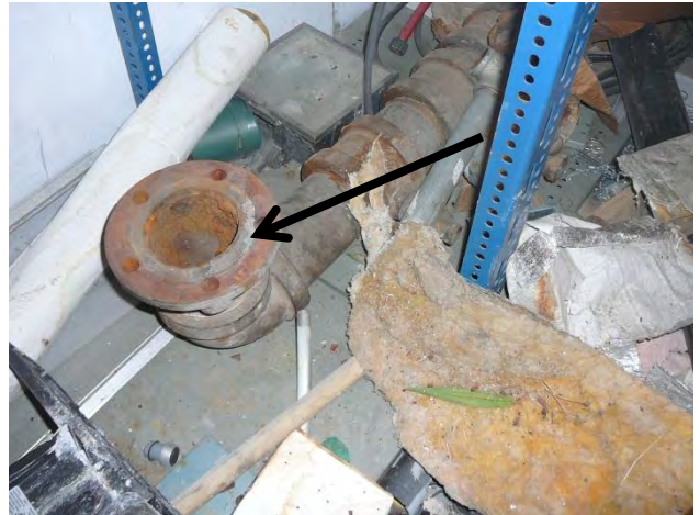
Sample A105 : Gasket containing asbestos in Basement Pool Mechanical room
