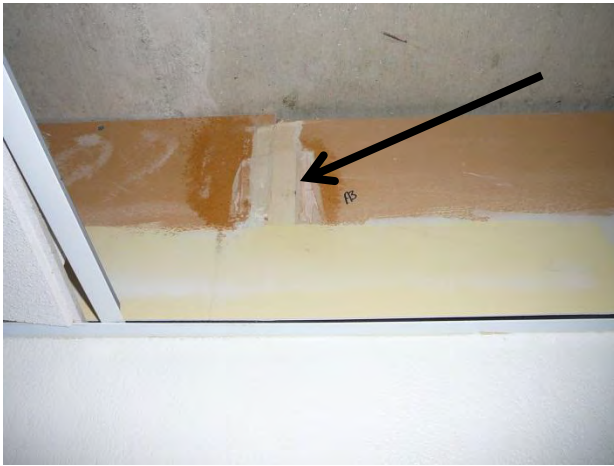
Sample A3 : Drywall putty containing asbestos in ceiling space of Main floor Hall 1
