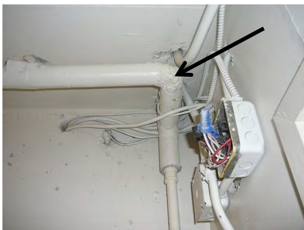
Sample A73 : Pipe elbow insulation containing asbestos in Lower floor Linen room
