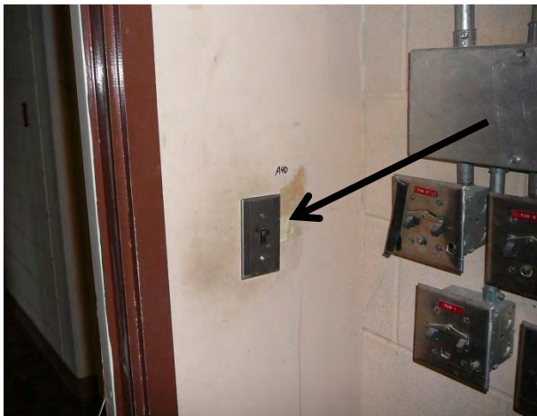
Sample A40 : Drywall putty containing asbestos in 2 nd floor Satellite Receiving room
