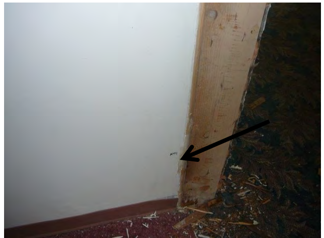
Sample A44 : Drywall putty containing asbestos in Main floor Room 249
