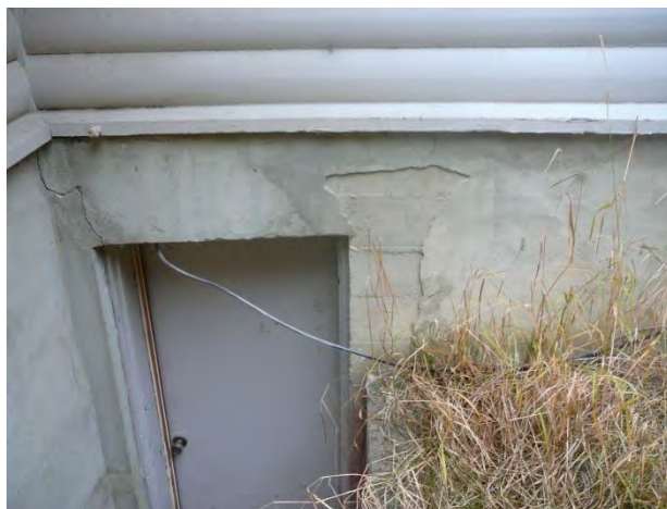
Sample A4 : Gray skim coat containing asbestos on exterior basement walls
