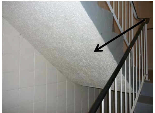
Sample A11 : Ceiling stipple containing asbestos in Main floor Stair 1
