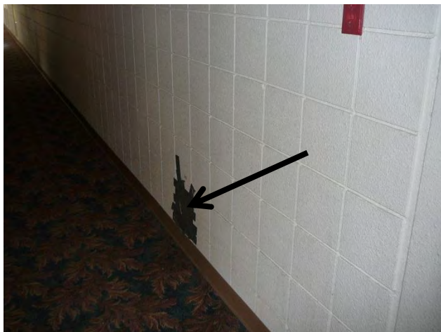
Sample A85 : Vermiculite containing asbestos in 2 nd floor Hall 3 wall
