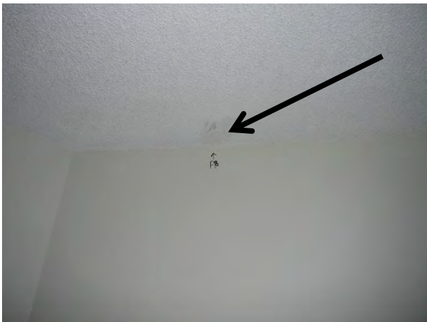
Sample A8 : Ceiling stipple containing asbestos in 2 nd floor Room 378
