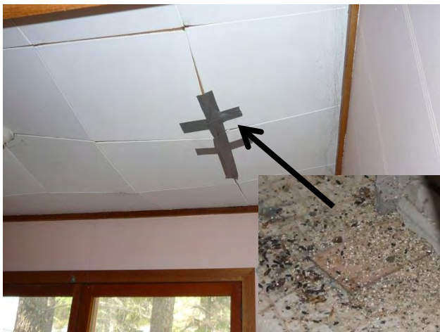
Sample A18 : Vermiculite containing asbestos in laundry room ceiling space
