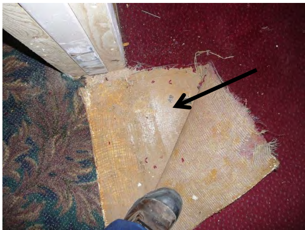
Sample A58a : Vinyl floor tile containing asbestos in Main floor Dining room
