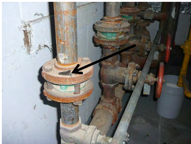
Sample A101 : Gasket containing asbestos in Lower floor Mechanical room
