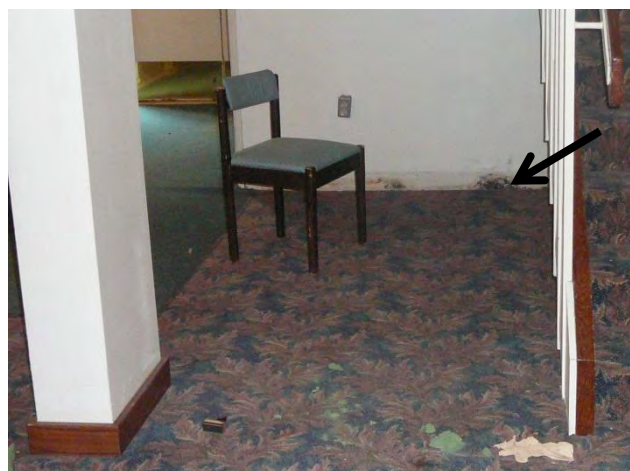
Mould under Lower floor Main Stairs
