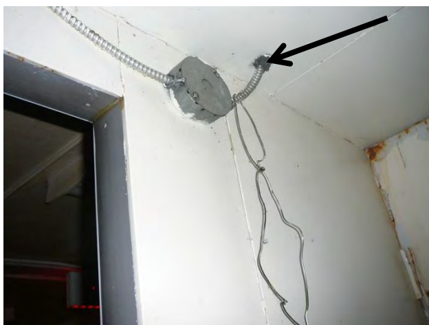
Sample A69 : Black caulking containing asbestos in Main floor Cooler 1
