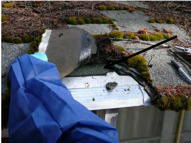
Sample A1 : Green shingles with tar containing asbestos on roof
