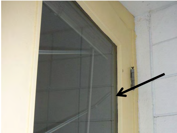
Sample A28 : Window caulking containing asbestos on 2 nd floor Room 382 exterior balcony door
