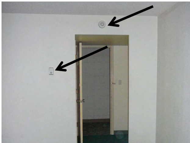
Thermostat containing mercury and smoke detector containing radioactive material in guest room
