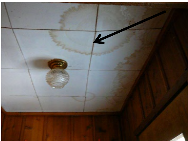
Water damage in Entry 2
