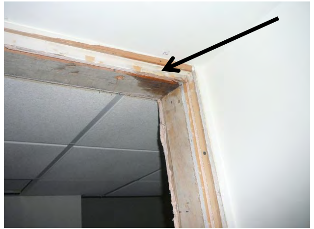
Sample A5 : Drywall putty containing asbestos in 2 nd floor Room 253
