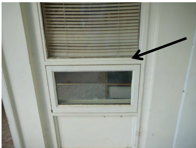
Sample A104 : Window caulking containing asbestos on Lower floor Games room
