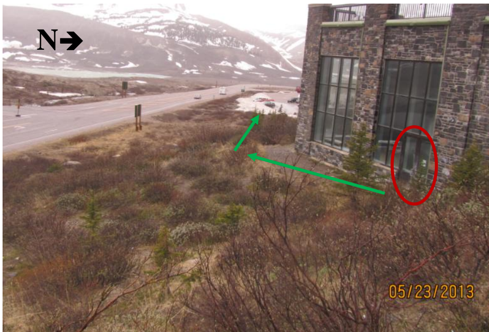
Photo 1. Photo facing West showing the South-East door (circled in red) coming from the Theatre. This door will be made into an Emergency Exit. The green arrows roughly indicate the placement of the proposed emergency egress.
