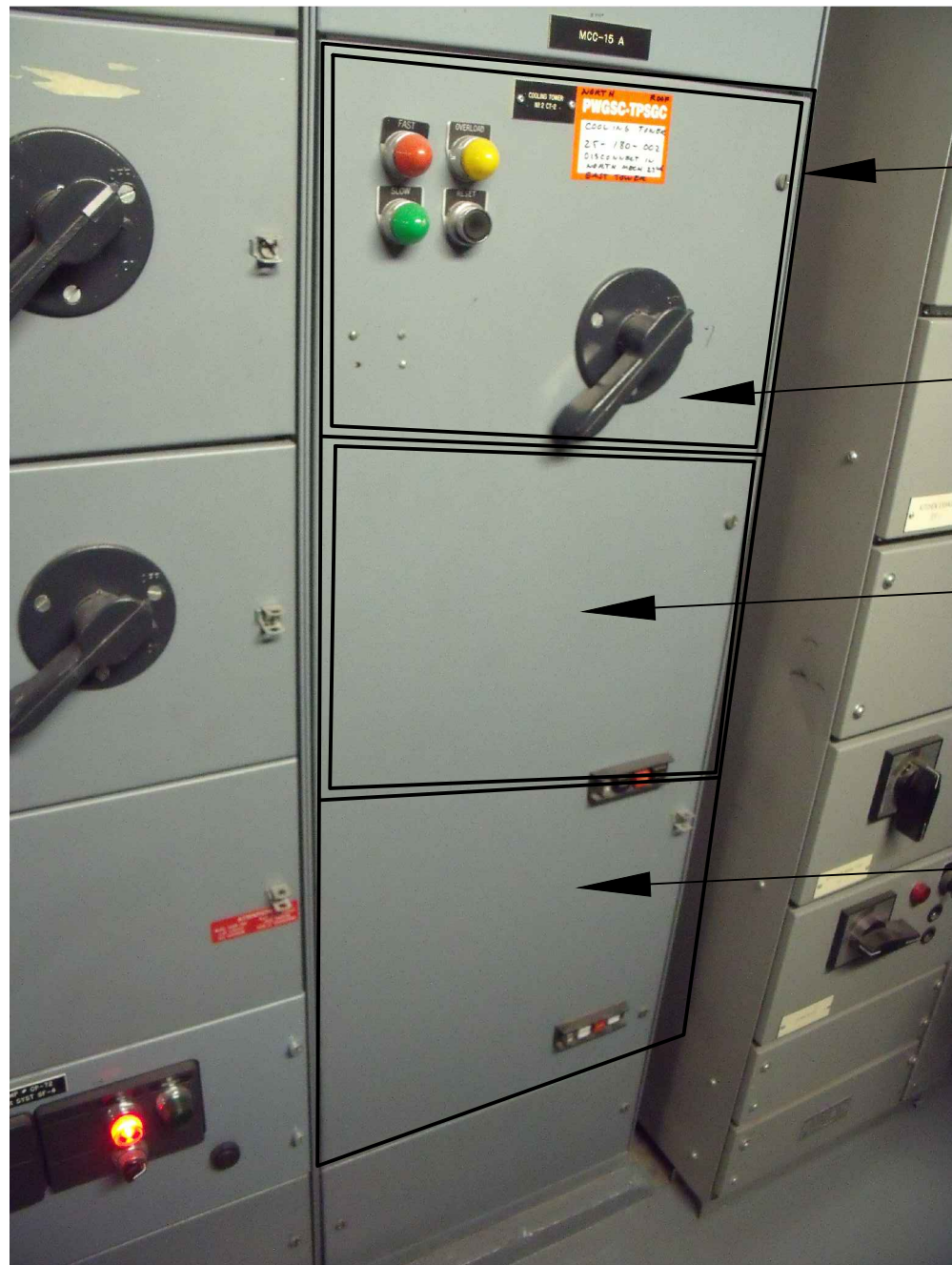
3 E1 EXISTING COOLING TOWER MOTOR STARTER (40+10 hp) SCALE N.T.S.
