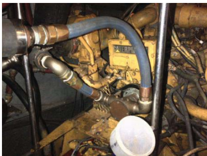
HD-05-Fig. 2 – Fire Pump Piping
