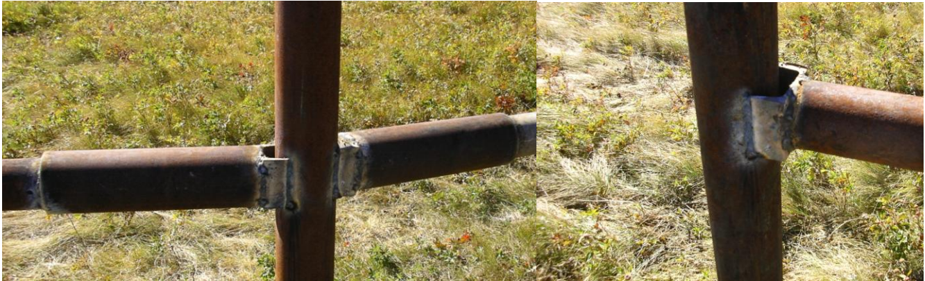
Examples of approved channel iron brackets and pipe sleeves for attaching horizontal crossbars.
