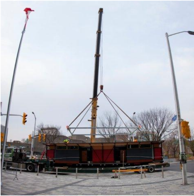
Past lifting operations
