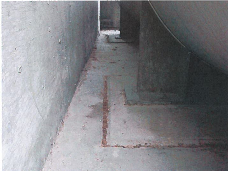
PHOTO 5: PUMPHOUSE DIESEL FUEL STORAGE TANK Tank support saddles
