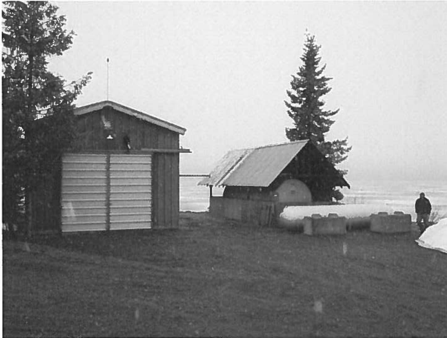
PHOTO 1: PUMPHOUSE BUILDING AND DIESEL FUEL STORAGE TANK
