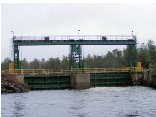
15 H16 NORTH DAM DOWNSTREAM FACE
