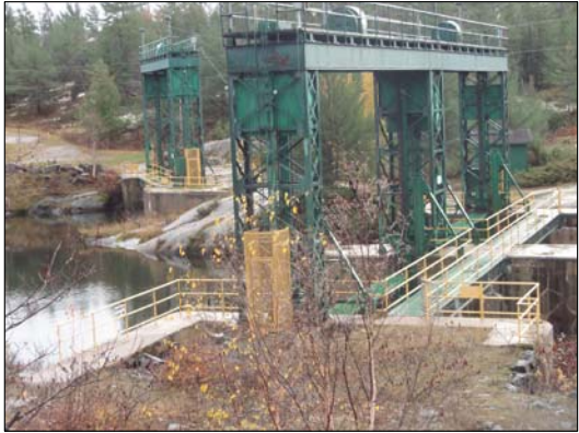
1 H16 MACHINERY BRIDGE DECK AND ACCESS WALKWAY
