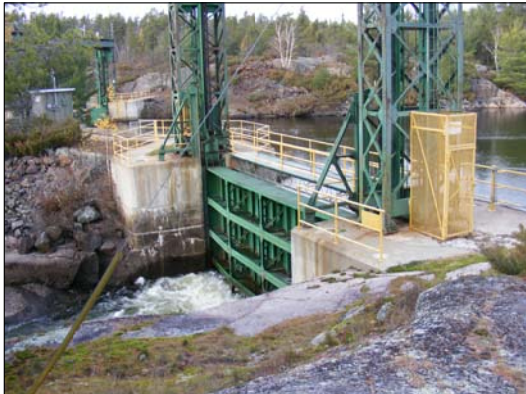
33 H16 SOUTH DAM: ROLLER GATE, DOWNSTREAM VIEW
