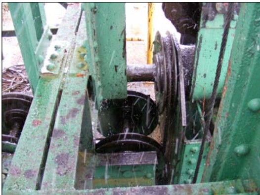
39 H16 PULLEYS AND CABLES (GATELIFTING MACHINERY)
