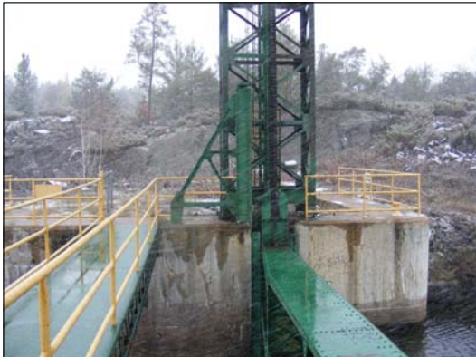
35 H16 NORTH DAM NORTH ABUTMENT SHOWING GATE GAIN AND TOWER
