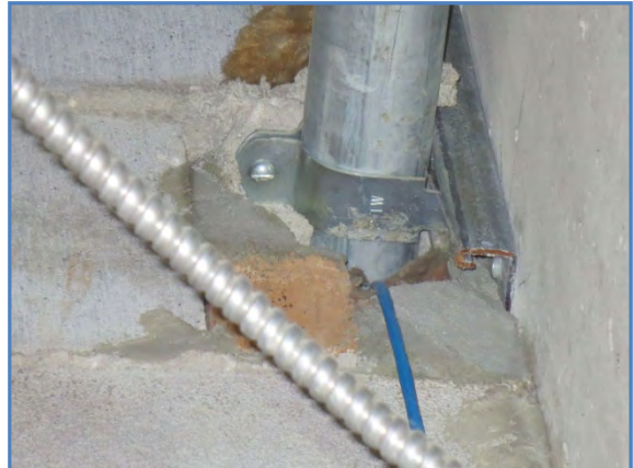
2029-02 Conduit through masonry wall above door.
