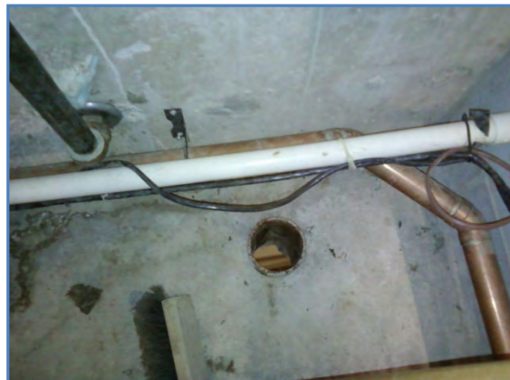
1003-04 Unprotected sleeved opening in floor
