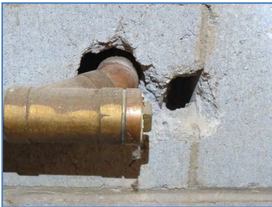
1003-03 2 openings through masonry wall at south; one with copper pipe
