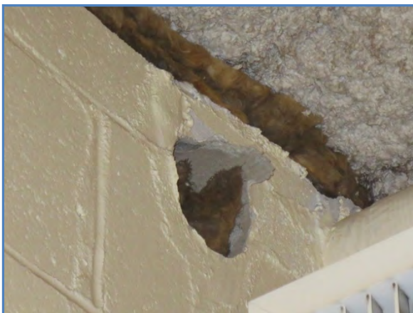
0010-02 Unprotected opening - above door
