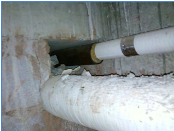
1003-05 Opening in masonry wall above door
