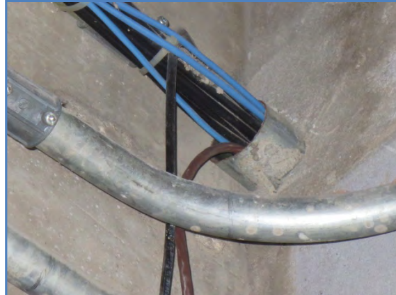
1024-01 Unprotected sleeve with conduit and cables above door
