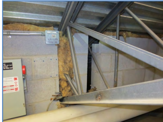
2051-02 Penetrations of roof trusses through masonry wall where packing has fallen away.
