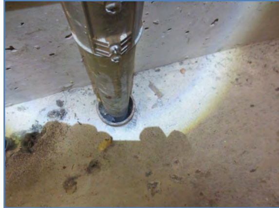
1026-04 Conduit through sleeved opening at floor near south wall
