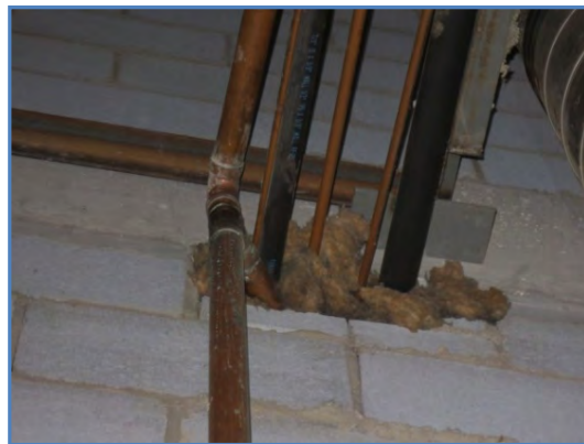
2004-01 Batt insulation to be removed from opening in south masonry wall and replaced with fire stopping
