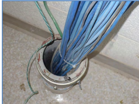
140-01 Data lines through unprotected sleeve
