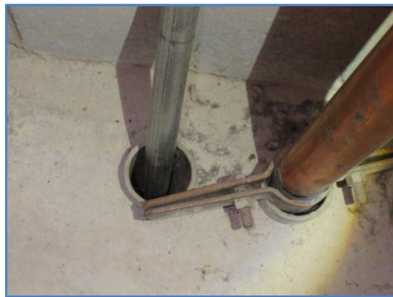
1026-02 Conduit through sleeved opening at floor near north wall
