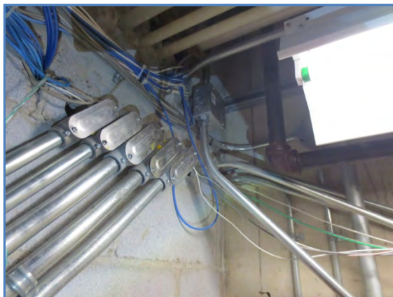
1026-01 Multiple openings through masonry wall above door
