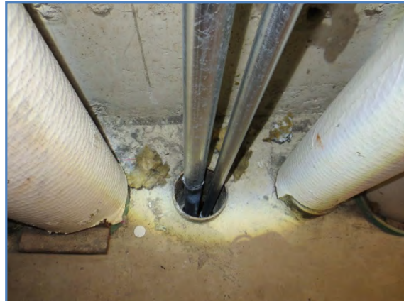
1025-02 Unprotected sleeved opening at floor - south wall
