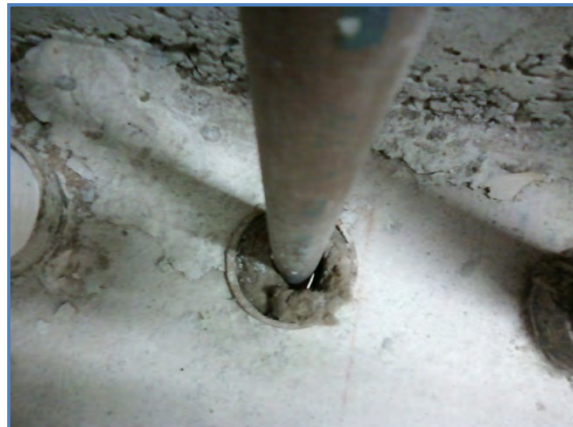
1005-02 Remove existing packing and fire stop
