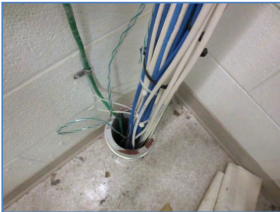
141-02 Data lines through unprotected sleeve
