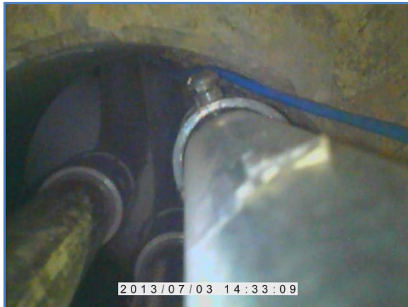
1025-05 Multiple (3) sleeved openings with conduit and cabling through south wall above corridor ceiling
