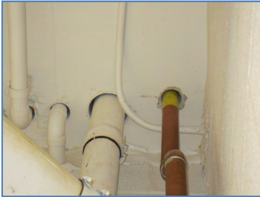
129-01 Sleeved and unsleeved openings through concrete floor slab
