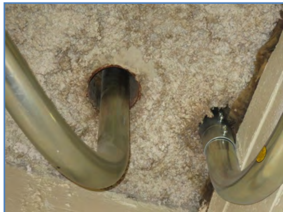
0010-01 Conduits through sleeved openings in floor slab - above door
