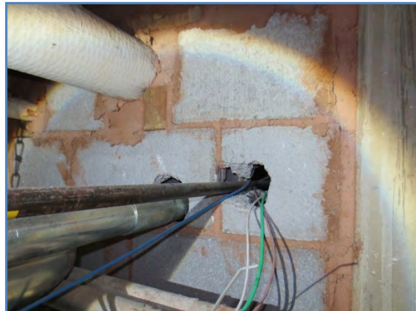
1025-06 Conduit and cabling through multiple holes in masonry wall above door
