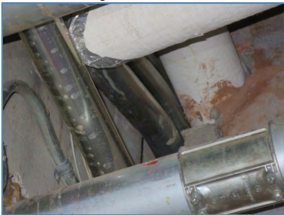
2031-01 Conduit through opening in masonry wall above door
