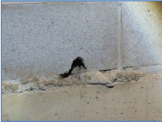
1025-01 Opening in masonry at north wall
