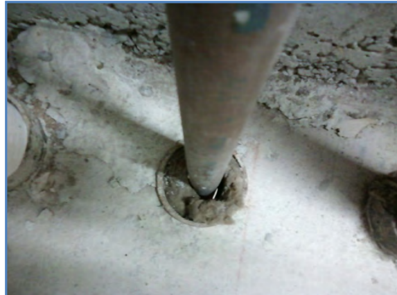
1005-02 Remove existing packing and fire stop
