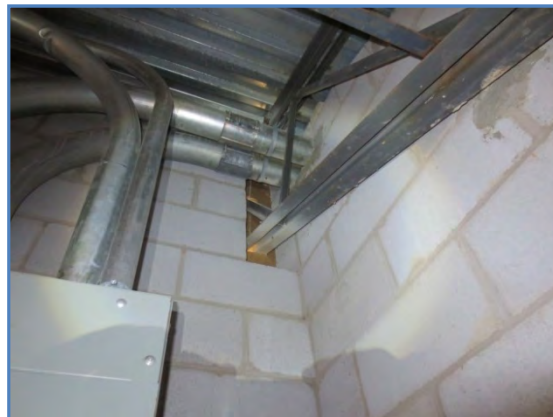
2053-01 Penetrations of roof truss through masonry wall at north
