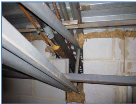
2201-01 Penetrations of roof truss through masonry wall at south.
