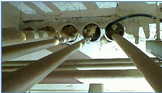
1111-01 Partially protected sleeved openings through masonry wall above door 1119-B openings. Replace existing packing with new fire stopping.
