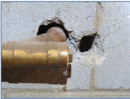
1003-03 2 openings through masonry wall at south; one with copper pipe
