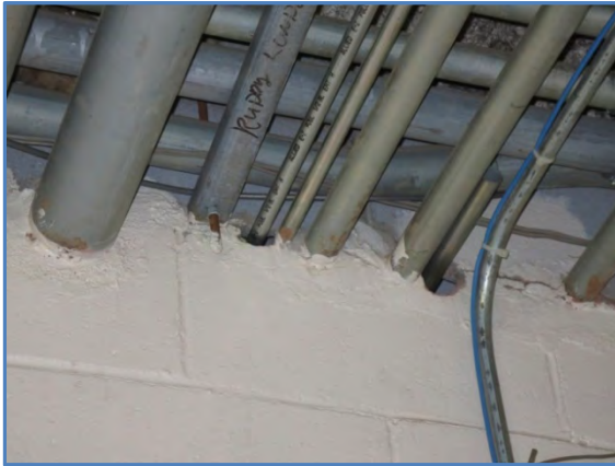
0007-01 Conduit through masonry block wall above door
