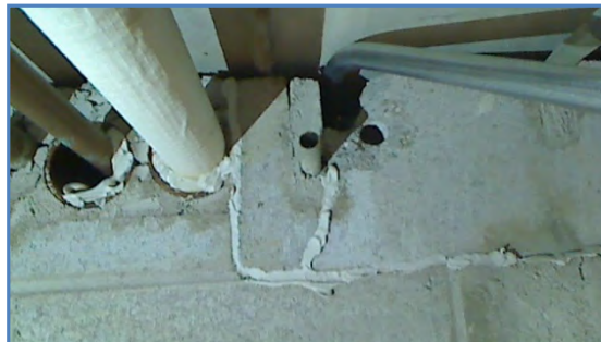
1112-01 Openings through masonry wall above door 1119-B.
