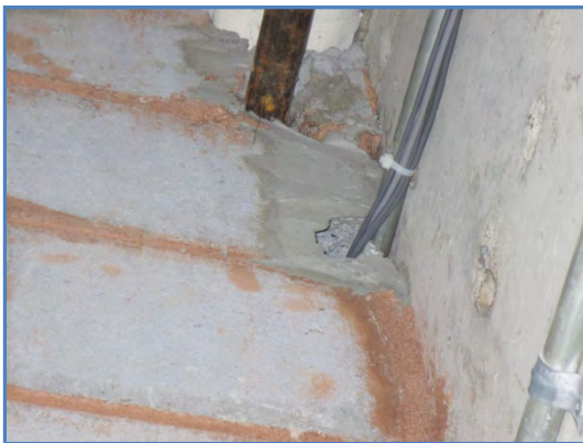
2003-01 Conduit/cabling through opening in masonry wall above door
