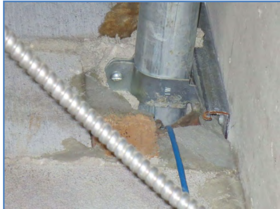
2029-02 Conduit through masonry wall above door.
