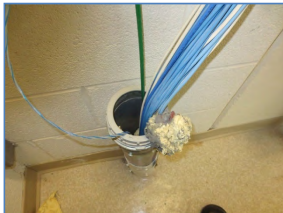
240-01 Data lines through unprotected sleeve
