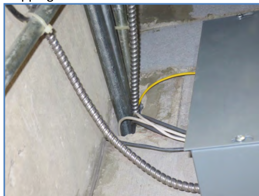
2005-02 Conduit and cabling through opening in masonry wall above door
