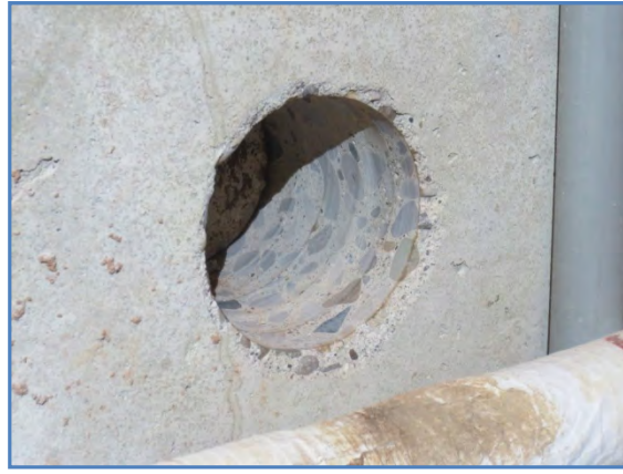
1003-02 Unprotected unsleeved opening through concrete wall at north
