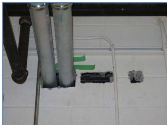
015-02 Conduit through openings in masonry - west wall
