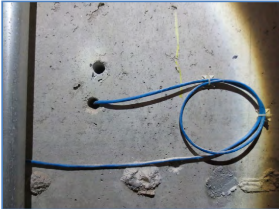
2029-01 Multiple 35mm openings through concrete wall; some with cabling
