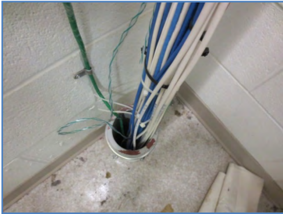
141-02 Data lines through unprotected sleeve
