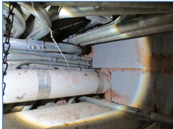
1025-08 Openings through masonry wall above door
