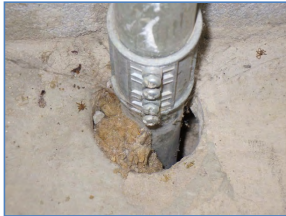
2050-02 Conduit through unsleeved opening. Remove existing packing and replace with fire stopping
