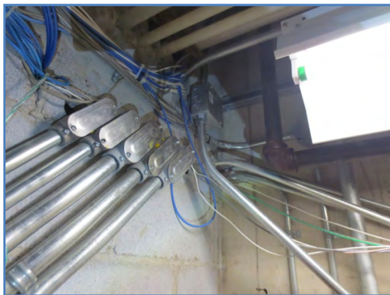
1026-01 Multiple openings through masonry wall above door
