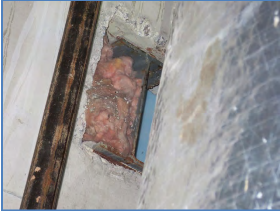
1006-01 Unprotected beam pocket on south wall
