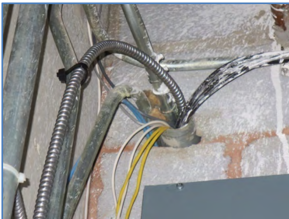
1005-03 Multiple conduits through masonry block above door
