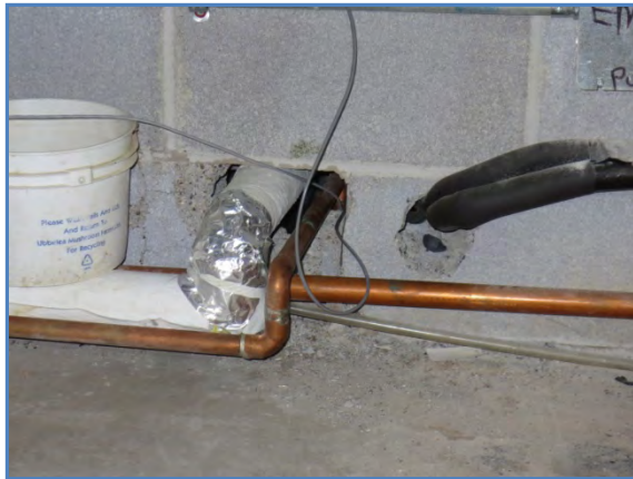
2050-01 Copper piping through openings in masonry wall at south
