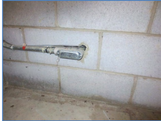
2054-01 Conduit through masonry wall at west
