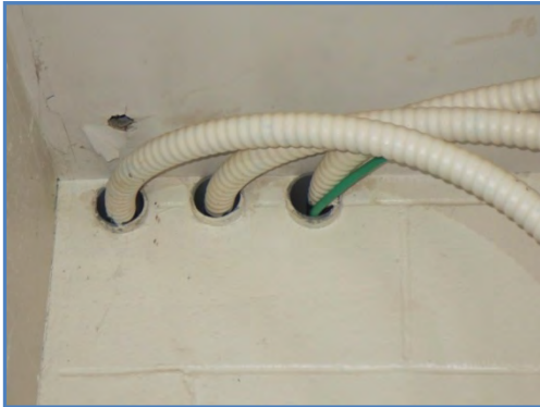
1305-01 Conduit through sleeved openings in masonry wall
