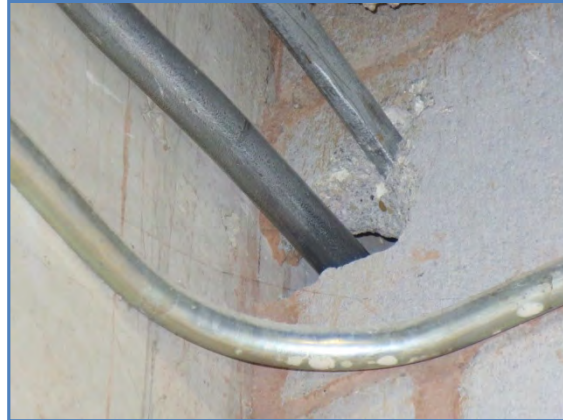
1004-02 Conduit through masonry wall above door
