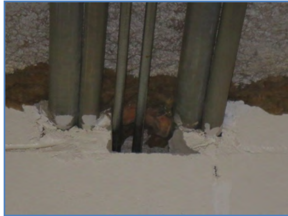
0007-02 Conduit through masonry wall at ceiling - several instances
