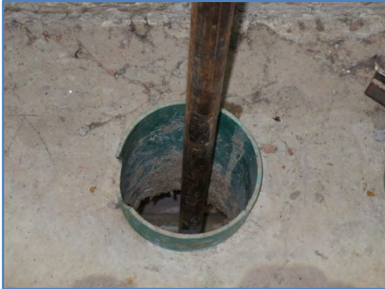
1004-01 Plastic sleeve with 25mm metal pipe at floor near north wall
