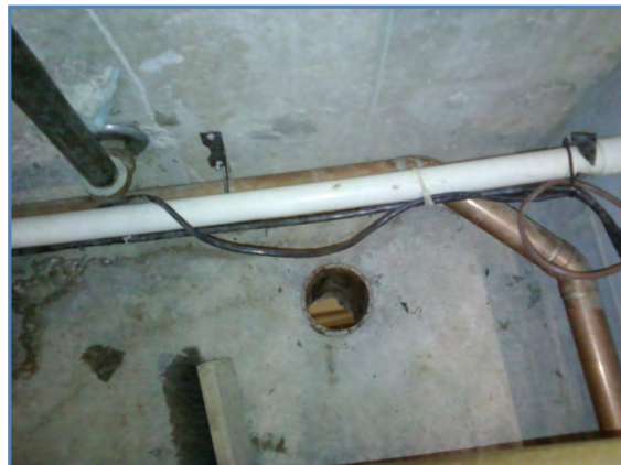
1003-04 Unprotected sleeved opening in floor
