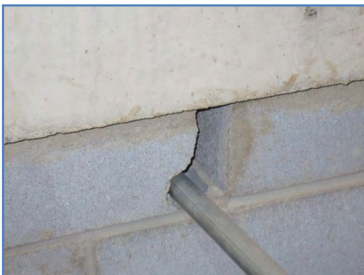
2005-01 Conduit through opening in north masonry wall just below 2 nd floor slab
