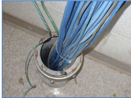
140-01 Data lines through unprotected sleeve
