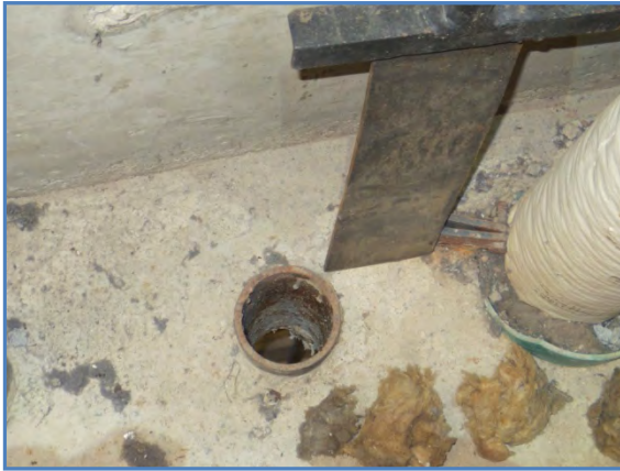
1003-01 Unprotected sleeved opening at floor - north
