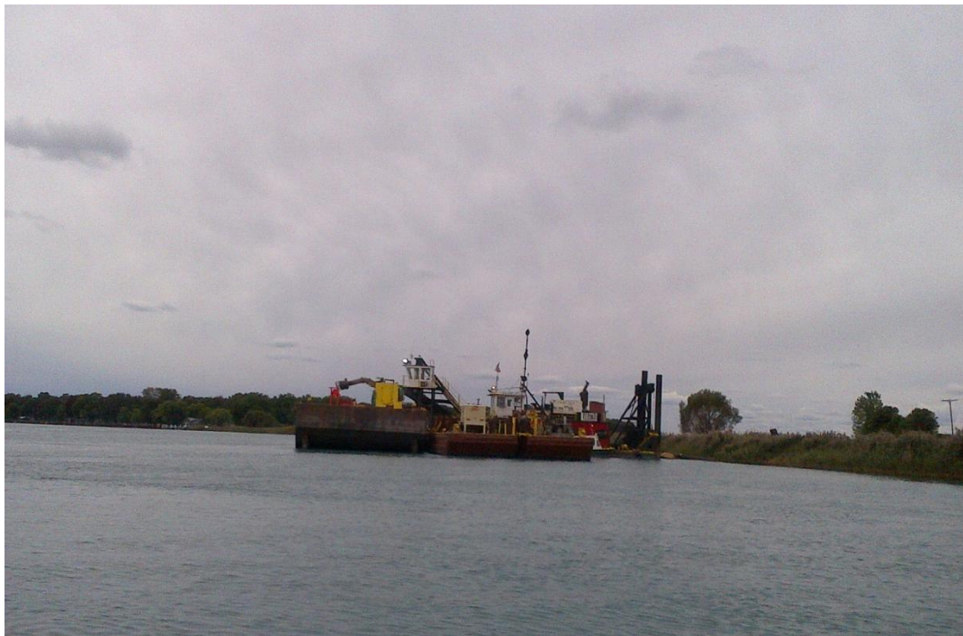
Photo 2: September 2012, View of offloading at pipeline access point.
