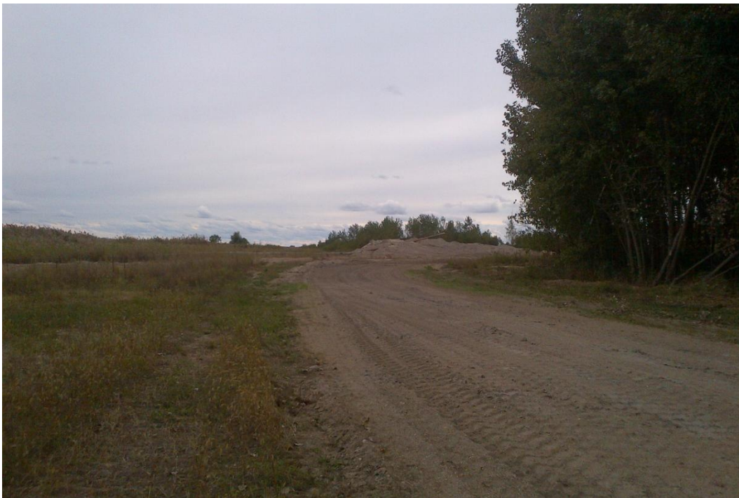
Photo 6: September 2012, View looking west along temporary haul road within CDF.
