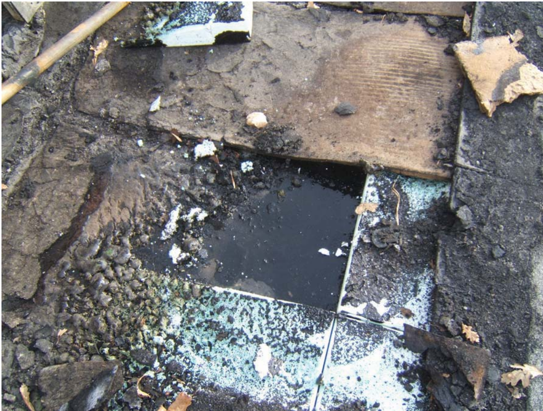
Photo 5 I removed a piece of the MEPS and we see the moisture laying on the VB and it is under the edge of this area.
