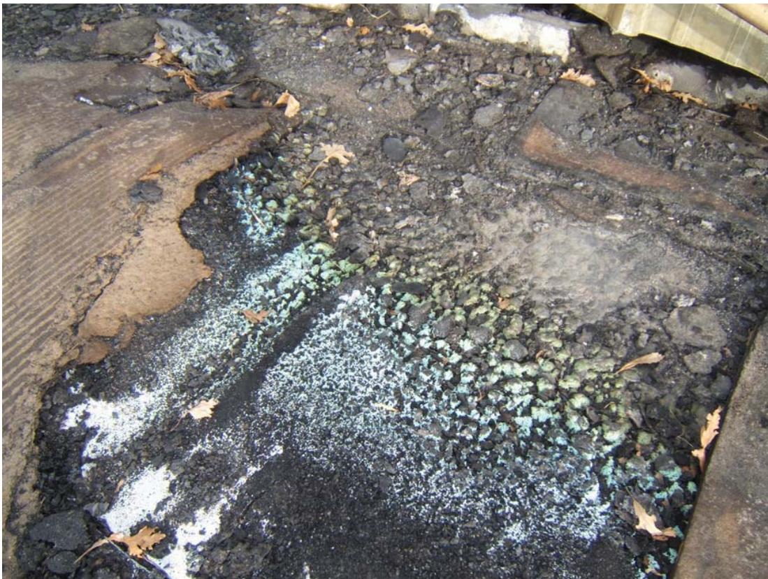
Photo 4 A closer look of the roof we see the melted insulation and some of the fiberboard.
