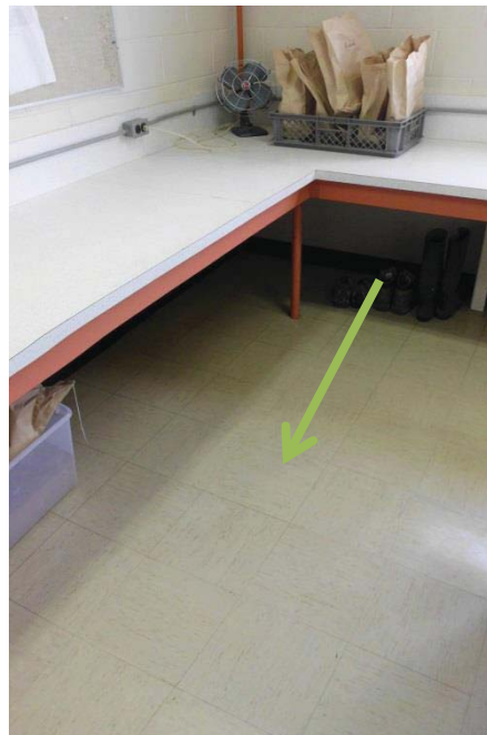
Asbestos containing materials in brown streak floor tiles in room 105
