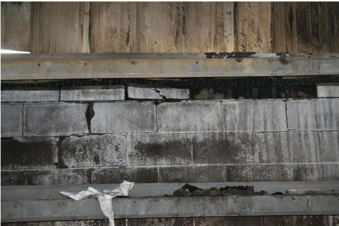
Fire damage to concrete block wall
