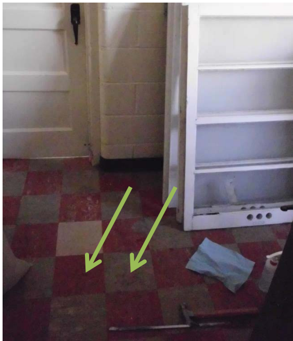
Asbestos containing materials in marble brown, and red, floor tiles in room 107
