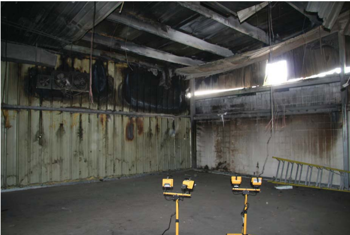
Fire damage at south wall
