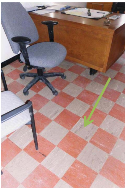
Asbestos containing materials in marble brown floor tiles in room 102
