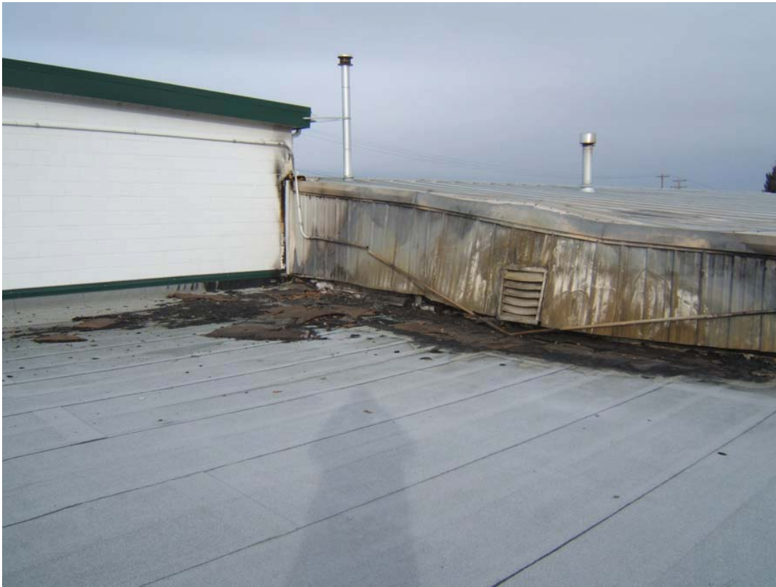
Photo 1 We see the damage to the roof along the North edge.
