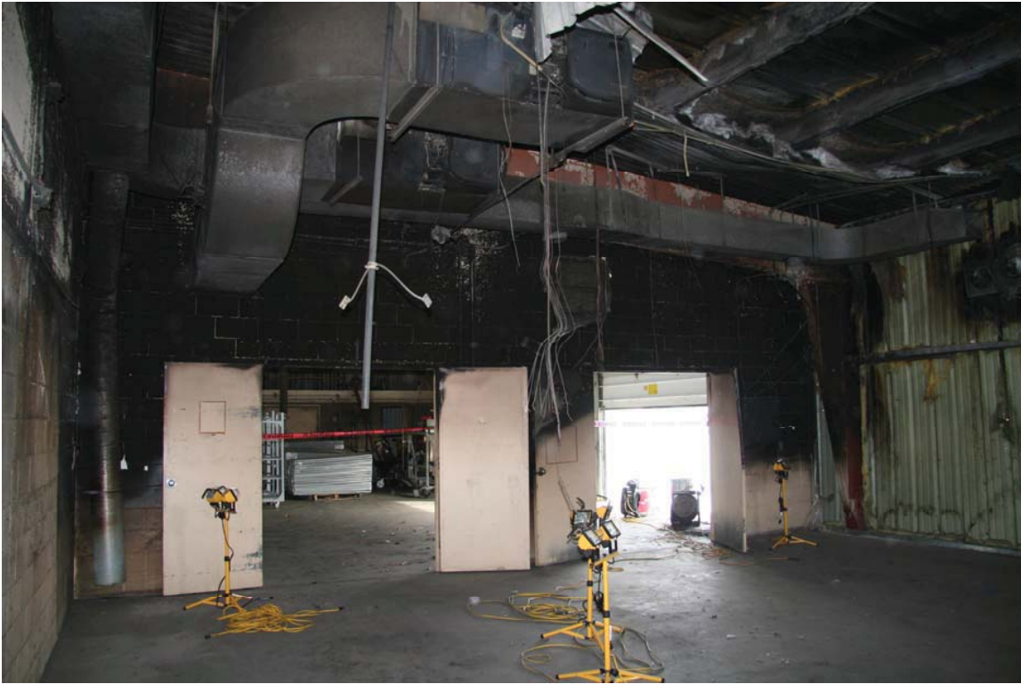
Fire damage in drying room
